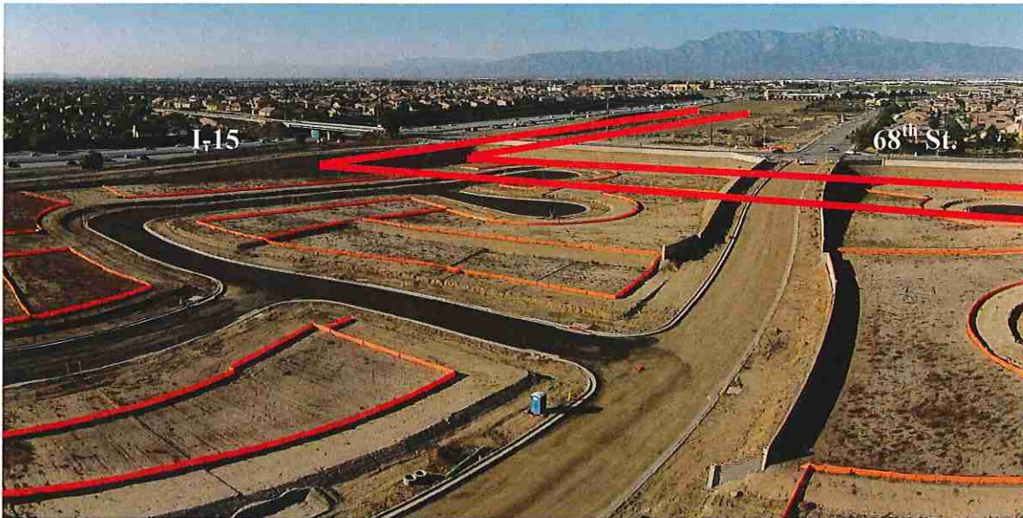
Photo 1: Looking north on Pats Ranch Rd. Cross street is 68 th Street. The picture show walls under construction and streets ready for asphalt. The RTRP would cause the removal of the northwest cul-de-sac and its homes. [The RTRP proposed easement is shown in red (approximate)]
