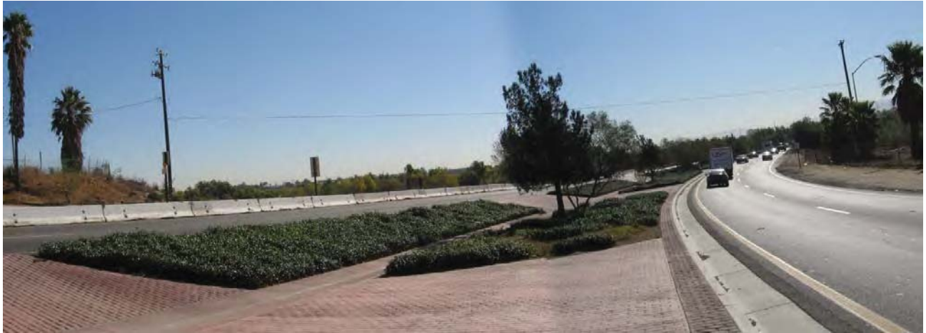
FIGURE 12. VIEW LOOKING SOUTH ON VAN BUREN BOULEVARD NORTH OF RIVER
