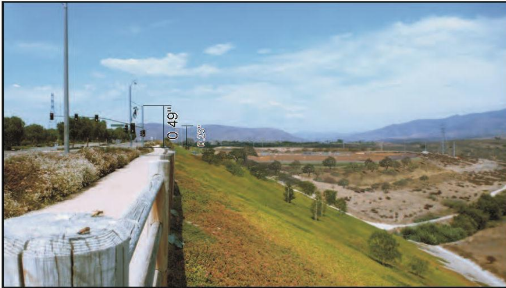
Exhibit 2 - SDG&E supplied visual simulation from Key View 7 using a 26mm equivalent focal length lens. The horizontal field of view for this photo is \pm 80^\circ . Note the vertical dimension of the street light pole and the existing monopole of TL 6913.
