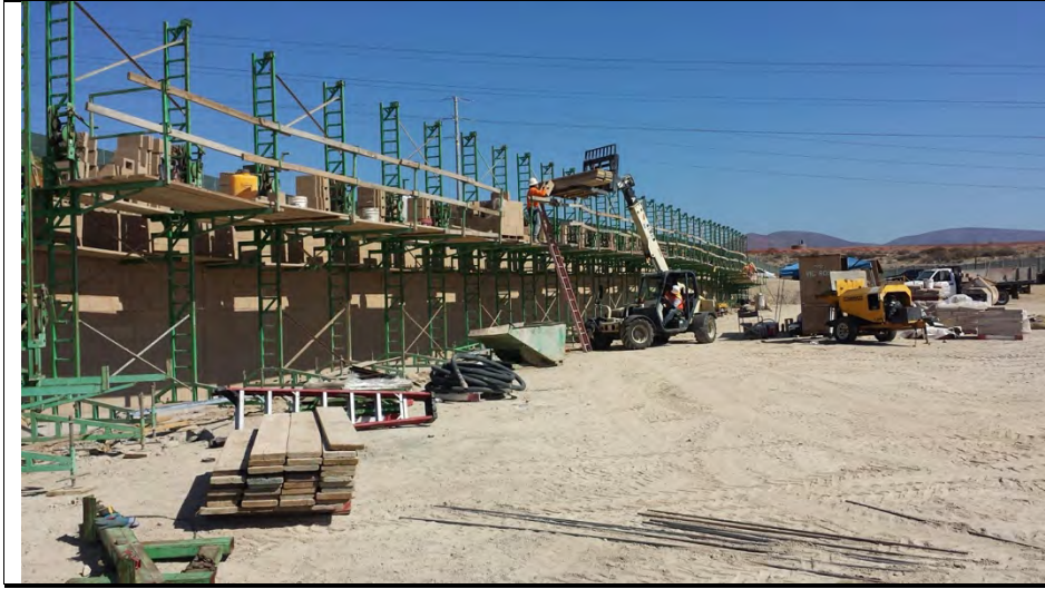
Photograph 3: Construction of the masonry wall during the week of October 15, 2016.
