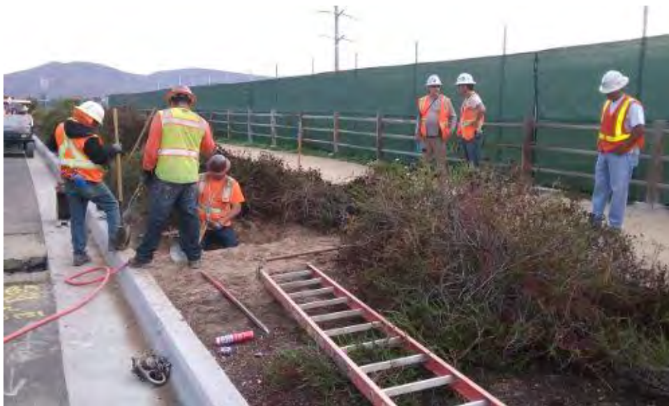
Caption Trenching for nonpotable water line with paleo monitor present.
