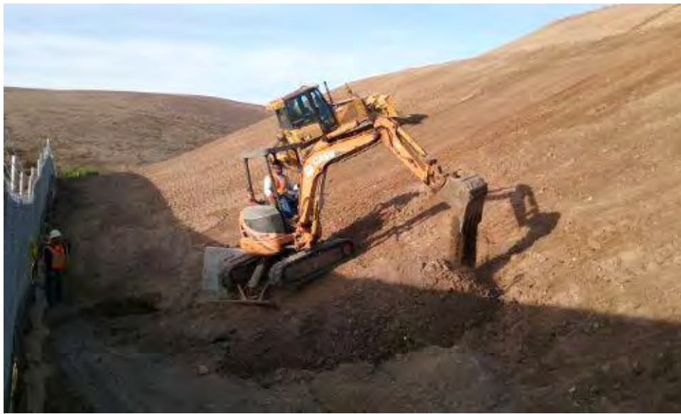
Caption Trenching and track-walking in northeast corner.
