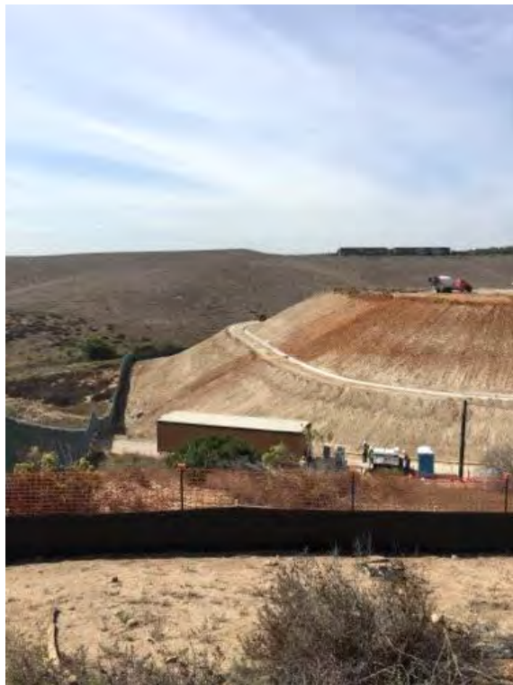
Caption Southern site including slopes. New concrete in v-ditch.
