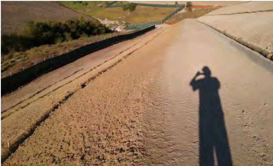
Caption Hydromulch has been applied on lower slopes on west end.
