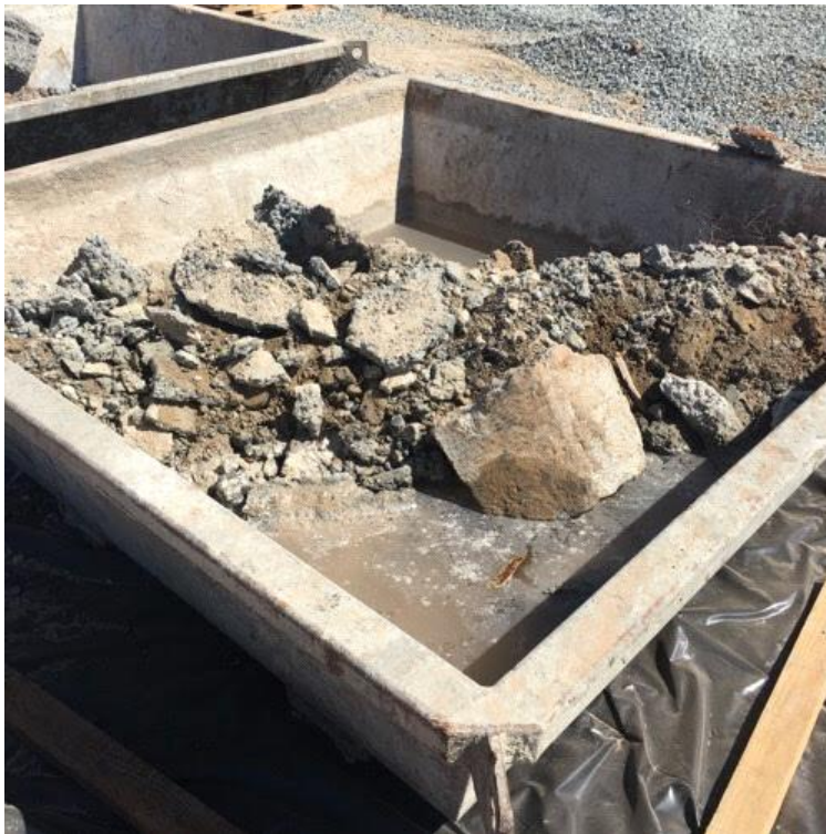
Caption Concrete washout
