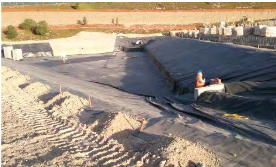
Caption Completion of lining installation for retention basin.
