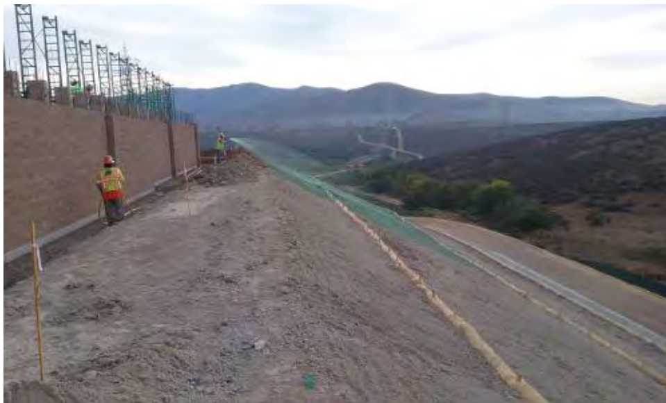
Caption Hydromulch application on slope.
