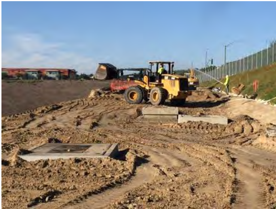
Caption Back-filling around handhole vaults in access road.
