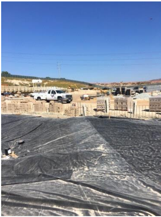
Caption Storm drain install
