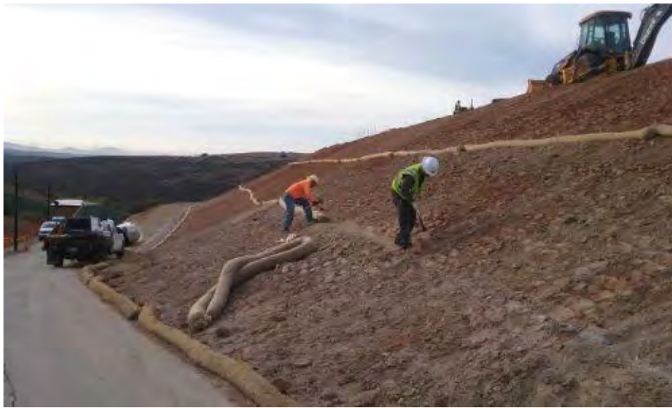
Caption Installation of straw wattles on slope.
