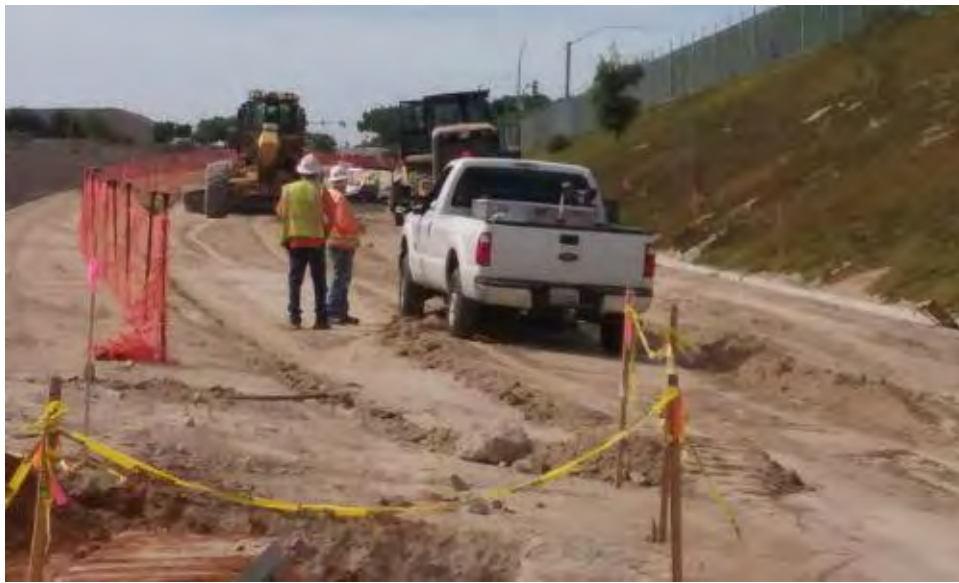
Caption Construction workers with idling graders in background.
