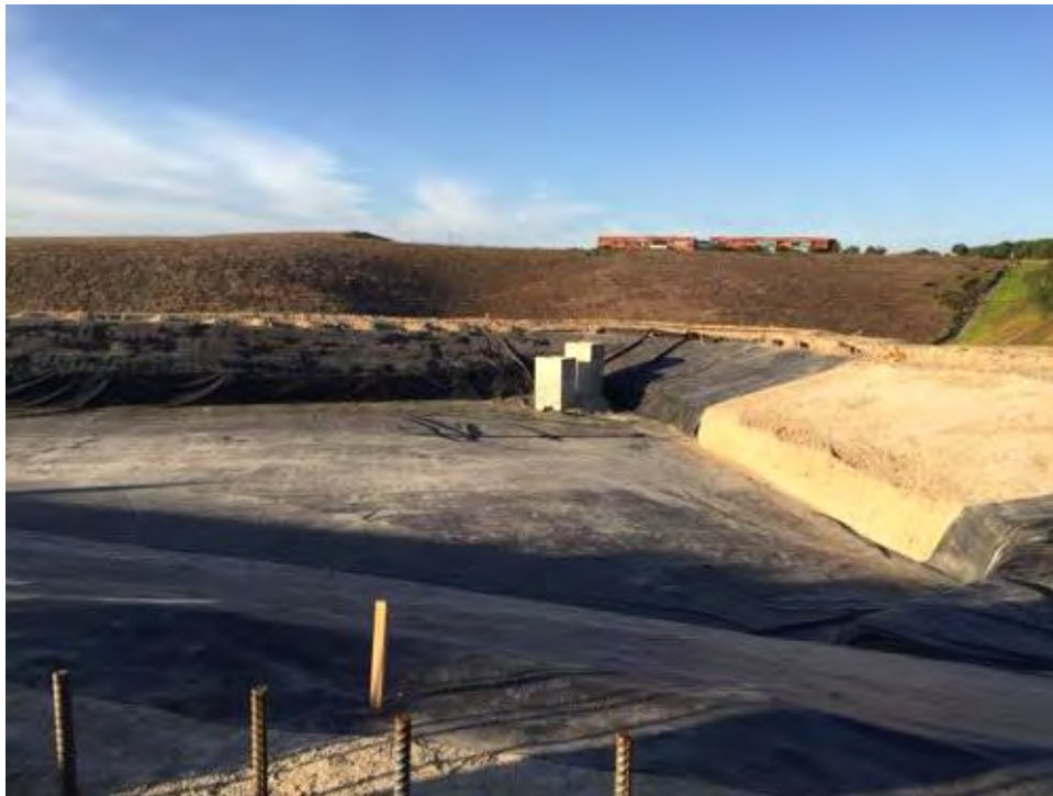
Caption Lining in bioretention basin
