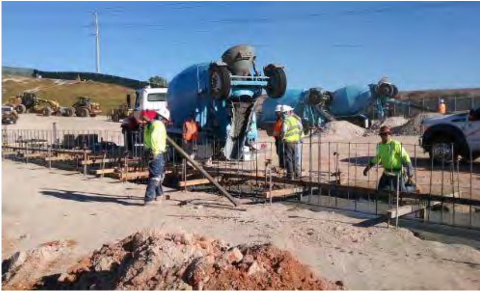
Caption Concrete pour for screening wall.
