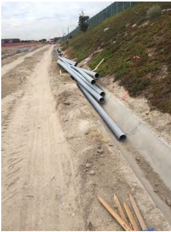
Caption Conduit pipes in drainage ditches.
