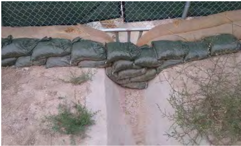
Caption Brow ditch outlet at western end of site.
