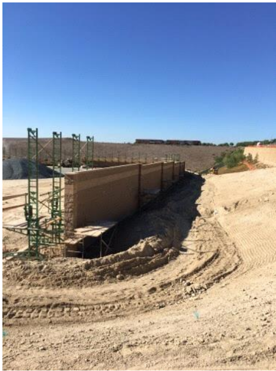
Caption Perimeter site masonry wall
