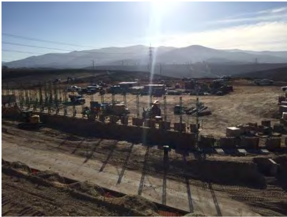
Caption Masonry wall and substation pad.
