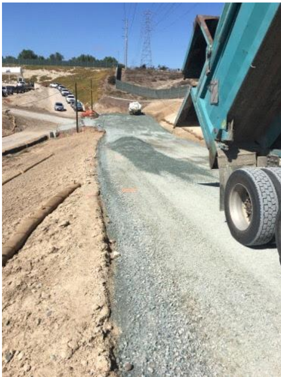
Caption Rock install along main access road
