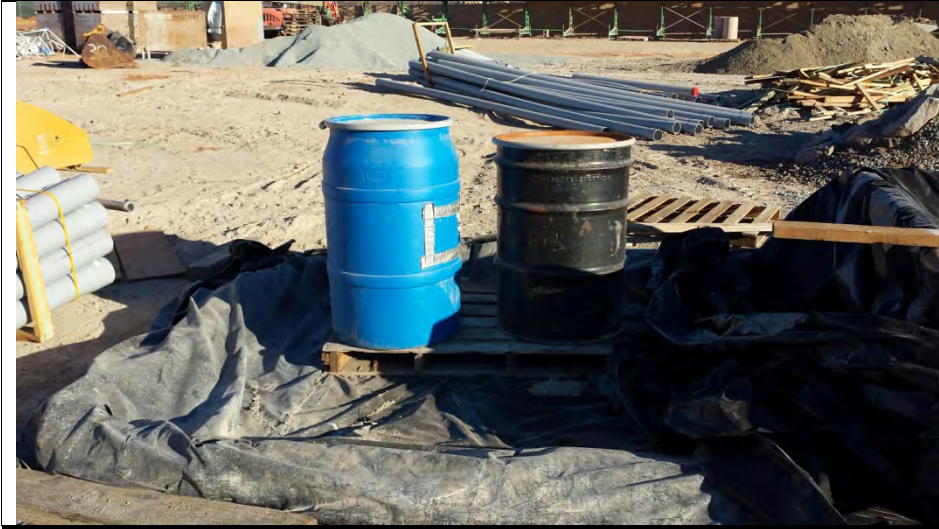
Photograph 3: 55-gallon containers with contaminated soil in secondary containment ready to be removed from the Salt Creek substation site, October 21, 2016.
