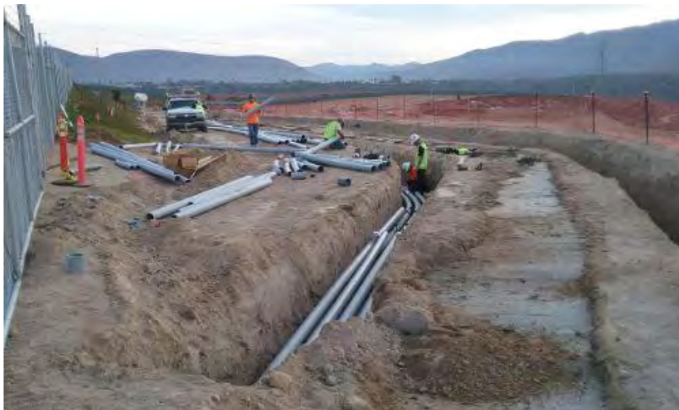
Caption Conduit installed in trench in entrance road.
