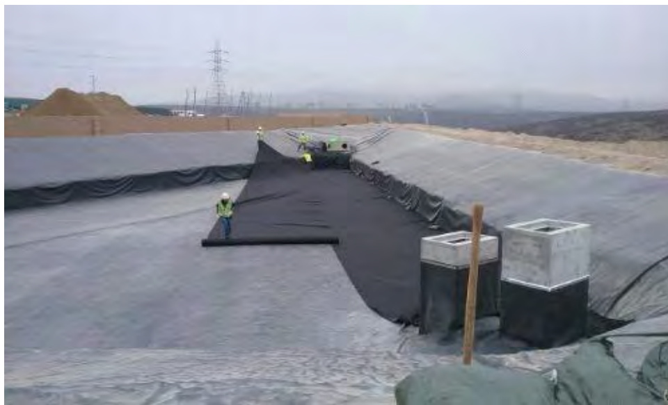
Caption Laying fiber rolls over liner in retention basin.
