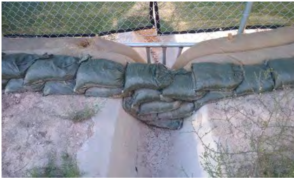
Caption No runoff off site from main culvert.
