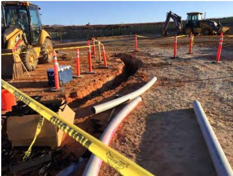
Caption Trenches for 12 kV get-away distribution lines.
