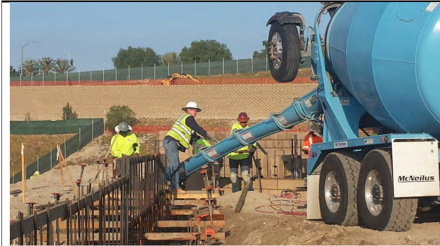
Photograph 1: Pouring foundation for the masonry wall during the week of October 15, 2016.
