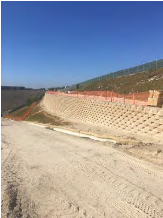
Caption Access road along northern portion of the site
