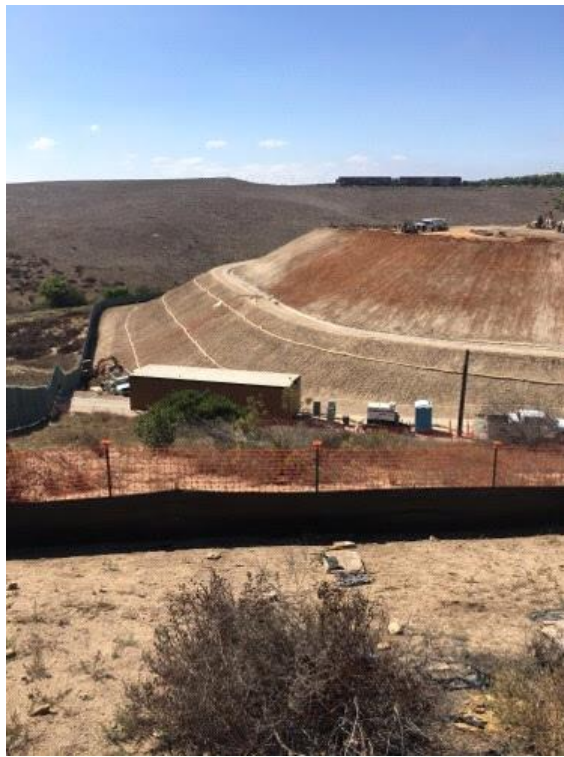
Caption Fiber install southern slopes
