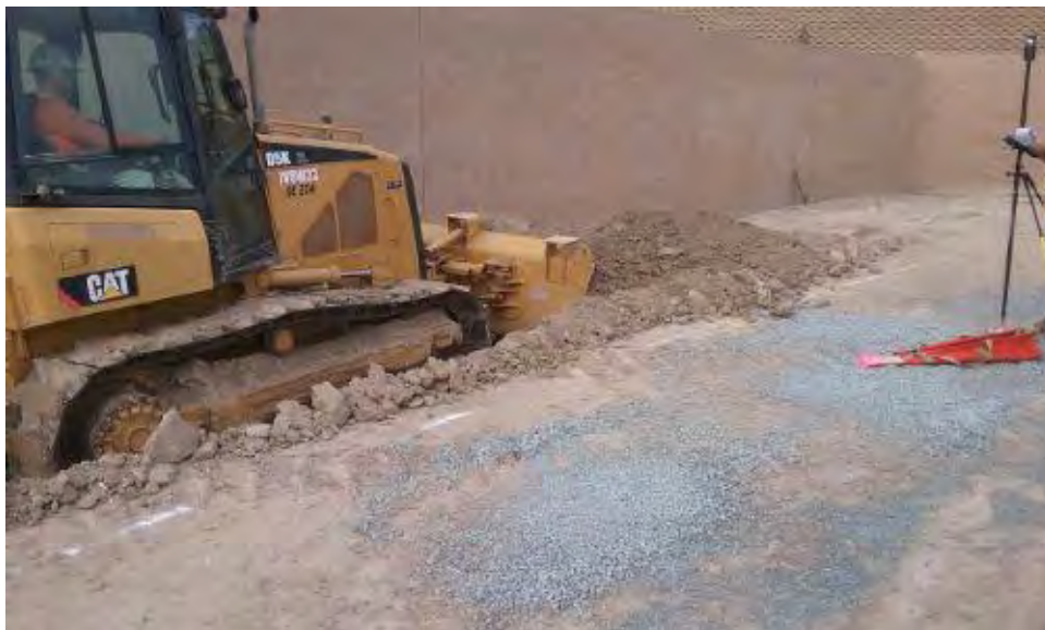
Caption Excavation for oil containment basin.
