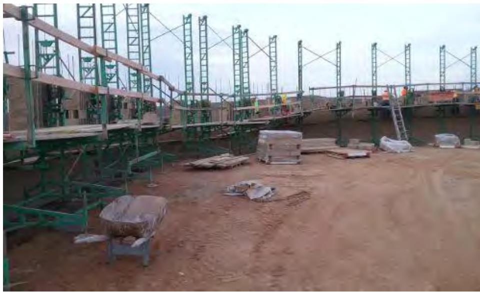
Caption Masonry screening wall construction.
