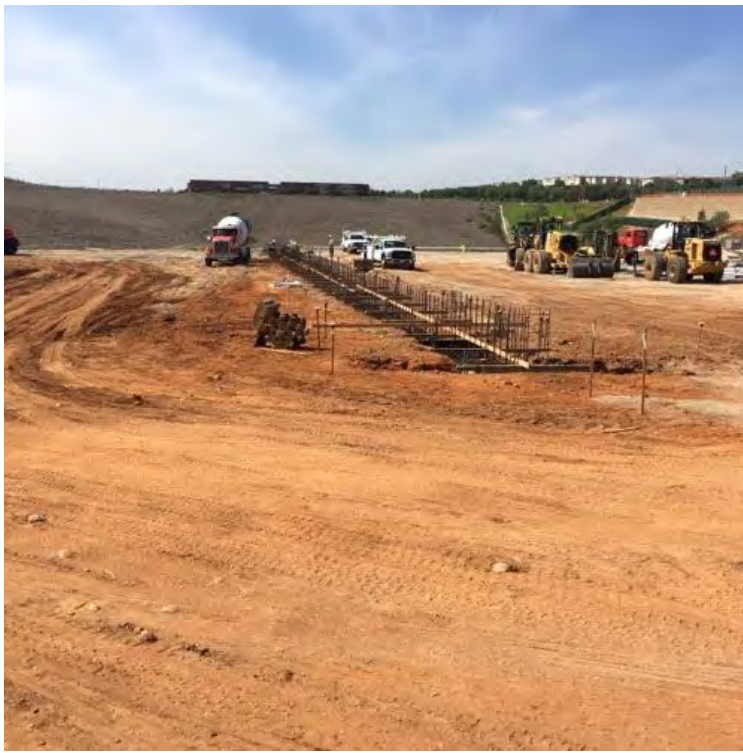
Caption Footings for masonry wall.
