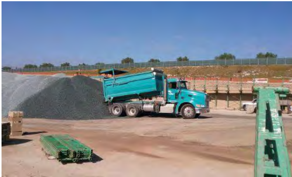
Caption Gravel delivery for retention basin.
