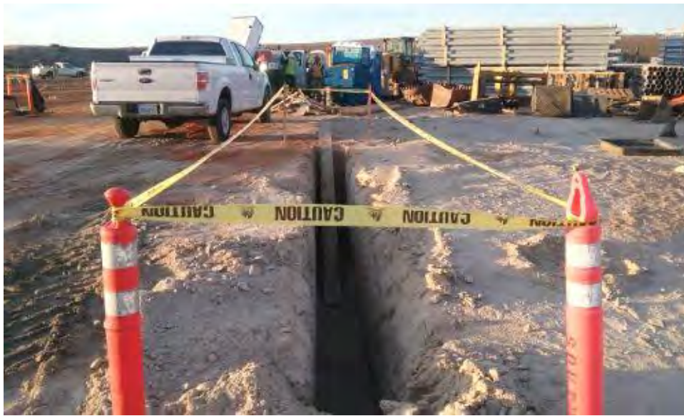
Caption Trench with animal exit ramp in place.
