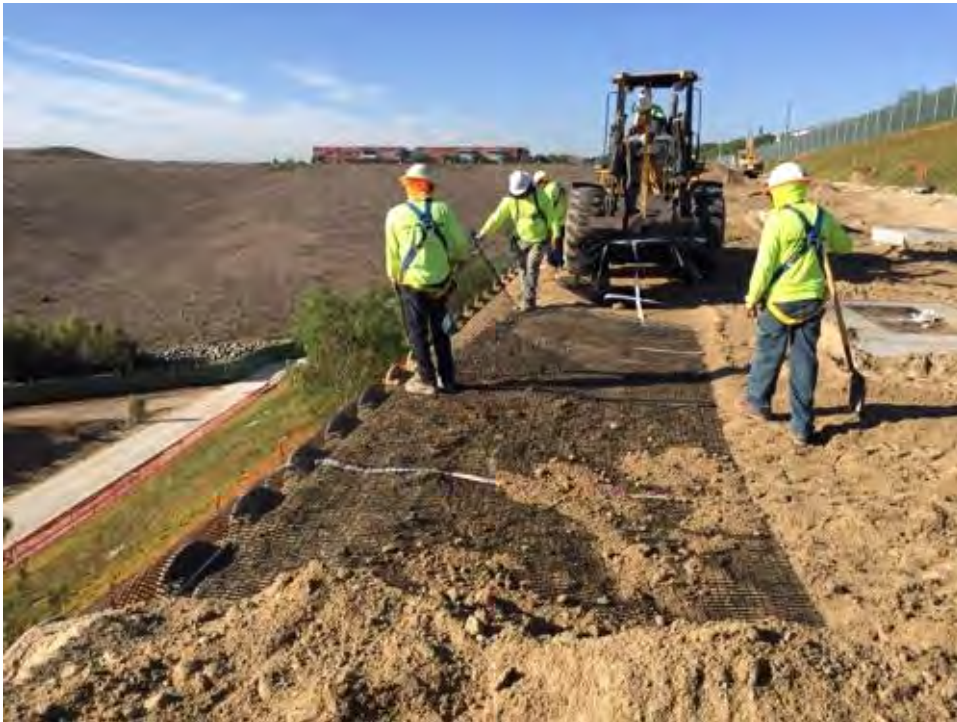
Caption Plastic mesh for Verdura wall stability.
