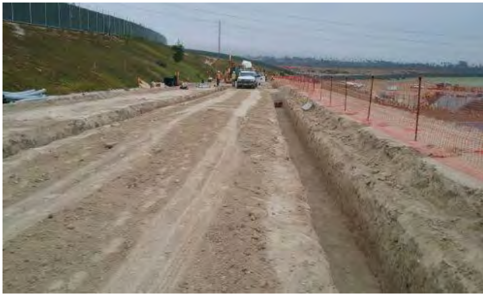
Caption Trenches for conduits in Hunte Pkwy access road.
