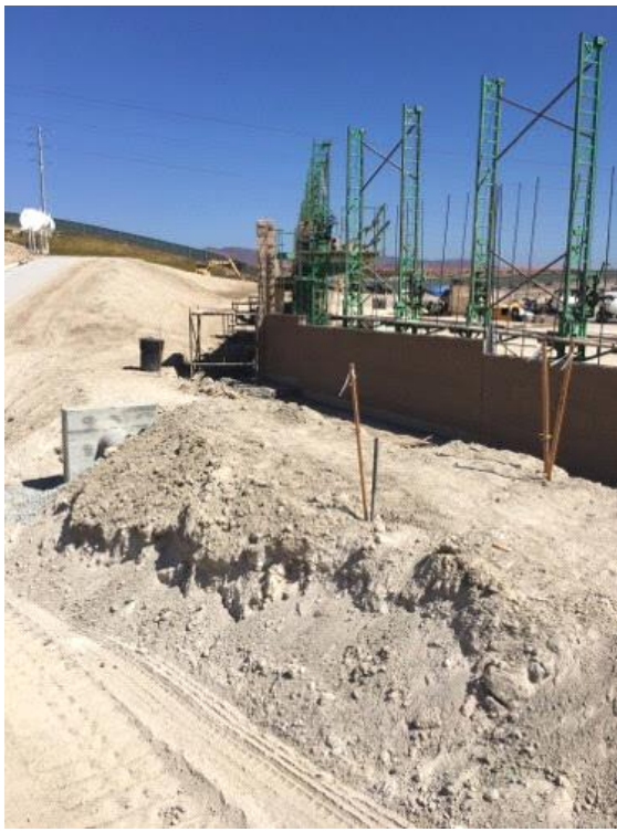
Caption Masonry wall install
