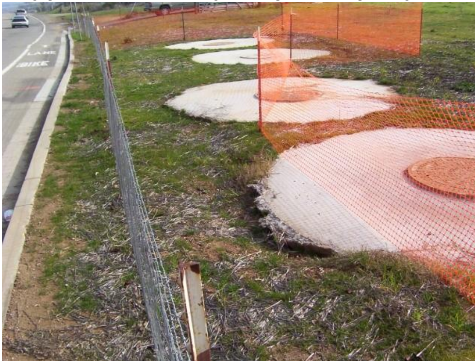
Photograph 2: Typical eight foot by eight-foot concrete apron poured around the vault lids to allow vault ingress and egress.
