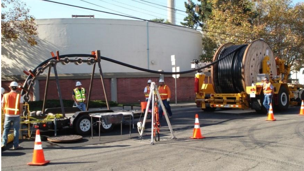
Photograph 7: Typical cable installation.
