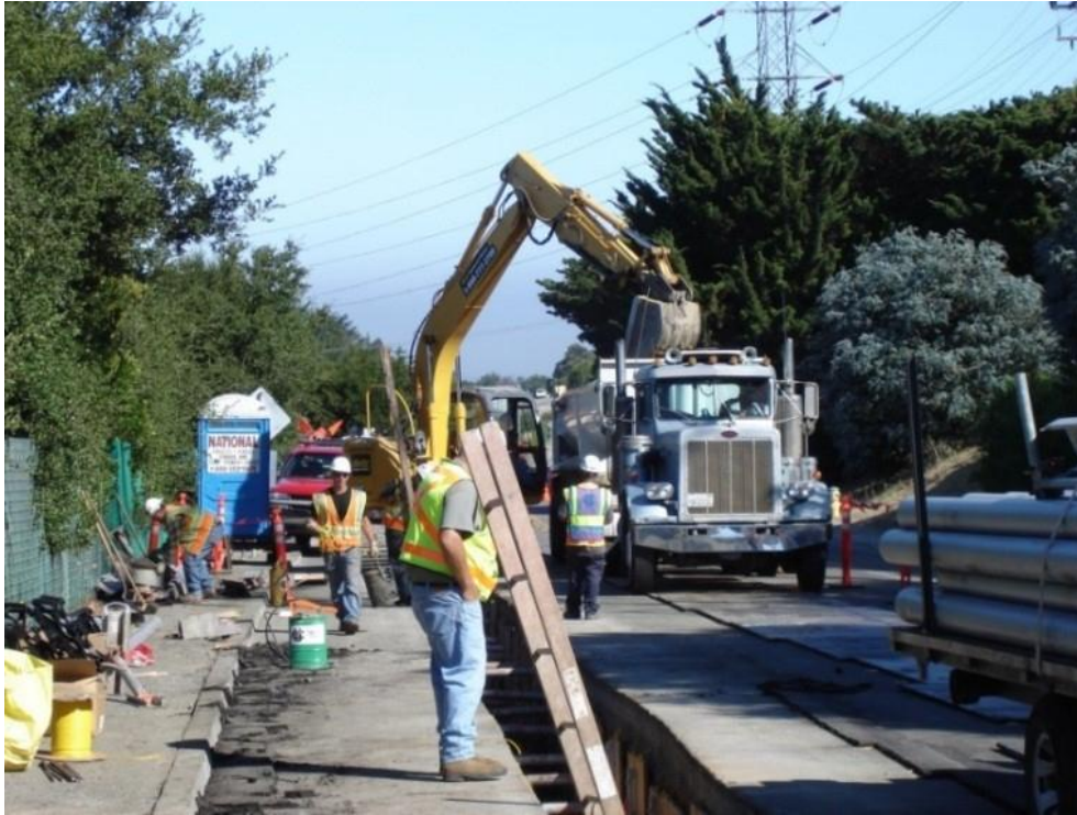
Photograph 5: Typical duct bank excavation with excavators. Dump trucks are positioned Parallel to the trench for extraction of soil.
