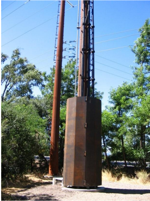
Photograph 1: Installation of a weathering steel riser pole with cable protecting shroud.
