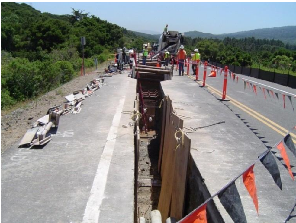
Photograph 6: Typical concrete duct bank installation.
