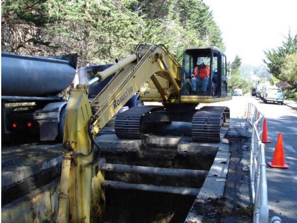
Photograph 3: Typical vault excavation within a public road.
