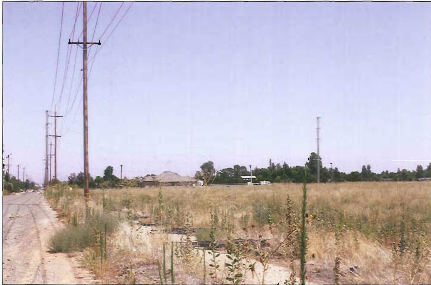
East Copper Avenue -- This simulation depicts the proposed power line connecting to the existing 115 kV power line parallel to East Copper Avenue. This view is east from the intersection of Sunnyside Avenue and East Copper Avenue. Based upon preliminary designs, the structure along Copper Avenue is depicted at approximately 85 feet tall; other structures are depicted at approximately 95 feet tall.
