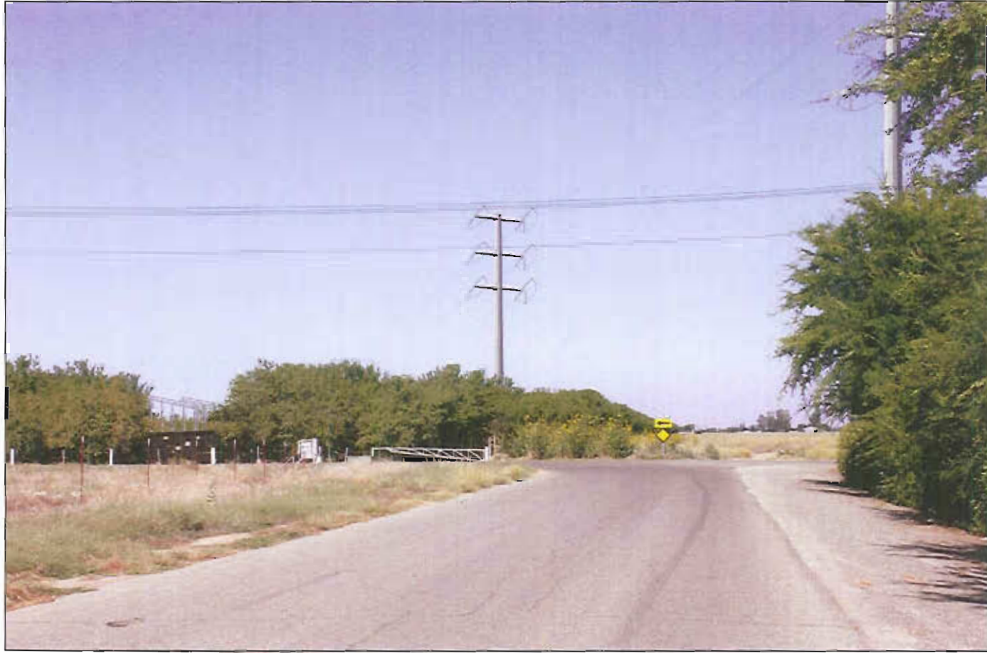
East of Sunnyside Avenue along Perrin Road -- Nearby residences would have views of the proposed substation as well as the proposed power line from this viewpoint. The substation wall and entry gates are visible through the almond orchard. Based upon preliminary designs, the structure located within the background is depicted at approximately 75 feet tall, and the turning structure is depicted at approximately 95 feet tall.
