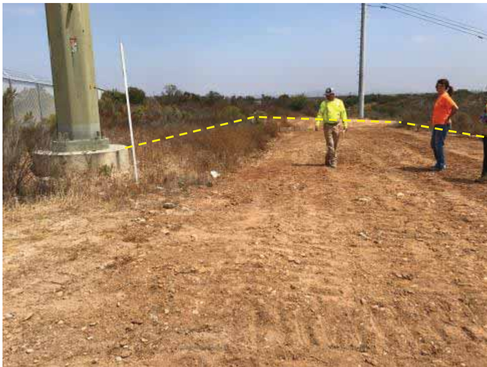
Photo 22. North-facing view of work area associated with Z479049.
