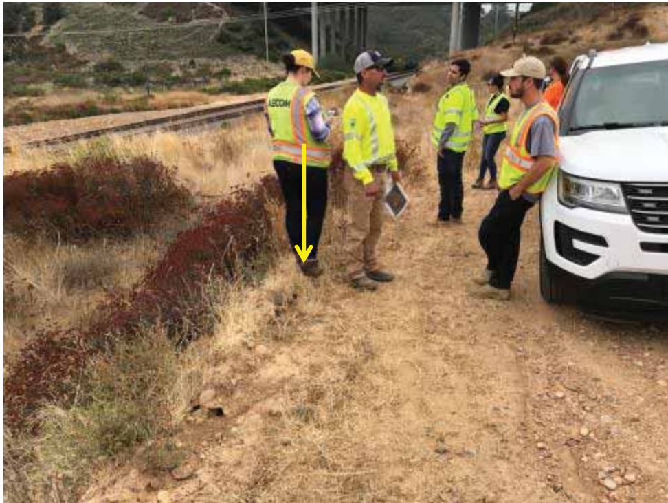
Photo 49. West-facing view of east pole location for GS-24.
