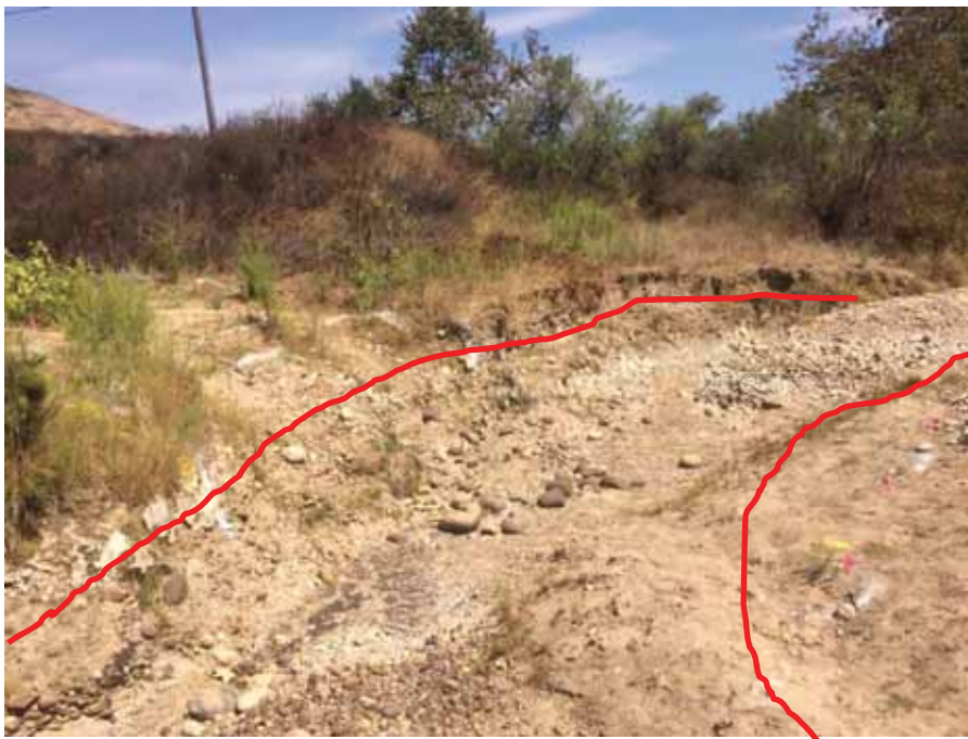
Photo 2. Photo (facing east) of Rose Creek drainage. Pink pin flags denote the limits of the steel plate. CDFW limits are denoted by red lines.
