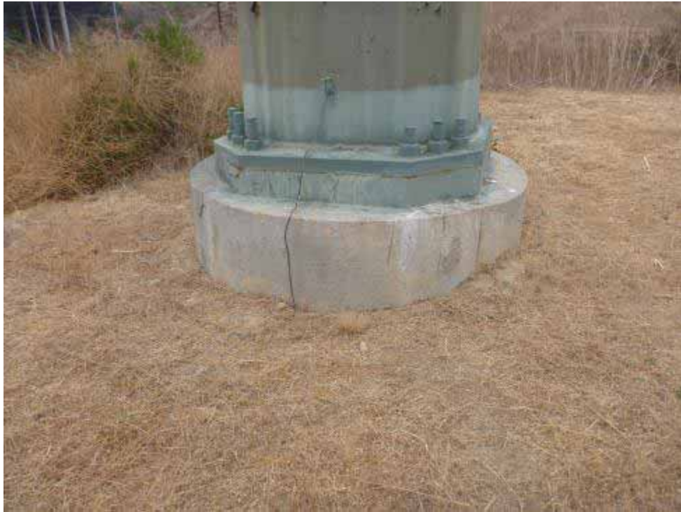
Photo 9. North-facing view of Z479044.
