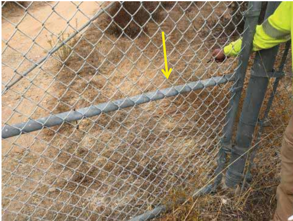
Photo 52. North-facing view of northwest pole location for GS-27.
