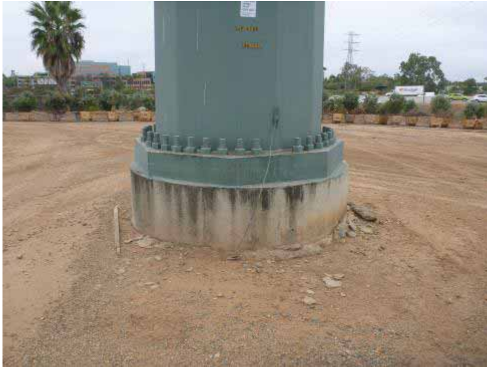
Photo 1. North-facing view of Z479040.
