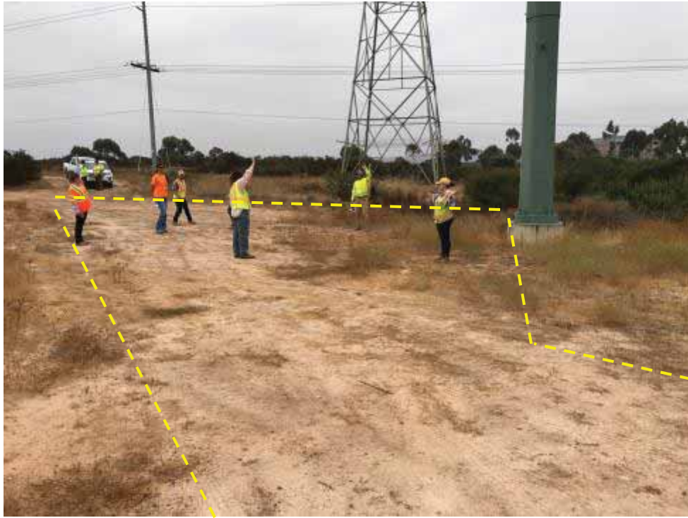
Photo 17. West-facing view of work area associated with Z479047.
