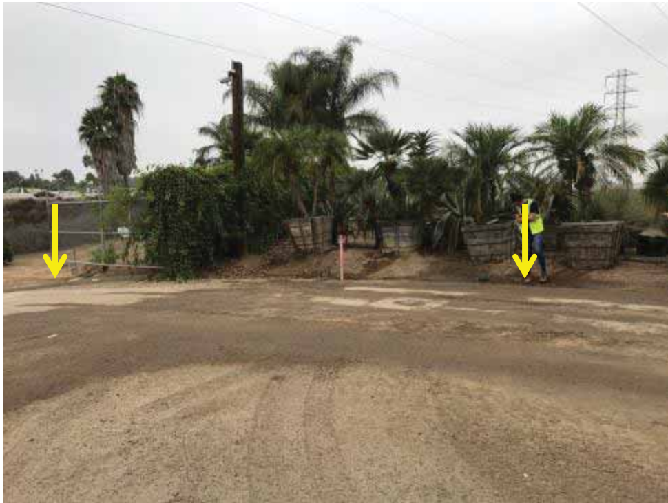
Photo 39. Northwest-facing view of GS-20 (yellow arrows indicate pole locations).
