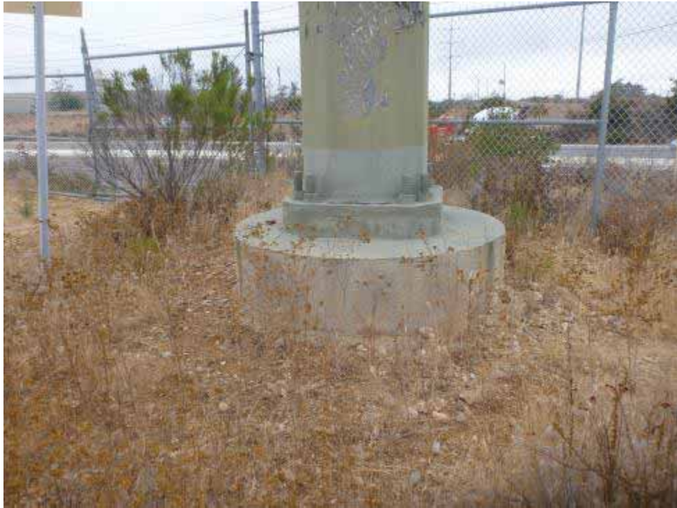
Photo 21. North-facing view of Z479049.
