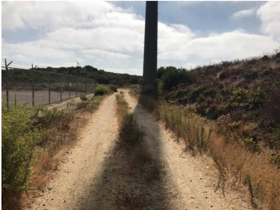
Figure 2: East-facing view of existing structure 39 at the Peñasquitos Substation.
