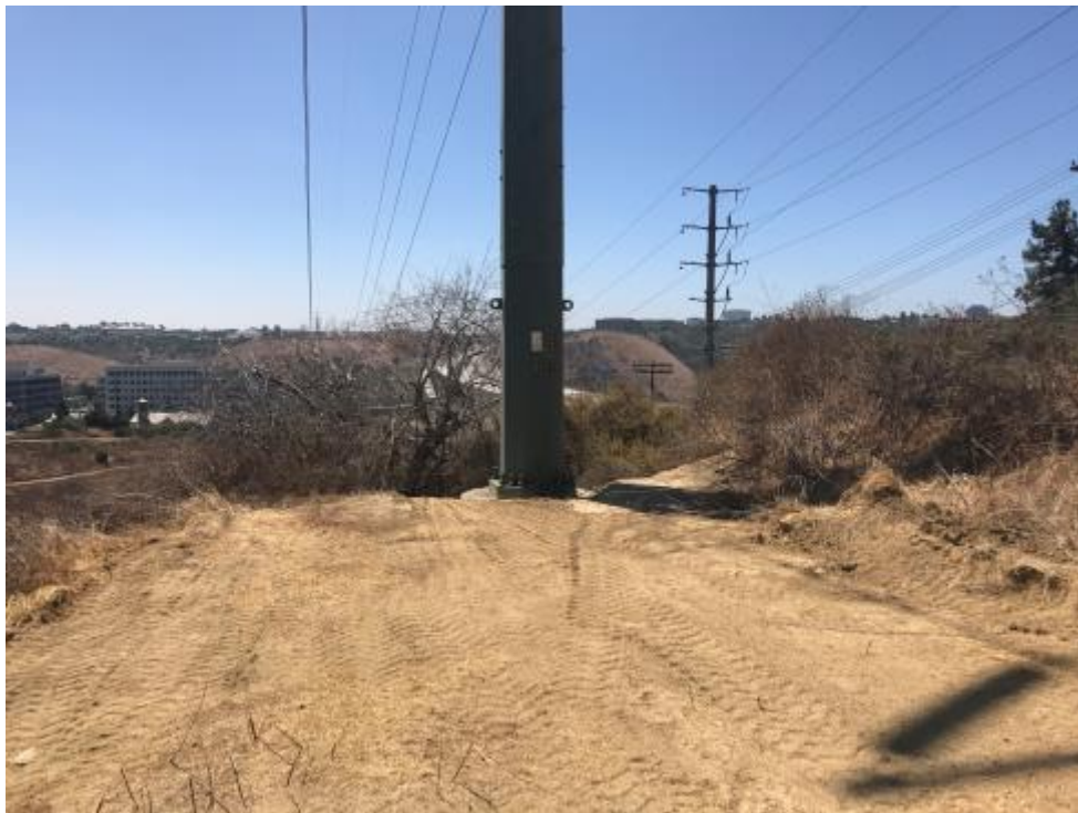
Figure 20: South-facing view of existing structure 47.
