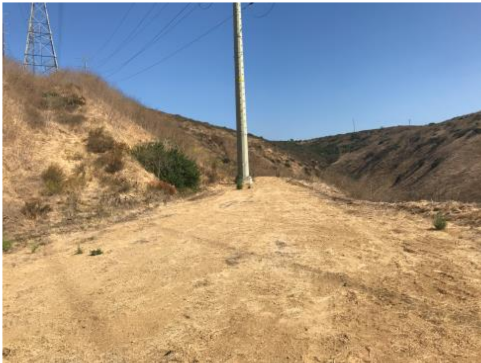
Figure 8: North-facing view of existing structure 42.
