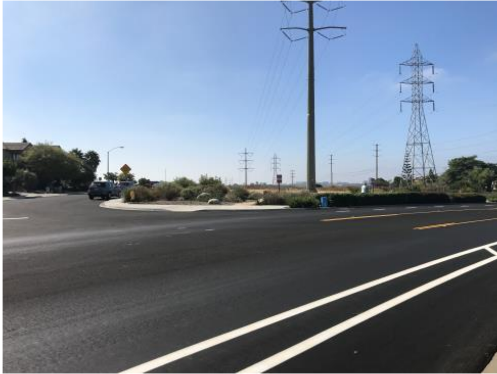
Figure 5: Southeast-facing view of GS 2 location from East Ocean Air Drive.
