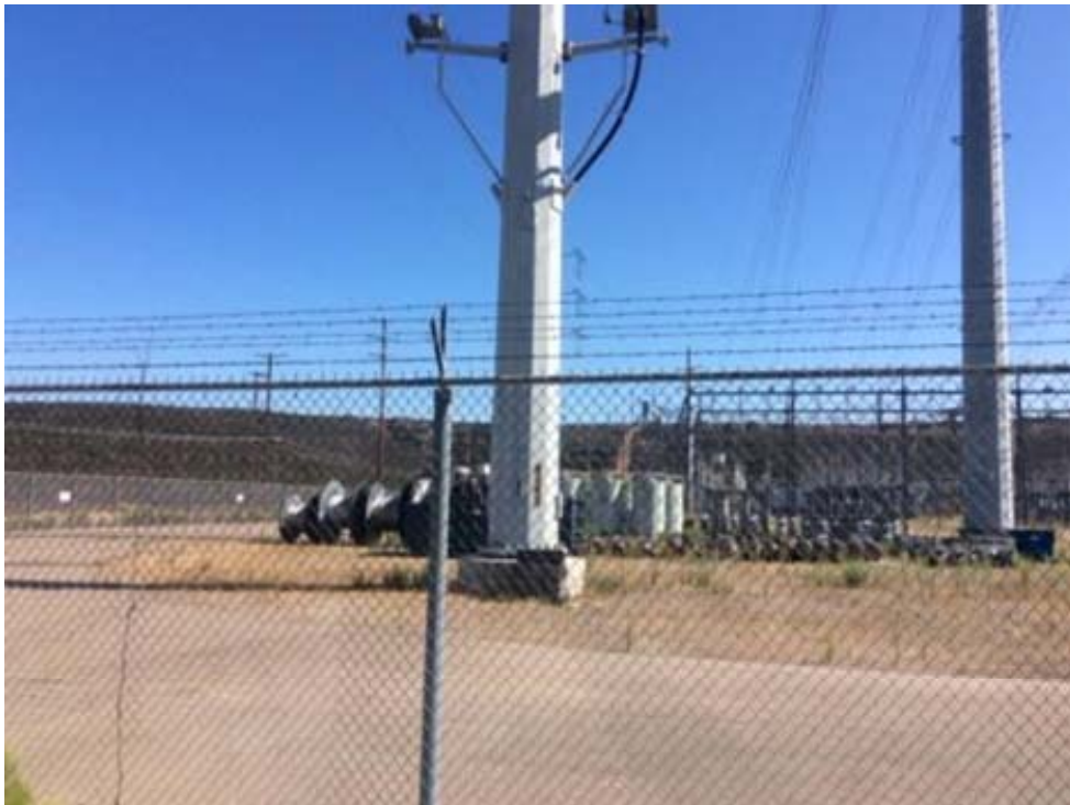
Figure 34: South-facing view of structure R01 to be removed.
