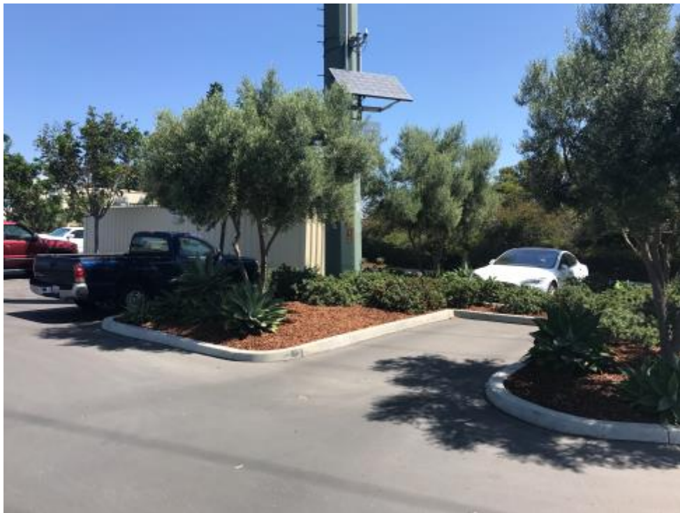
Figure 18: East-facing view of existing structure 46.
