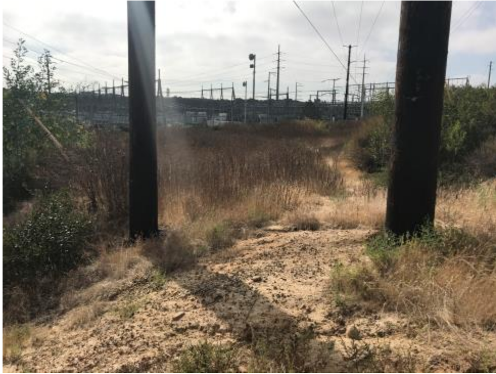
Figure 1: East-facing view of alternating current (AC) mitigation site location northwest of the Peñasquitos Substation.
