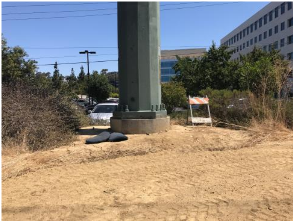
Figure 26: East-facing view of existing structure 48.
