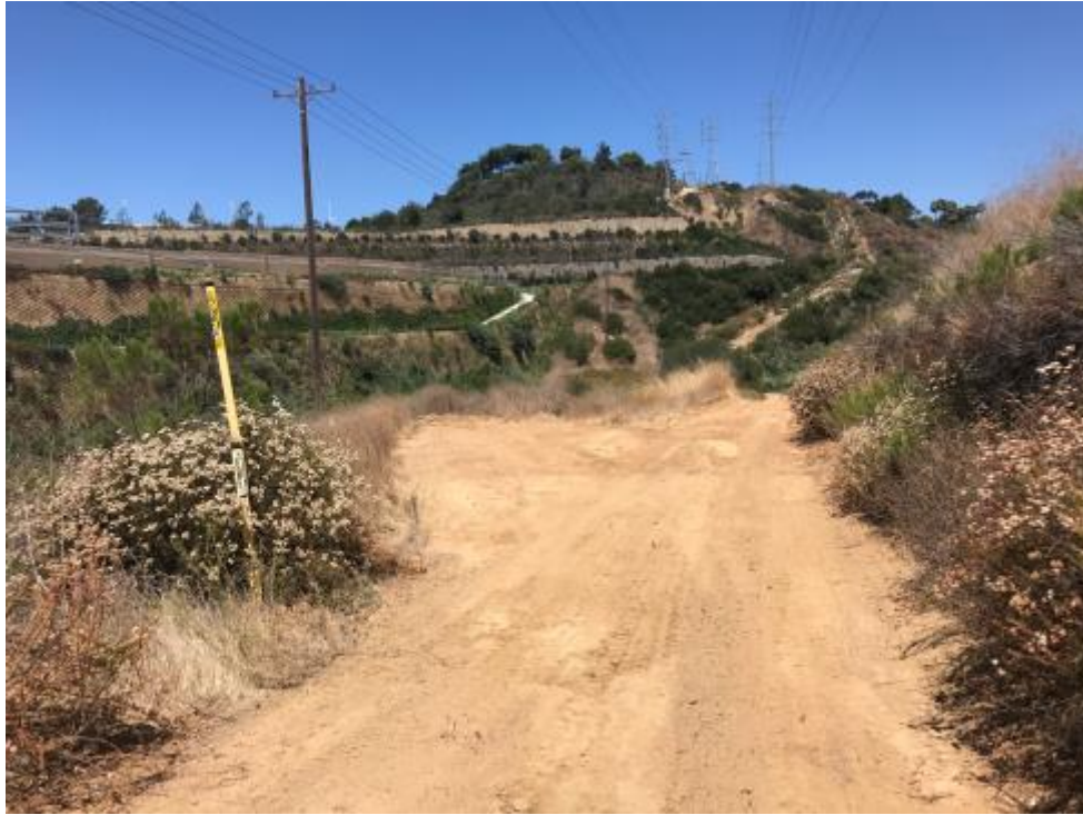
Figure 25: North-facing view of ADSS interset structure north of Mira Mesa Blvd.
