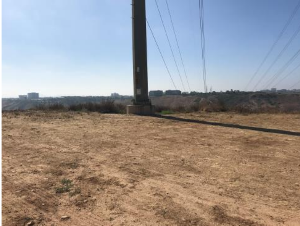
Figure 7: Southeast-facing view of existing structure 41.
