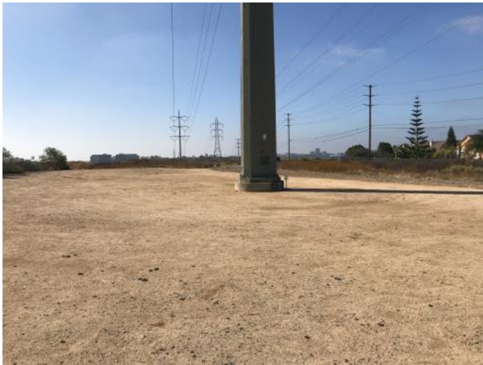
Figure 6: South-facing view of existing structure 40.
