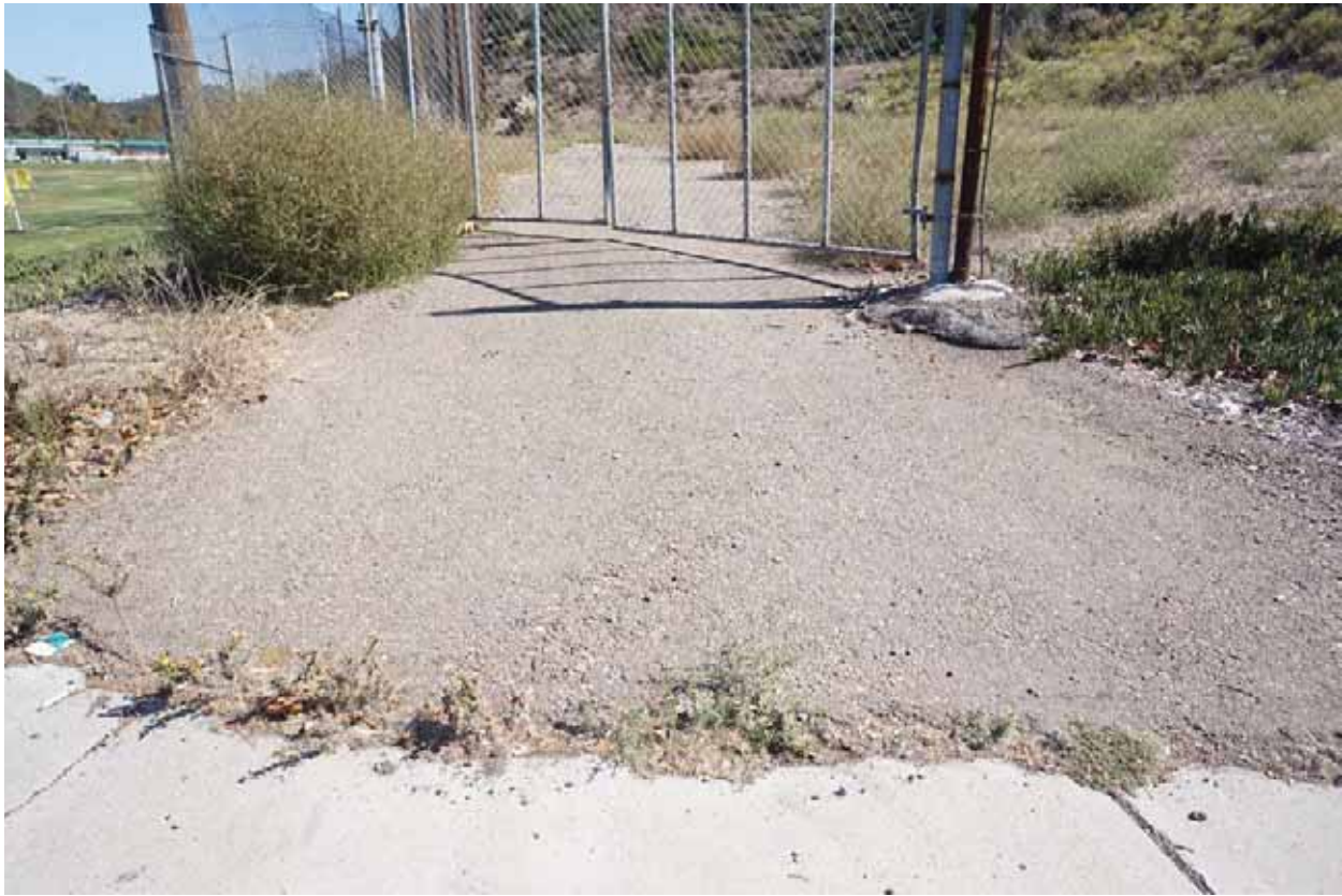
Driving Range Yard Photo taken 11/17/2016
