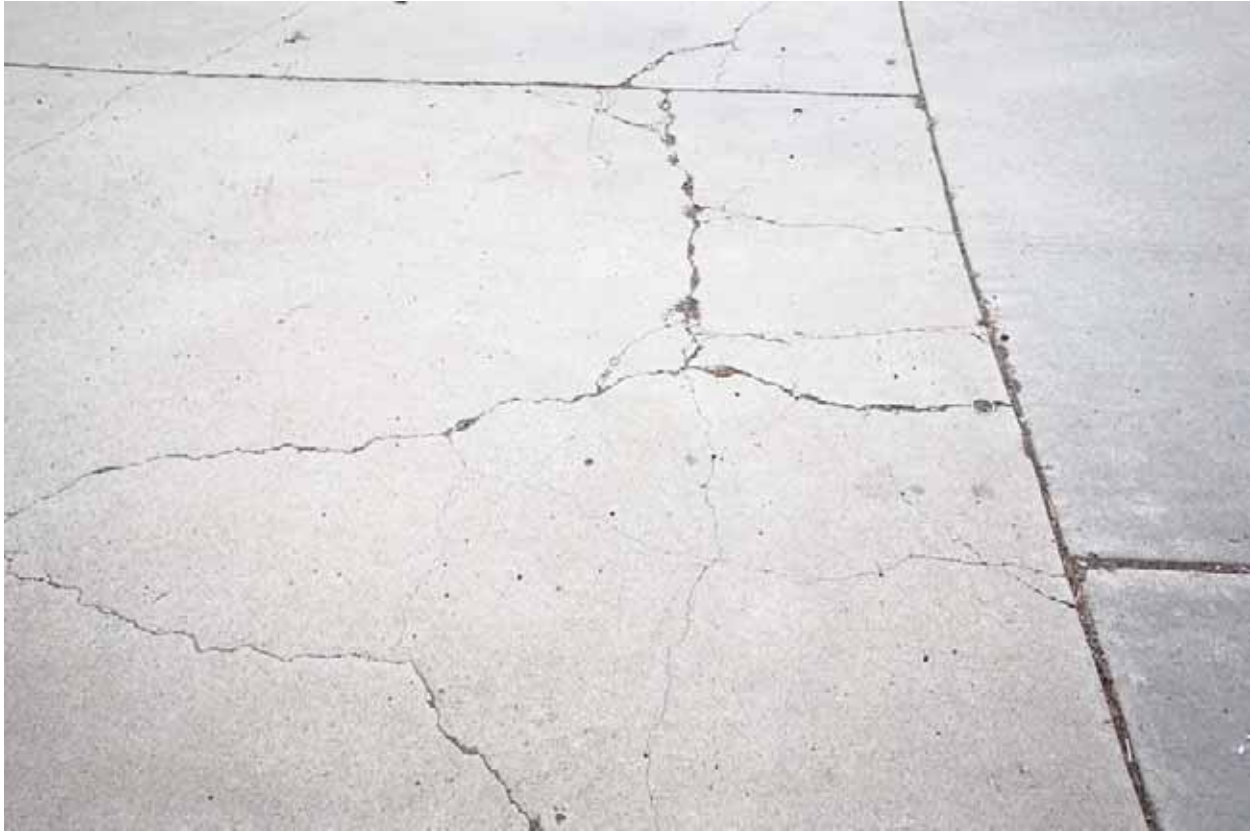
Driving Range Yard Photo taken 11/17/2016
