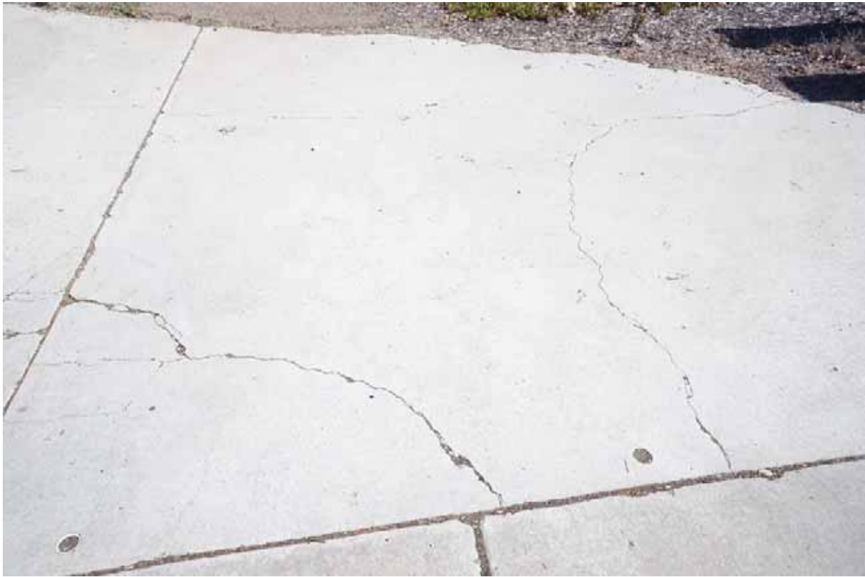
Driving Range Yard Photo taken 11/17/2016
