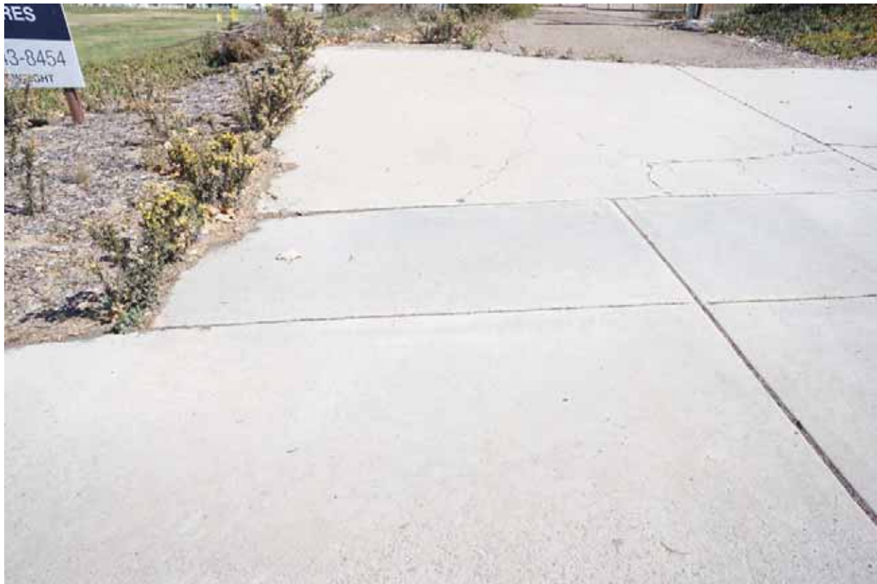
Driving Range Yard Photo taken 11/17/2016
