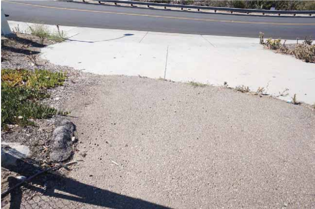
Driving Range Yard Photo taken 11/17/2016
