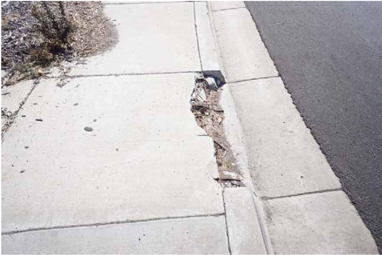
Driving Range Yard Photo taken 11/17/2016
