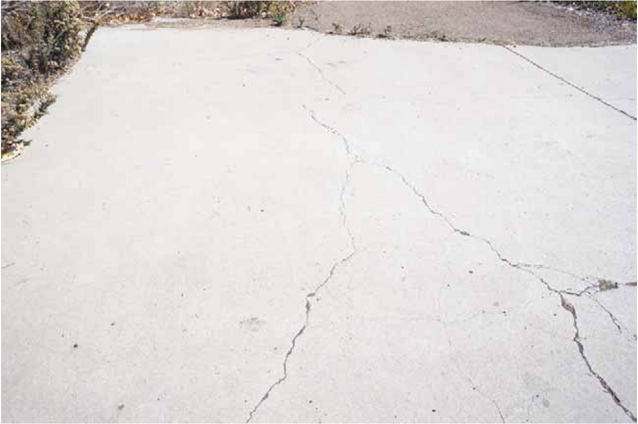
Driving Range Yard Photo taken 11/17/2016
