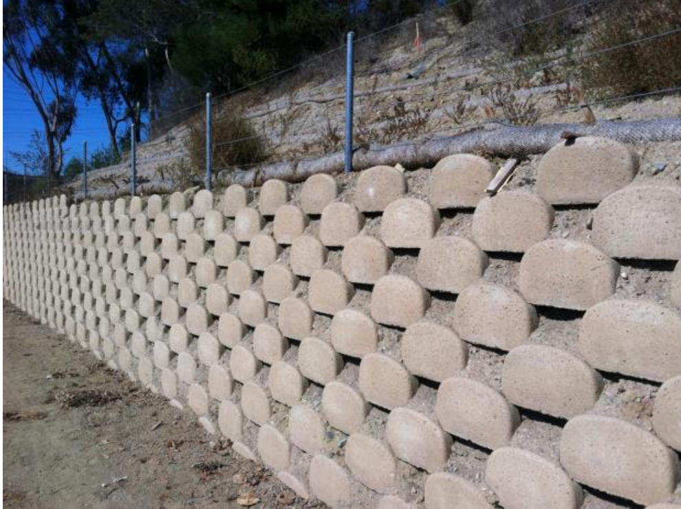
Figure 2.4-2: Typical Retaining Wall Face
