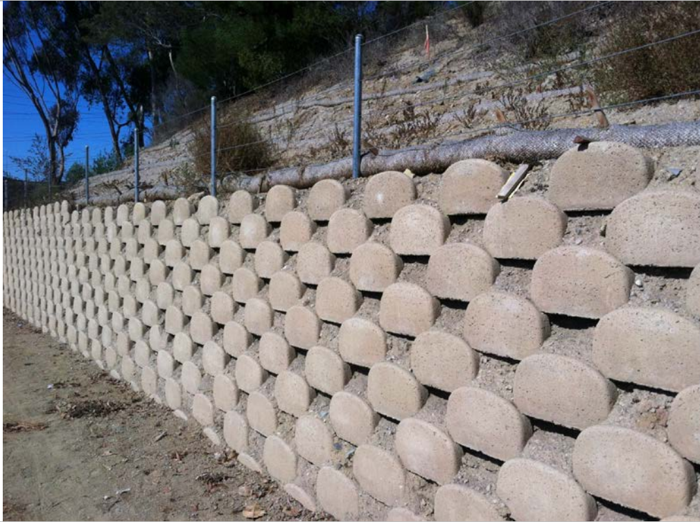
Figure 2.4-2: Typical Retaining Wall Face
