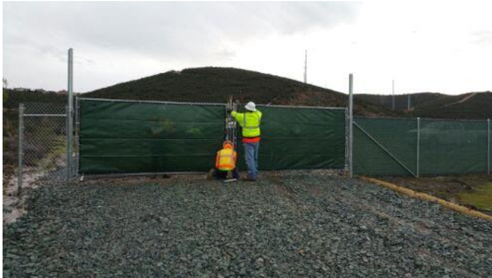
Caption Gate installation, Stonebridge.
