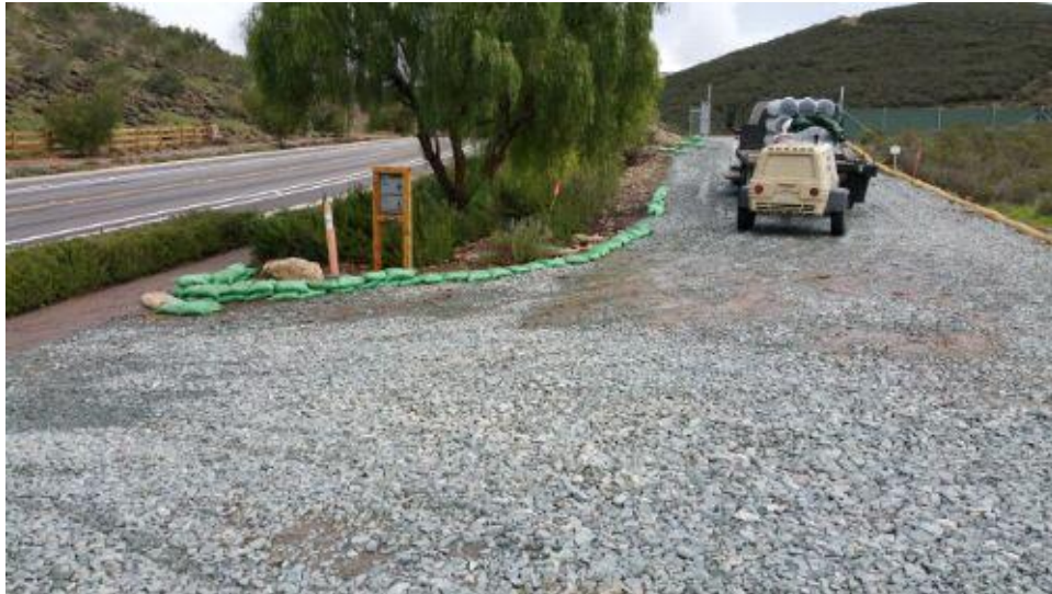
Caption BMPS installed around disturbed area. Stonebridge.
