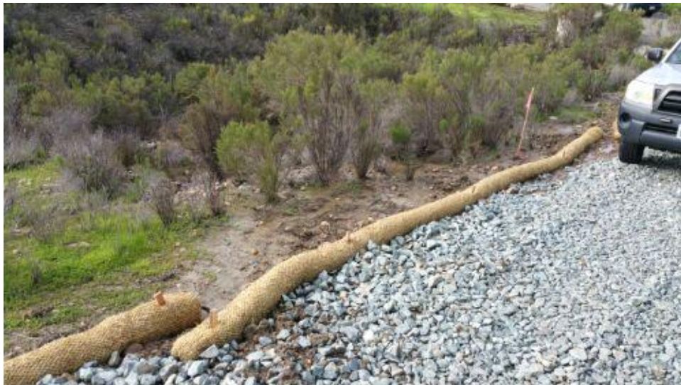
Caption Diverted flow directed to detention basin. Stonebridge.
