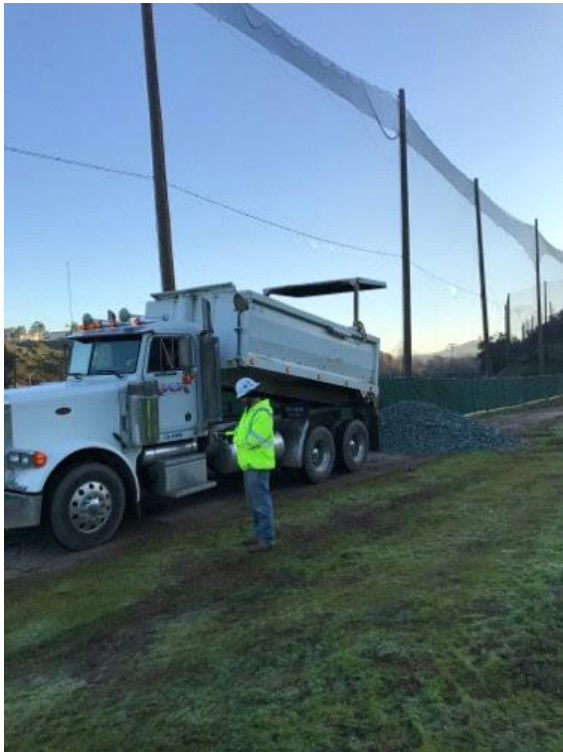
Caption Rock for apron at entrance at Driving Range Yard.
