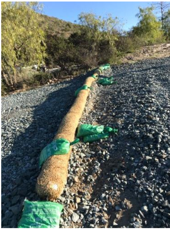
Caption Swale created to divert flows on access road at Stonebridge Yard.
