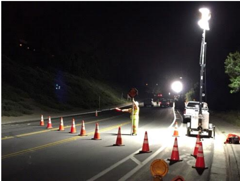
Caption Lighting, cones, signage, and traffic flaggers in place
