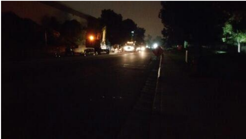
Approach to staging area on Trade St. from east. Plates being delivered ; no flagger present, but this is compliant per Safety Officer (equipment properly lit).
