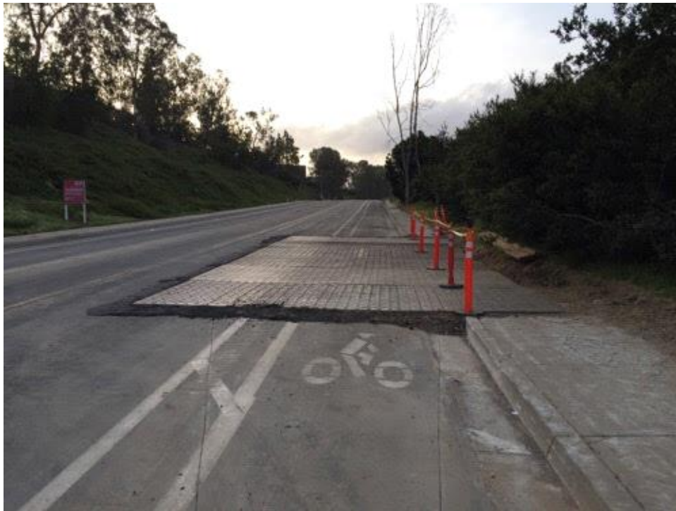
Caption Steel plates in place covering trenches.
