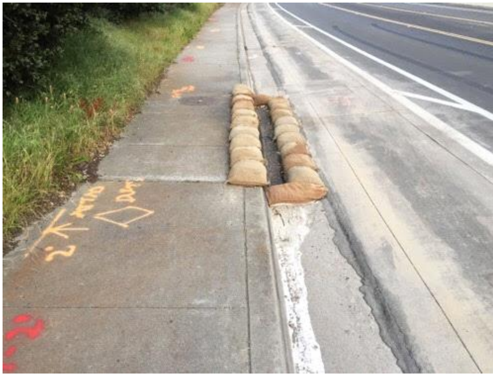
Caption BMP's in place for SWPPP.
