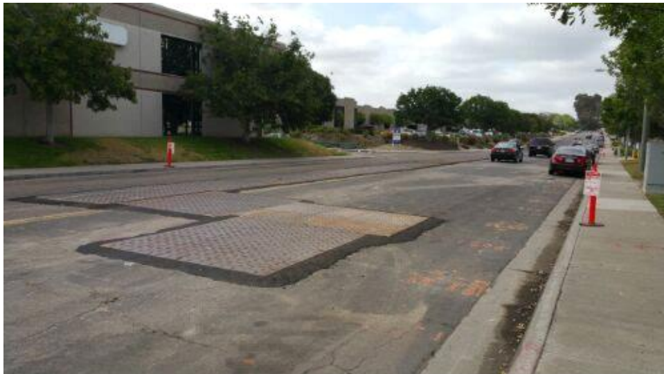
Caption Trench plates at Trade PI. site; traffic moving freely.
