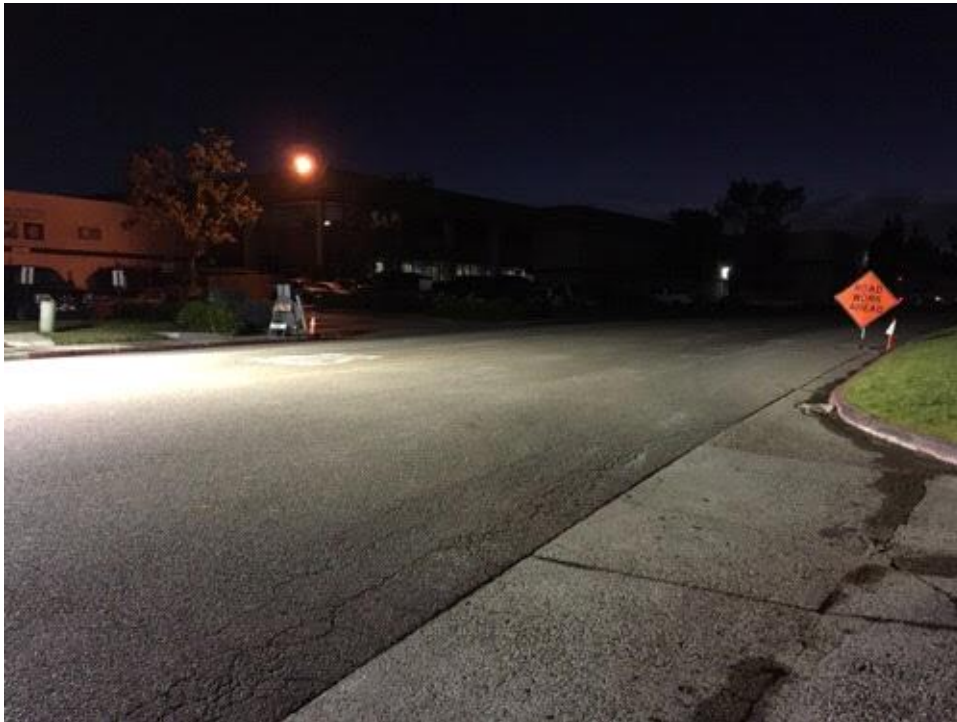
Caption Adequate lighting and signage in place.
