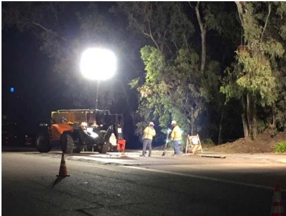
Caption Abundant lighting in place for work.
