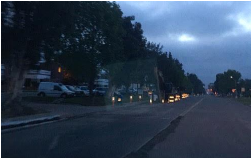
Caption Arjons work site. Traffic flowing and work is complete.
