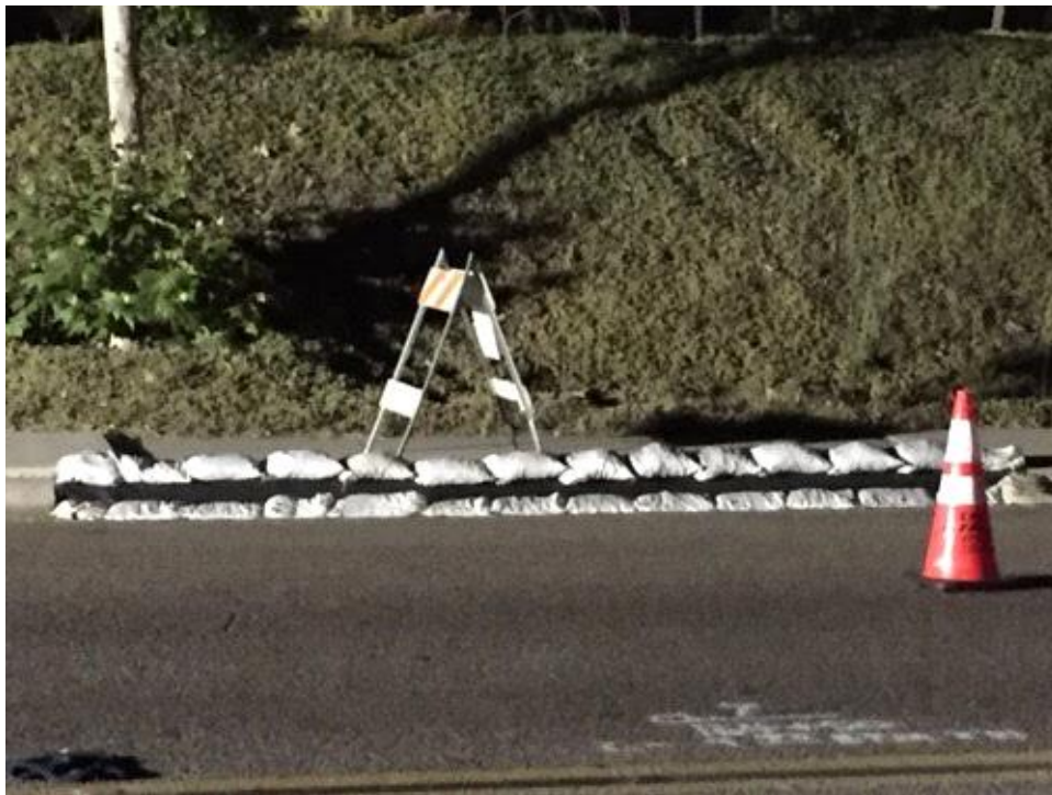
Caption BMPs in place.
