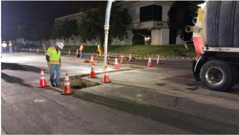
Placing protective barriers around trench (Trade Pl.).
