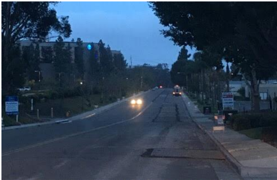
Caption Trade place work site. Traffic flowing and work complete.
