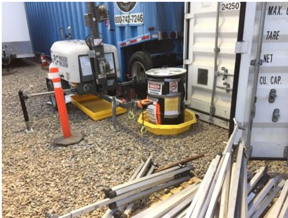
Caption Hazardous waste properly stored and labeled.
