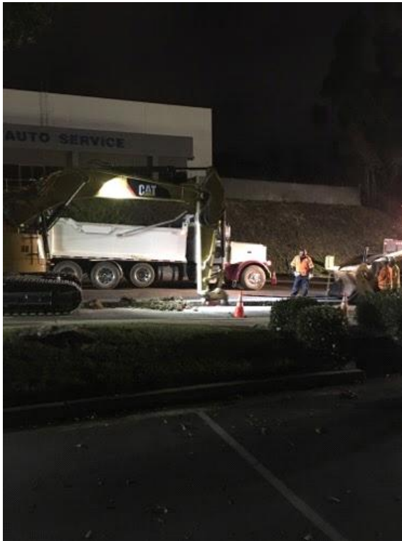
Caption Excavation on Trade Place
