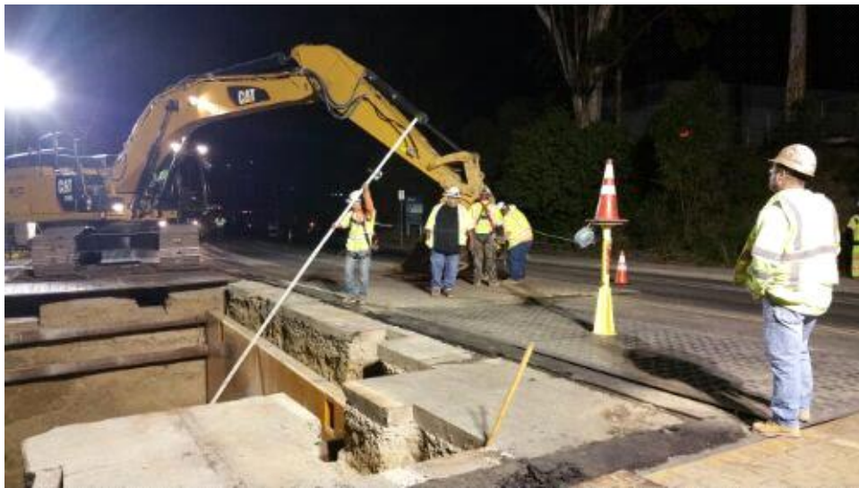
Caption Workers connected to anti-fall device near vault.
