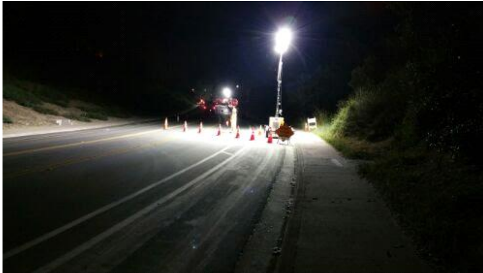
Caption Approach to Carroll Road site from west.
