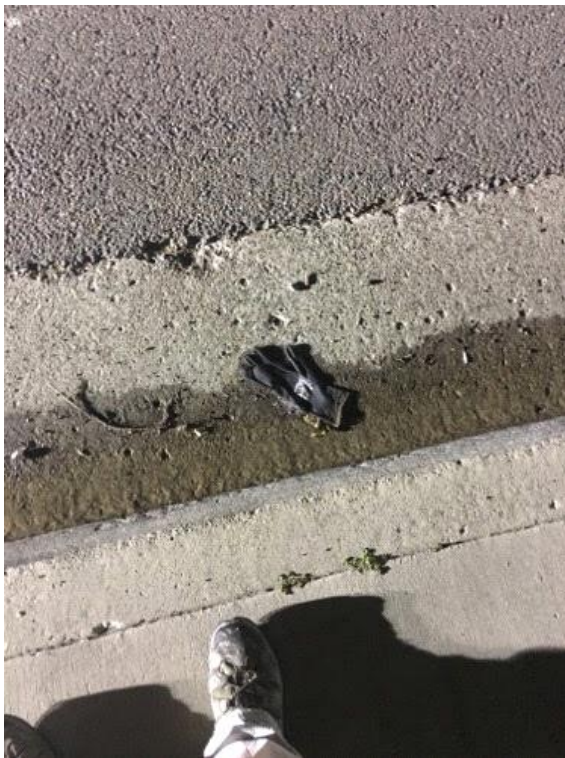
Caption Work site debris in gutters
