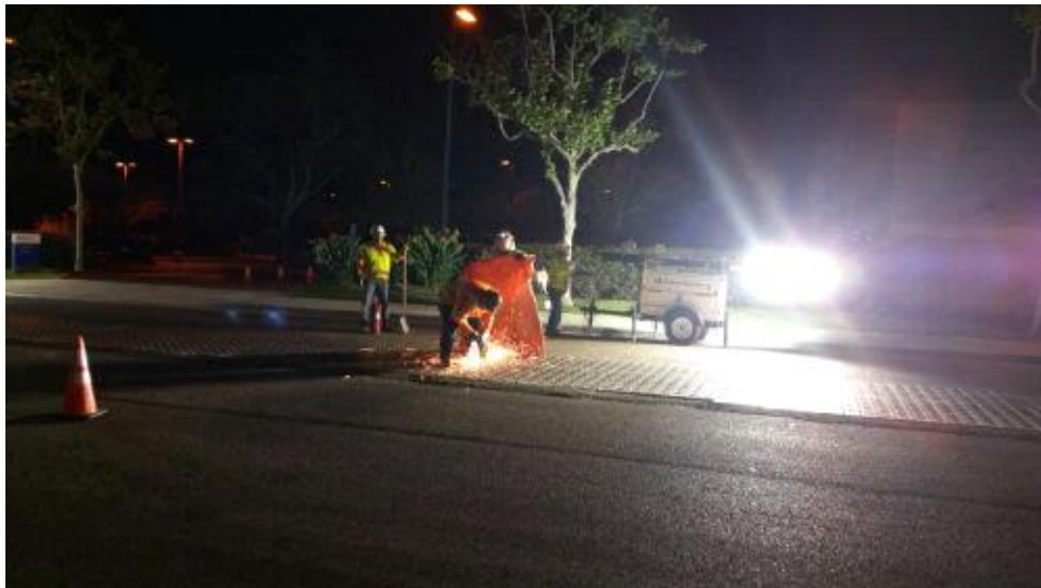
Caption Cutting trench plate with proper fire safety measures.
