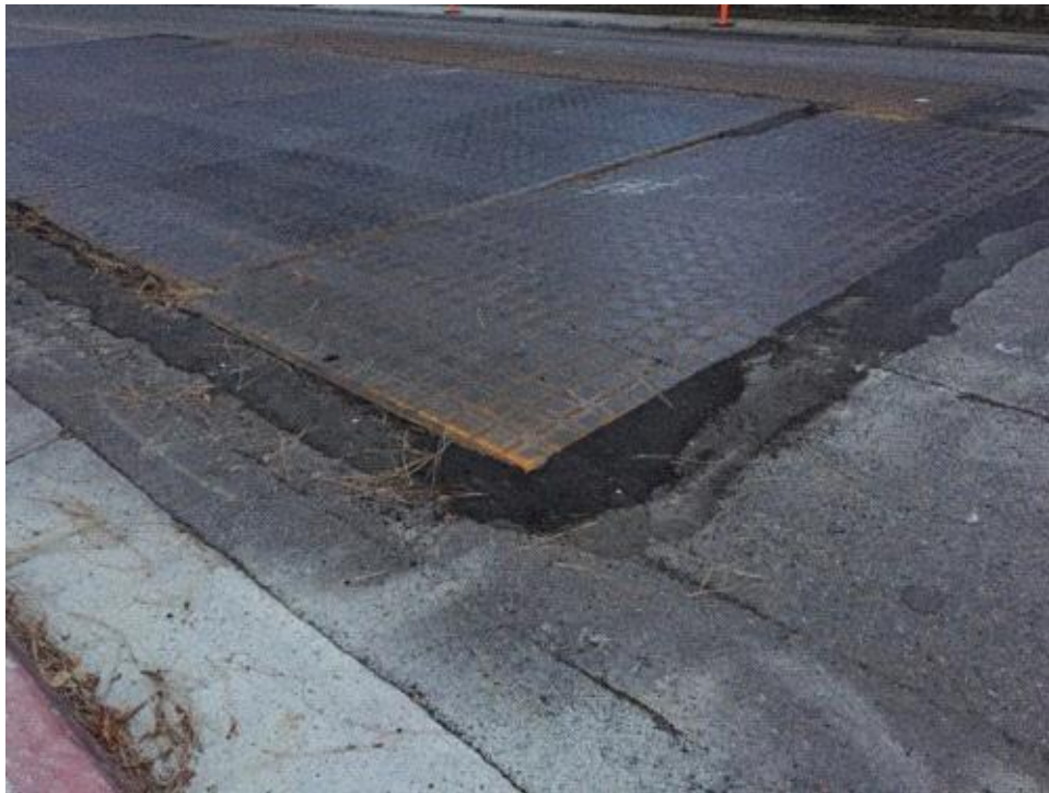
Caption Steel plates covering trenches and sealed with asphalt.
