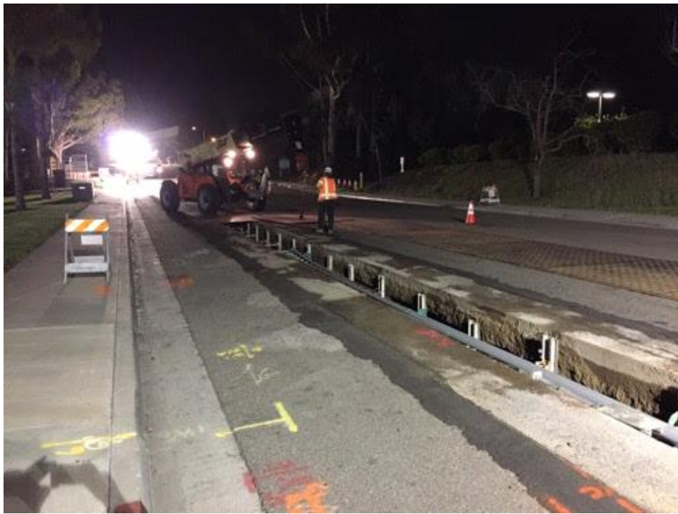
Caption Open trenches with clearly marked boundaries
