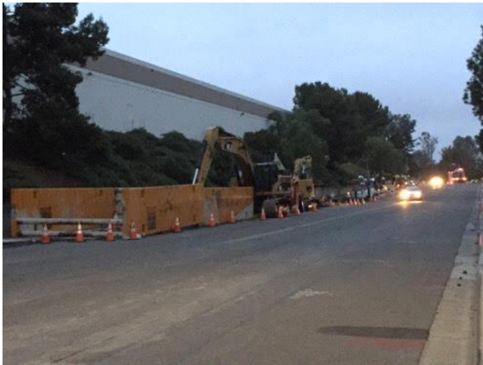
Caption Equipment returned to storage location and street is cleared.
