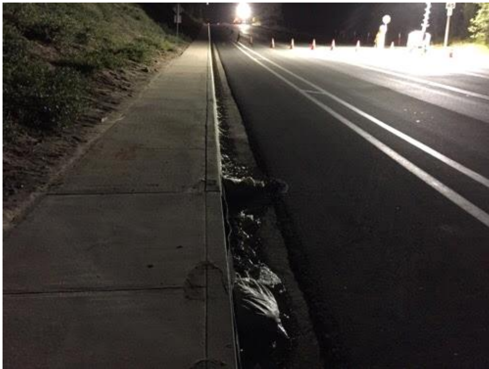
Caption BMPs in place and in good working condition.
