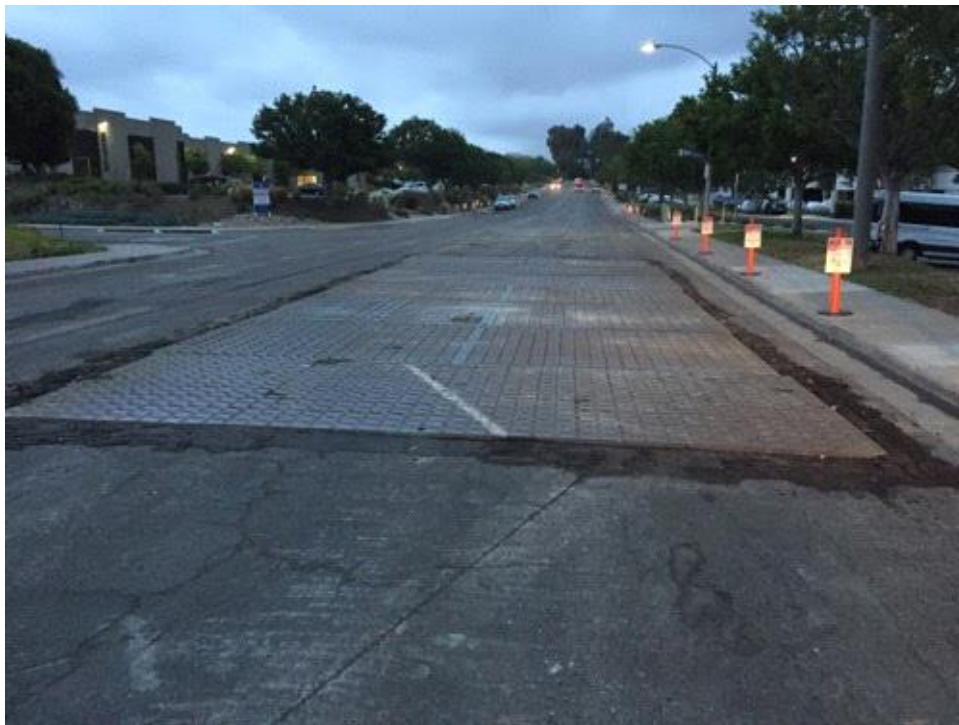
Caption Trenches covered with steel plates and capped with asphalt.
