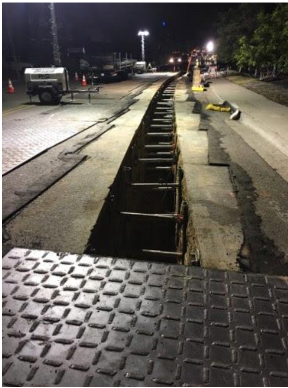
Caption Trade St open trench with shoring
