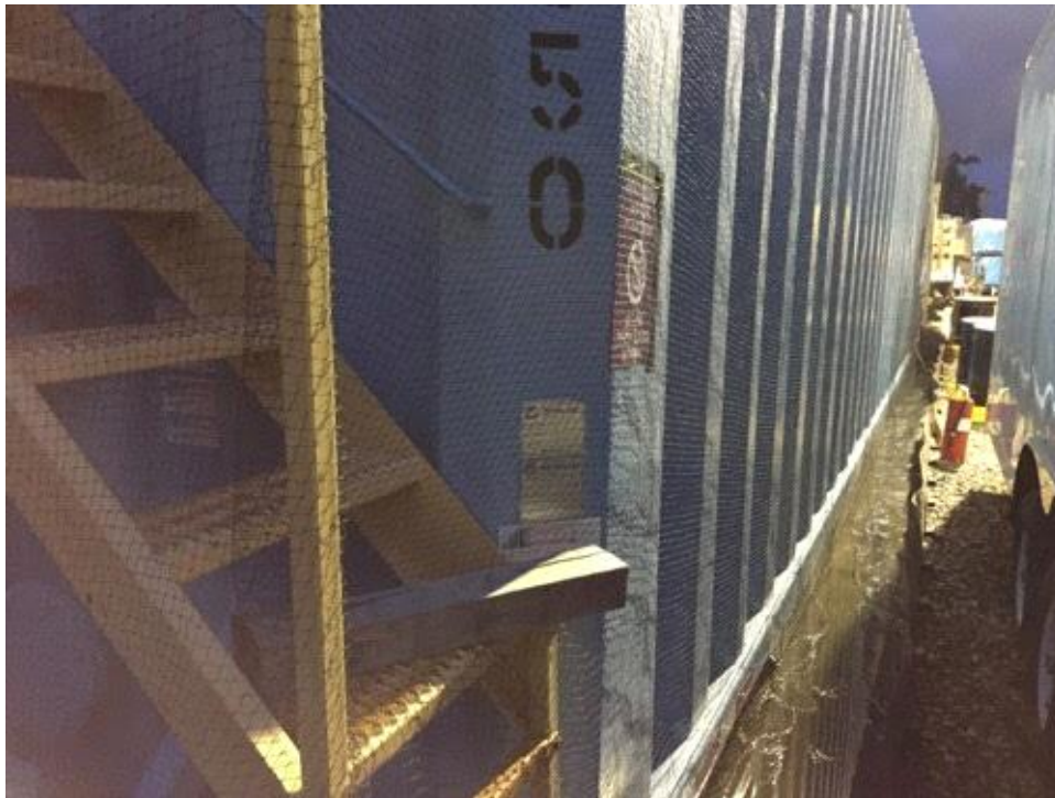
Caption Bird netting in place to discourage nest building on stationary equipment.
