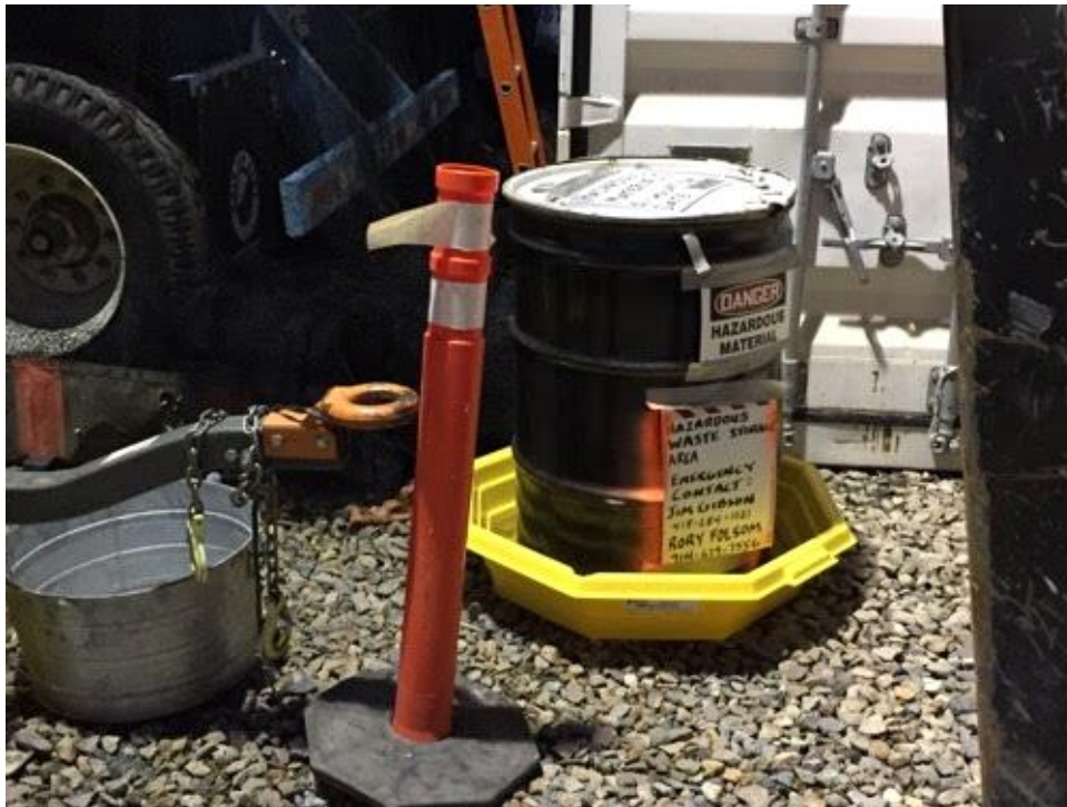
Caption Hazardous materials clearly marked and stored in secondary containment.
