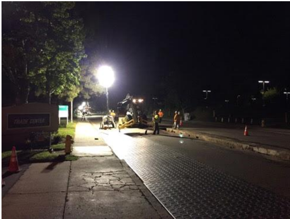
Caption Removing steel plates to continue with underground work.
