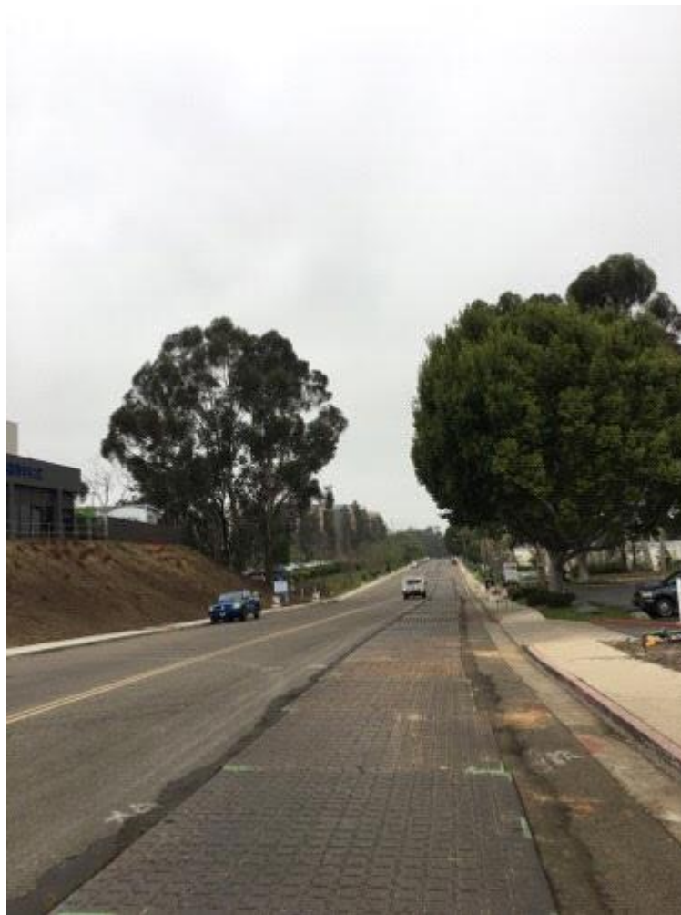
Caption Trade Street trench plates.
