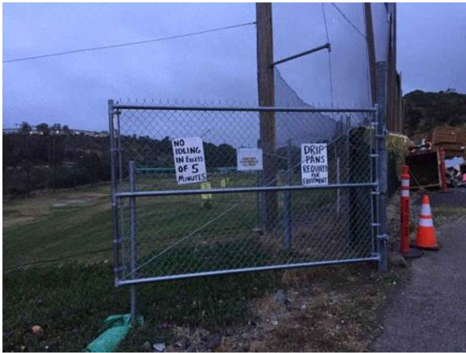
Caption Requirement reminders posted at entrance to storage yard.
