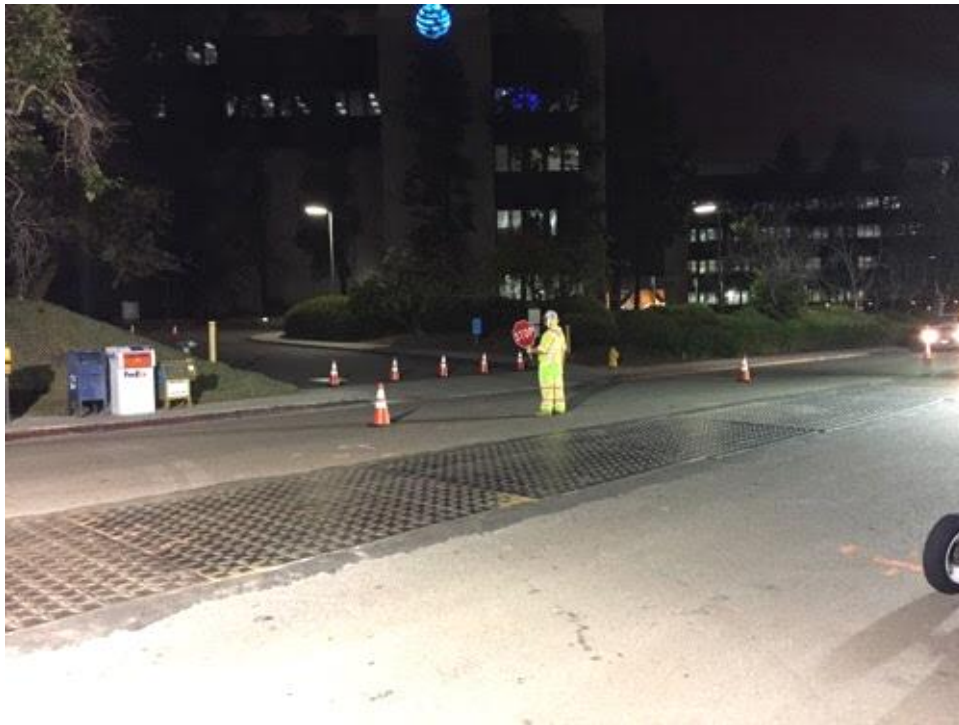
Caption Traffic flaggers in place.
