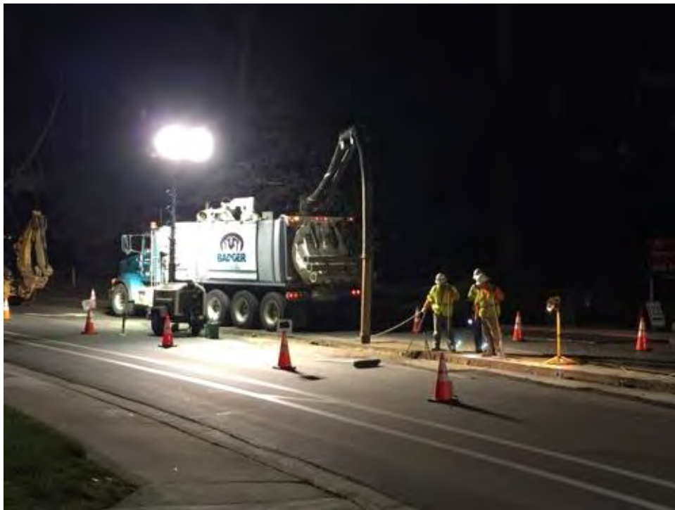
Caption Potholing in progress.
