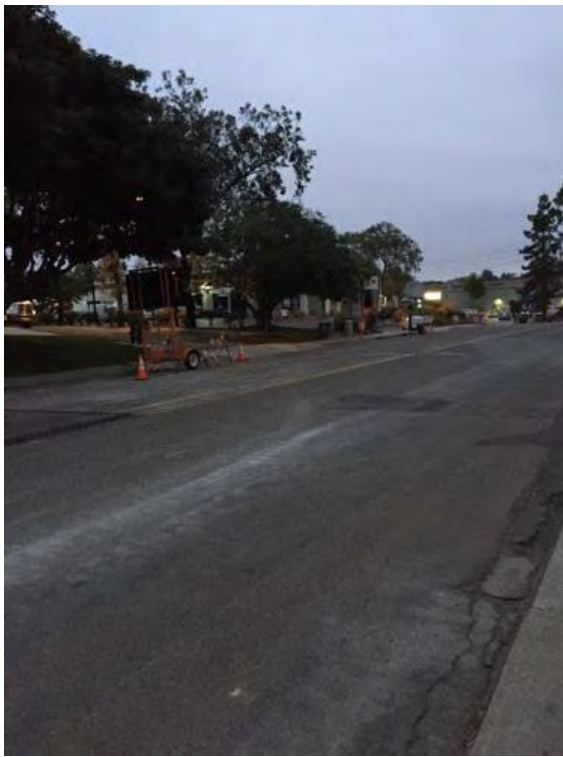
Caption Constrction removed from street by 5:00 A.M.
