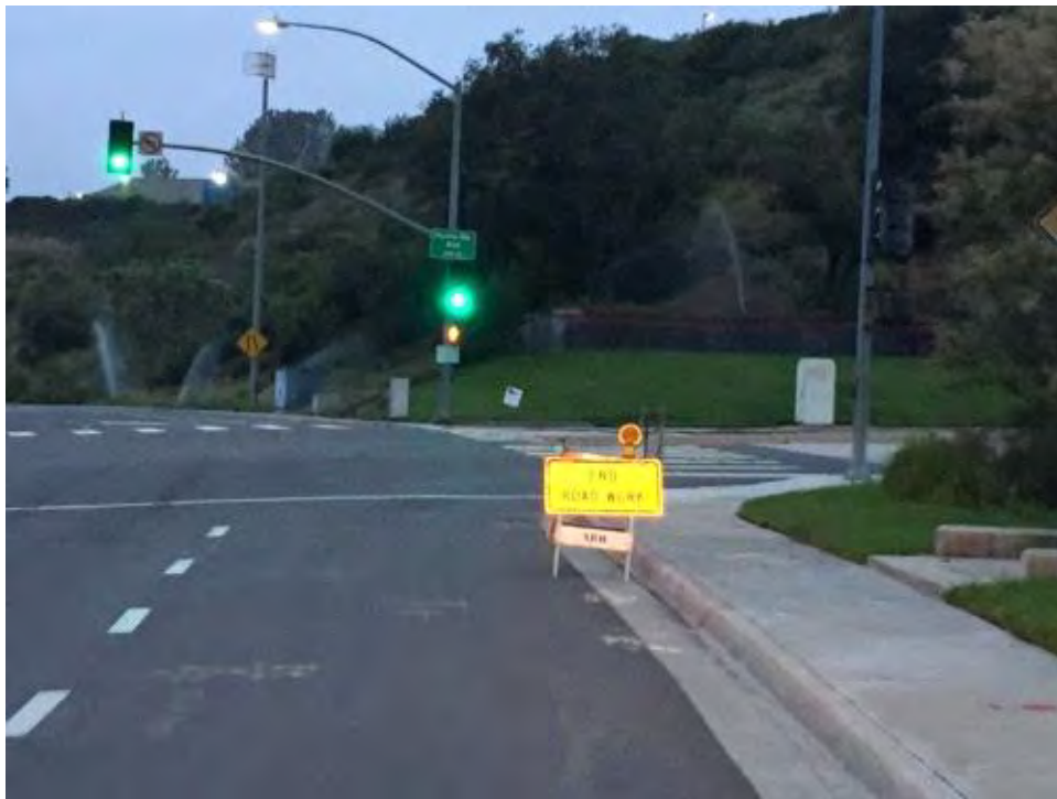
End of construction area clearly marked.
