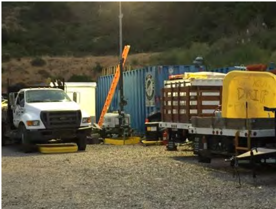
Caption Drip pans for secondary containment in place.
