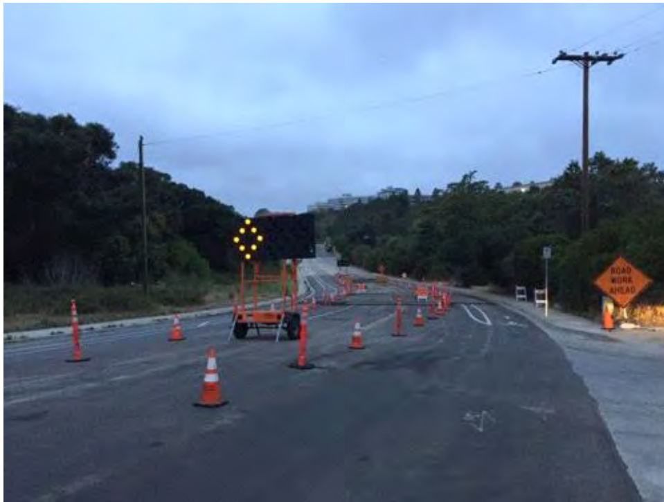
Caption Traffic signage and cones in place.
