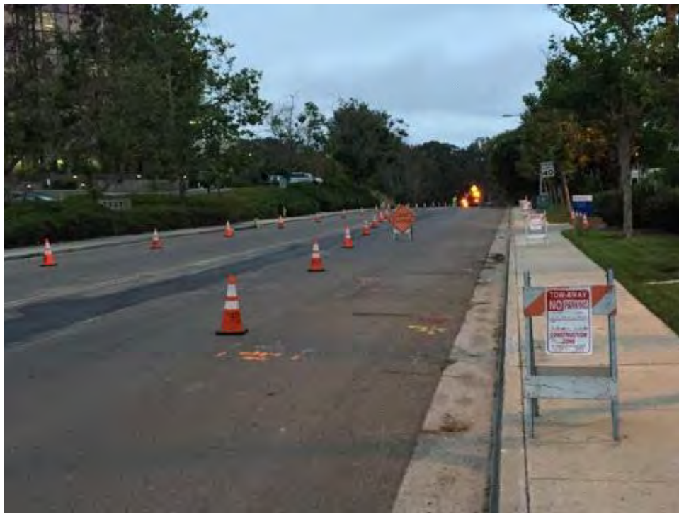
Caption Traffic cones and signage in place.
