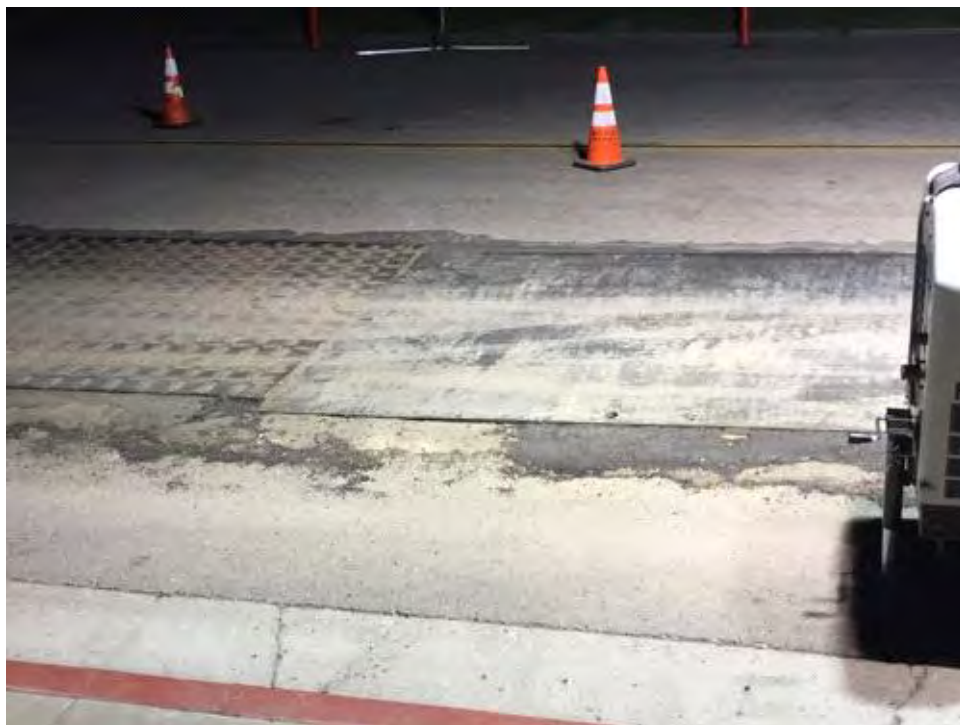
Caption Steel plates covering trenches.
