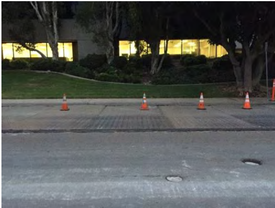
Steel plates covering vault at end of construction.
