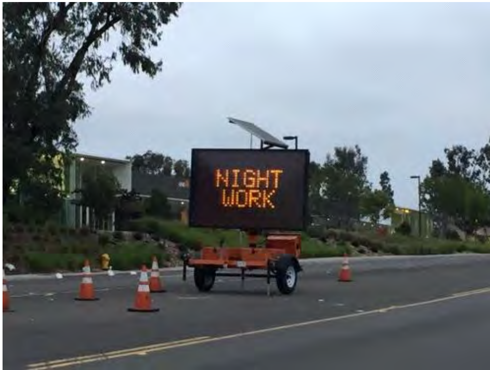
Caption Digital traffic signage in place.
