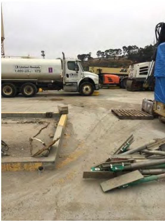
Caption Vulcan Staging Yard.
