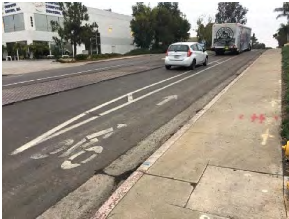
Carroll Rd. work site with asphalt rock debris.
