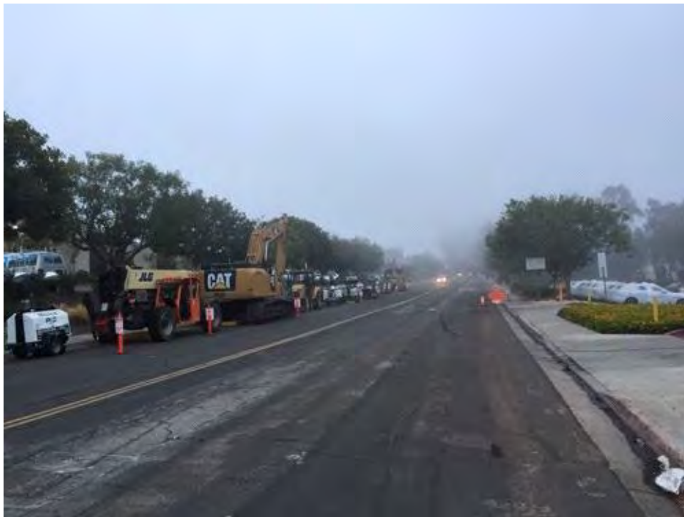
Caption Equipment safely stored and returned to unrestricted public access.
