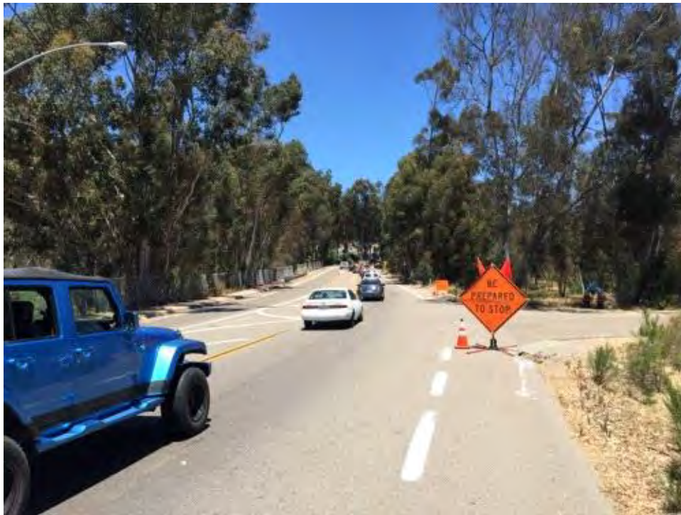
Caption Signage and cones in place at entrance of Pomerado Road.
