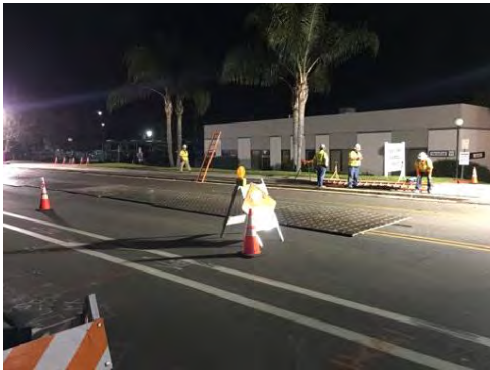
Caption Steel plates covering trenches on upper Carroll Canyon Road.
