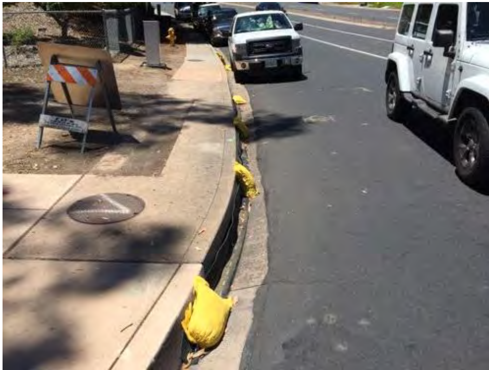
Caption BMPs in place on Willow Creek Road.
