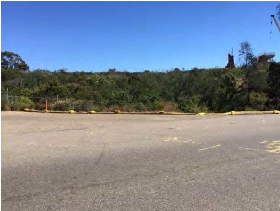
Caption Wattles in place on Pomerado Road.
