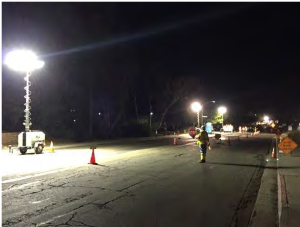
Caption Abundant lighting in place on Trade Place.
