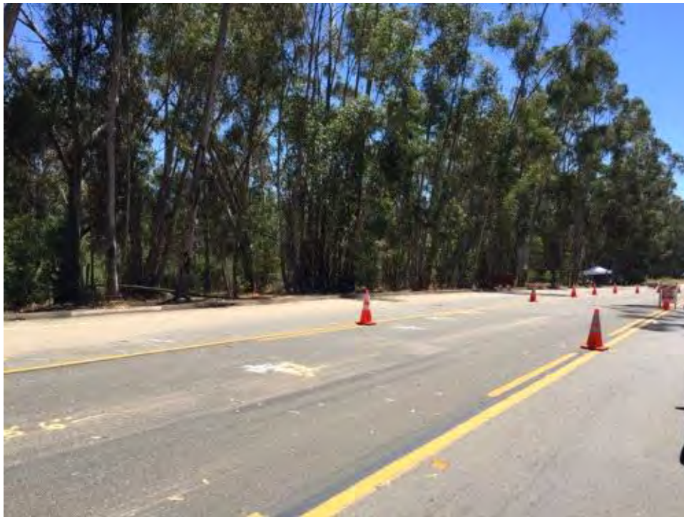
Caption Cones and markers in place on Pomerado Road
