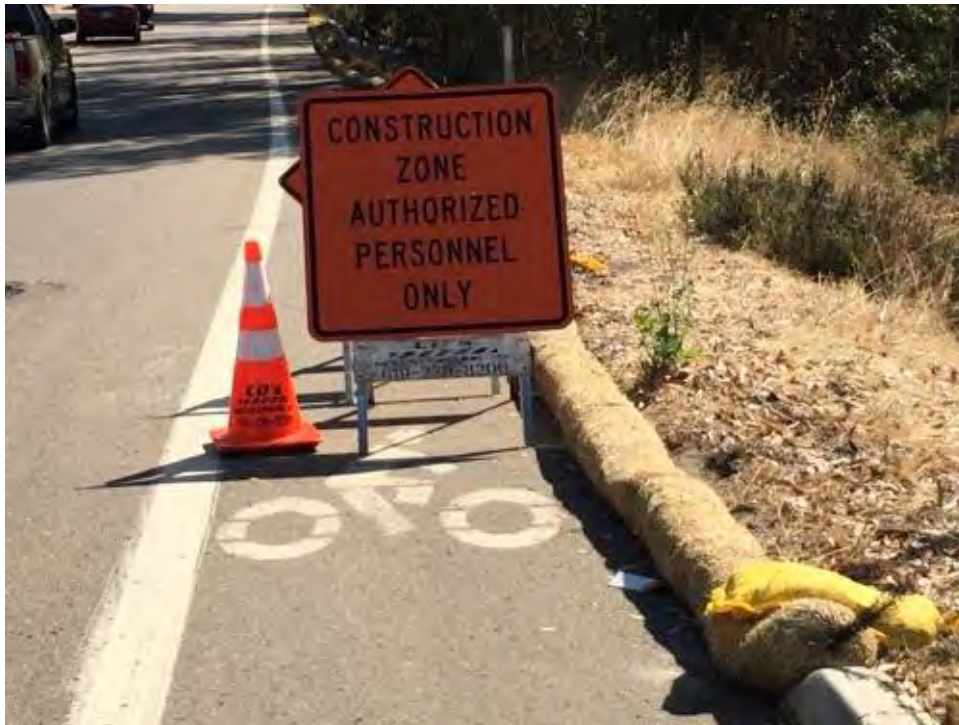
Caption BMPs in place on Pomerado Road
