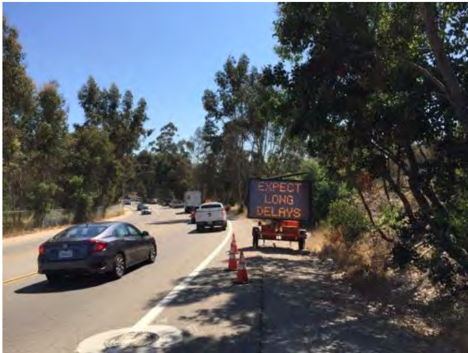
Caption Digital signage in place. Pomerado Road beginning of construction zone.
