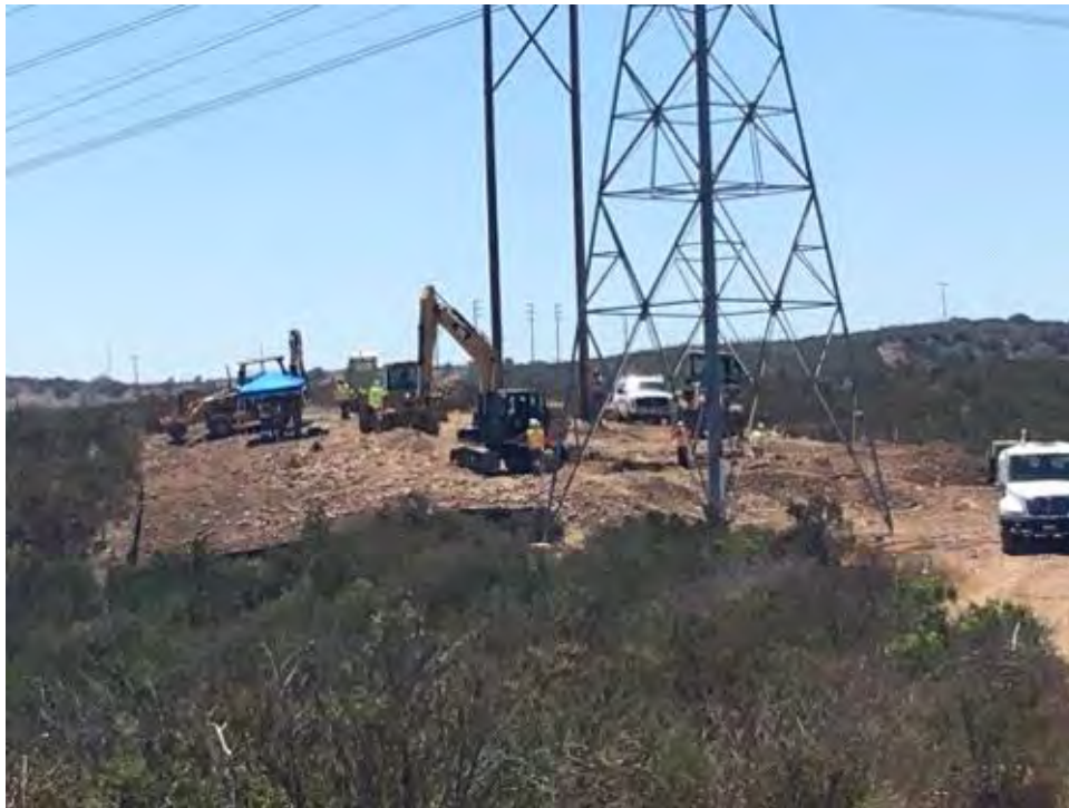
Caption P04 overview of grading
