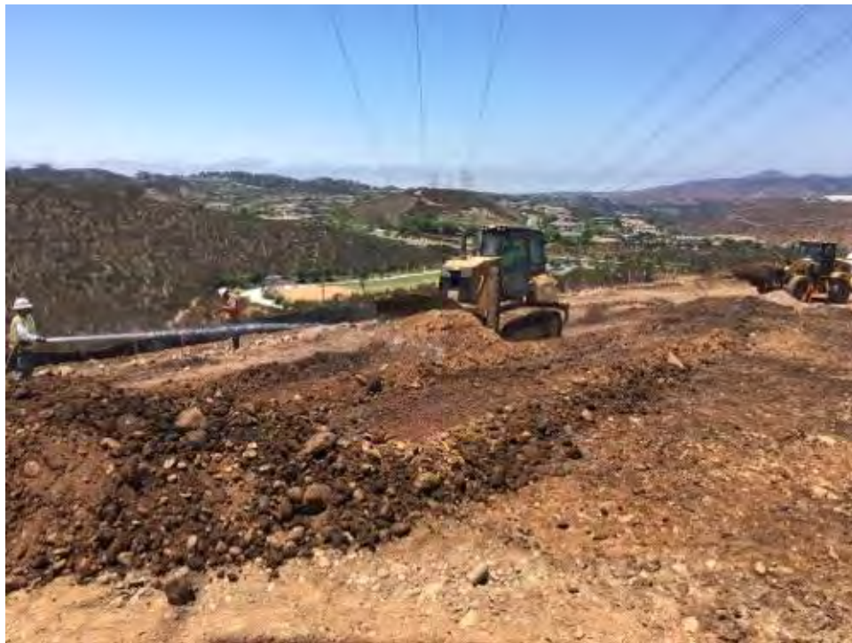
Caption P04 work site.
