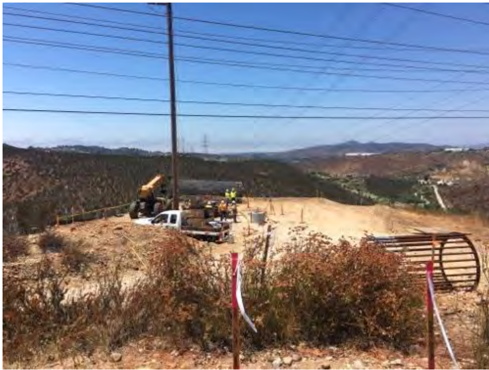
Caption P03 work site.
