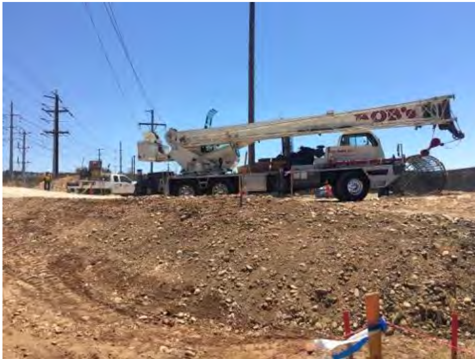
Caption Crane at P0.3
