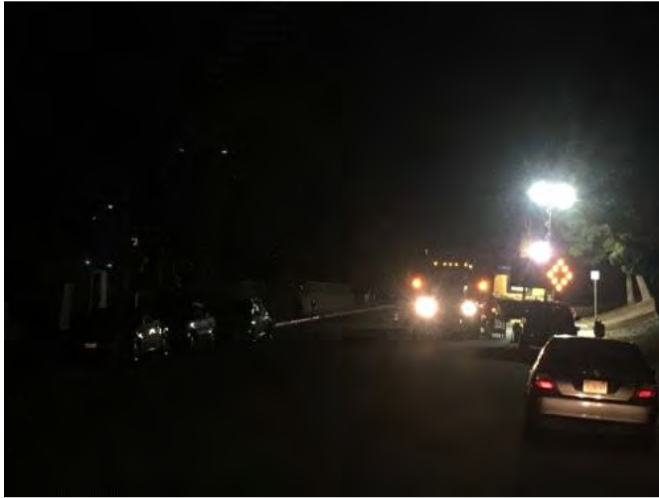
Caption Equipment staging area on Clayton Drive. Photo Attributes Capture Date/Time: Wed Jul 26 2017 23:13:43 GMT-0700 (PDT) Coordinates: 32.895044, -117.130942 View Direction: North
