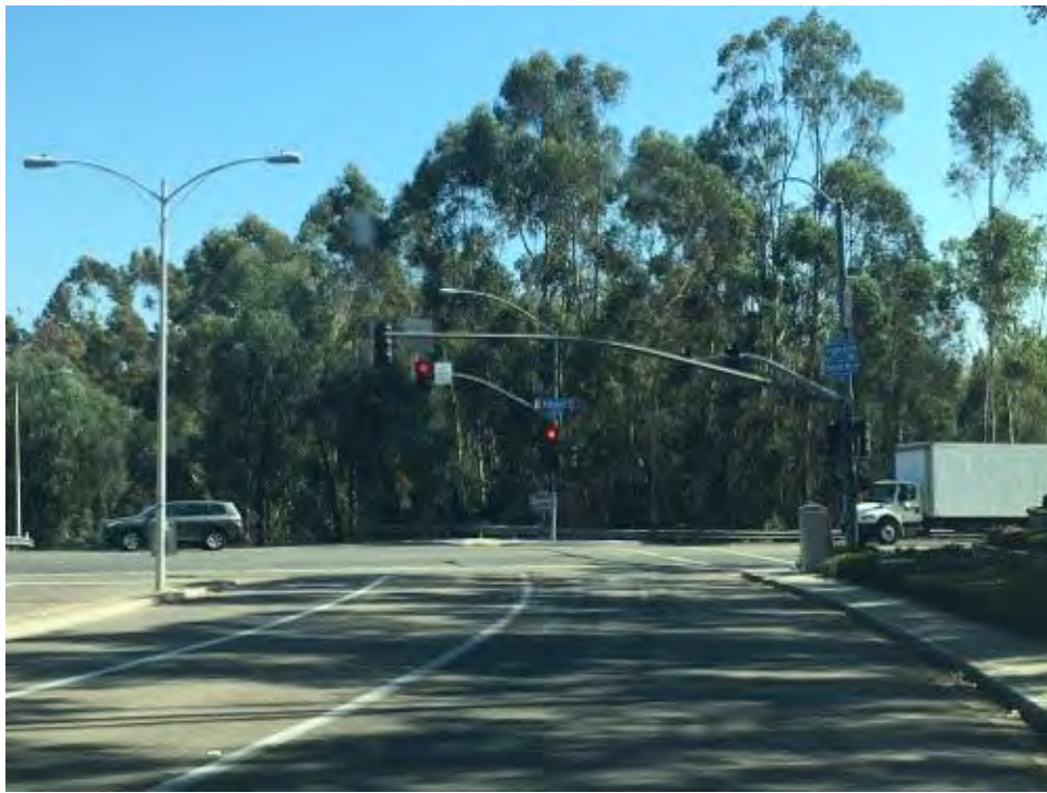
Caption Pomerado Road and Scripps Ranch Blvd. following construction.
