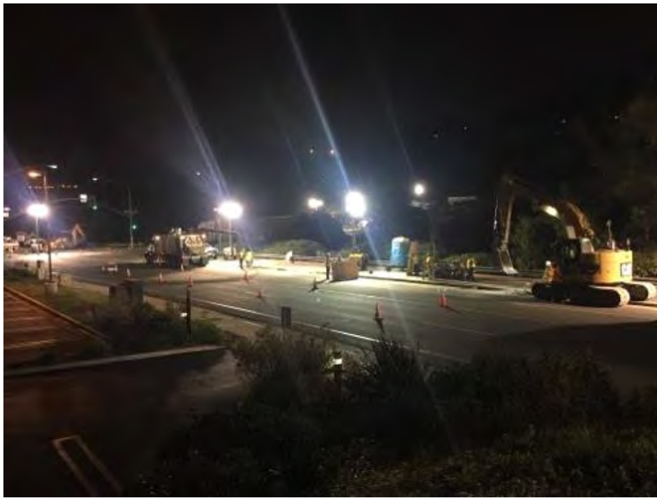
Caption Trenching/excavation on Carroll Road east of Nancy Ridge Drive.
