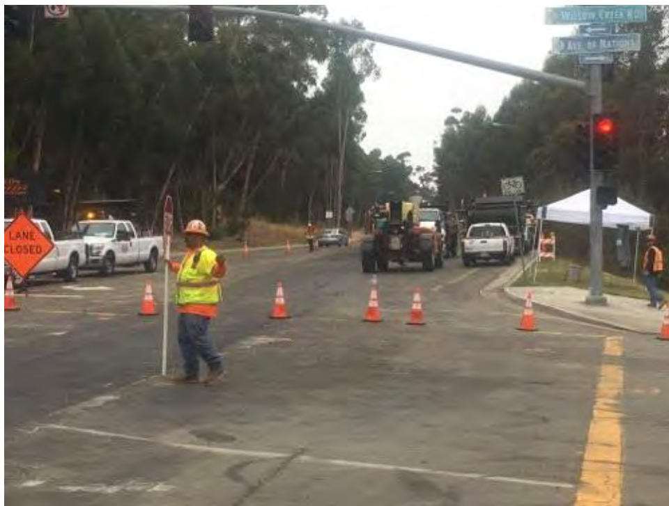
Caption Pomerado Road work site east of Avenue of Nations.
