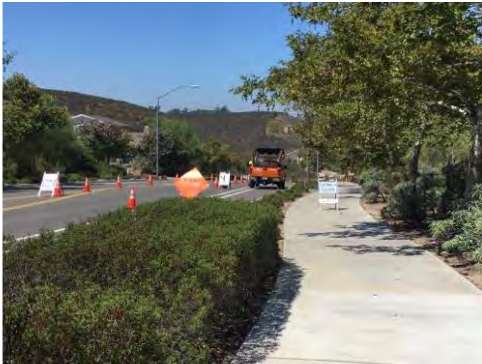
Caption Traffic control on Stonebridge Parkway near P05.
