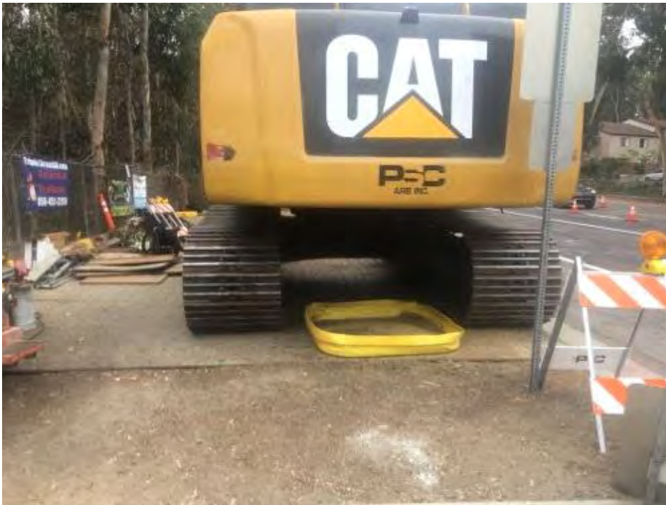
Caption Drip pan beneath excVator.
