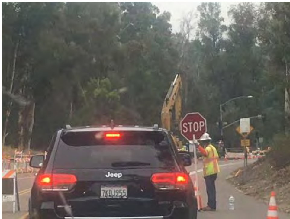
Caption Traffic control east of Fairbrook Road, vault work site active.
