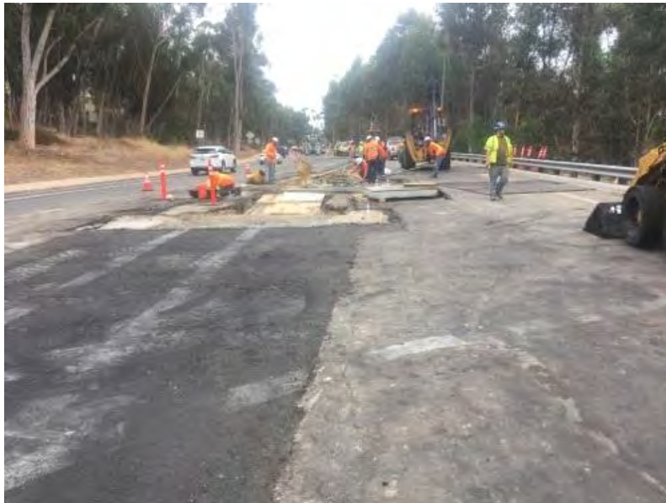
Caption Trench work
