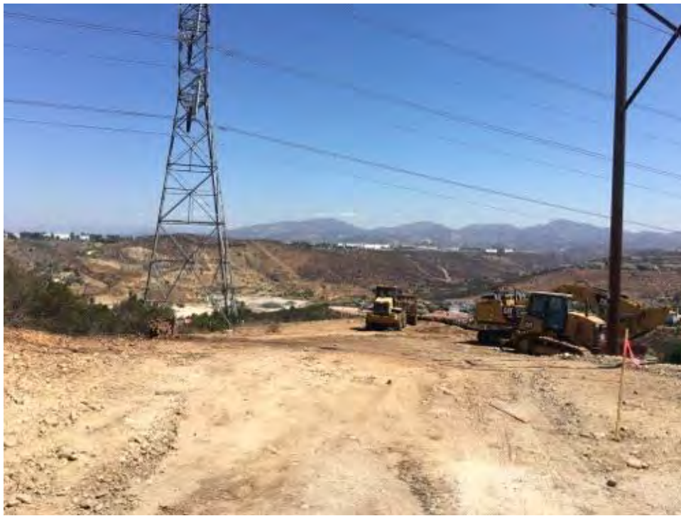
Caption P05 being used to stage equipment.
