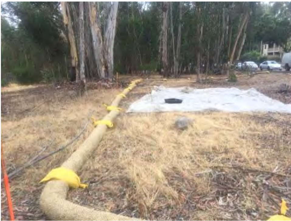
Caption MPR #5 storage area not currently in use.
