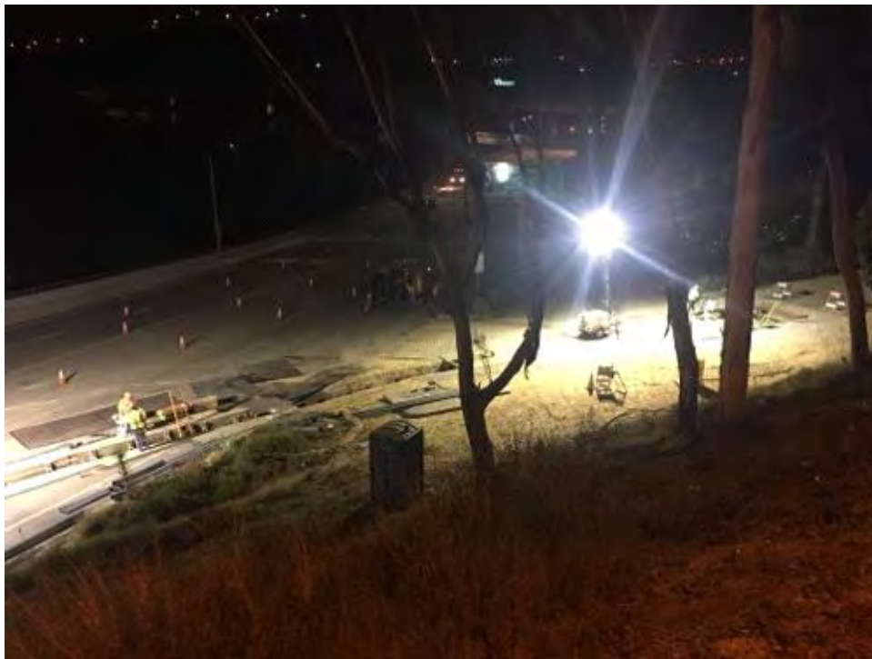
Caption Trench near CCM MCP entrance.
