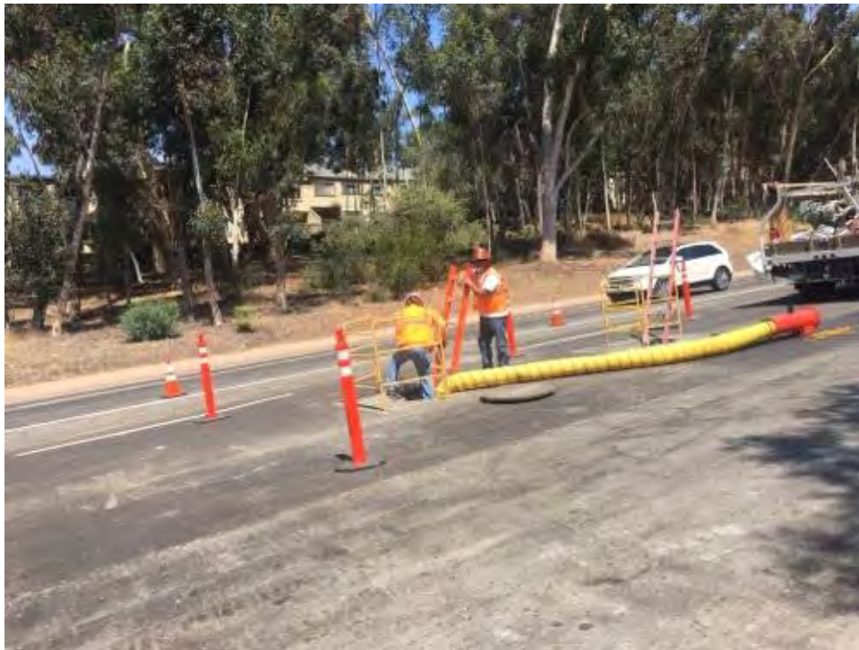
Caption Vault work on Pomerado Road.
