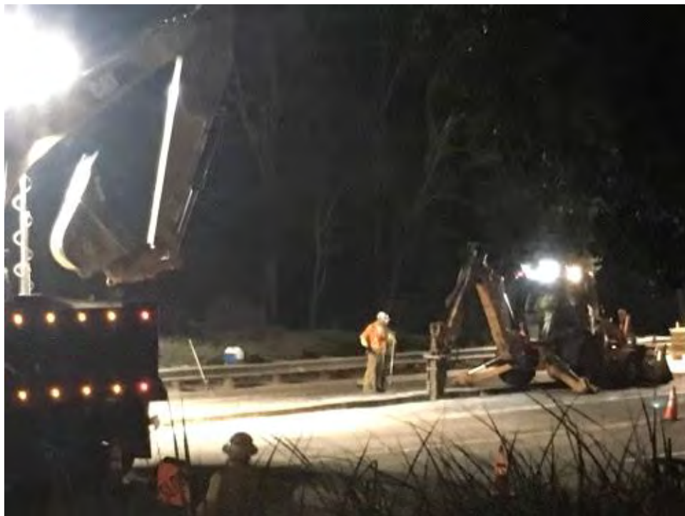
Caption Excavation on Carroll Road.
