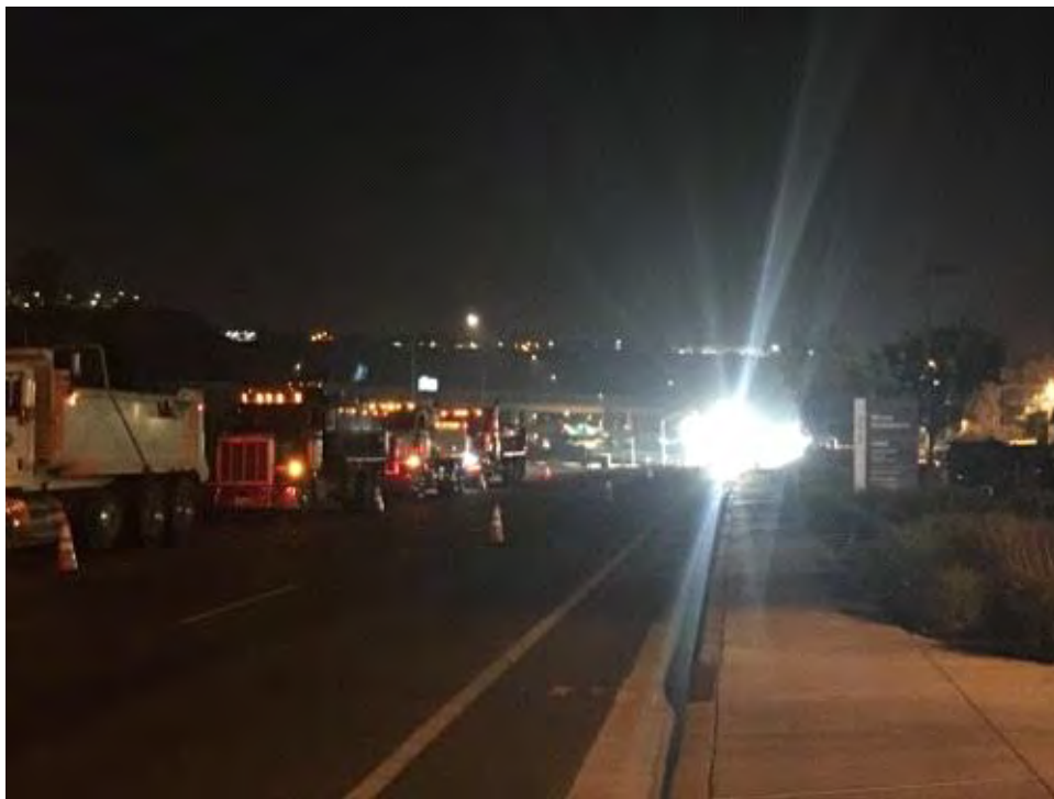
Caption Truck line waiting for fill material.
