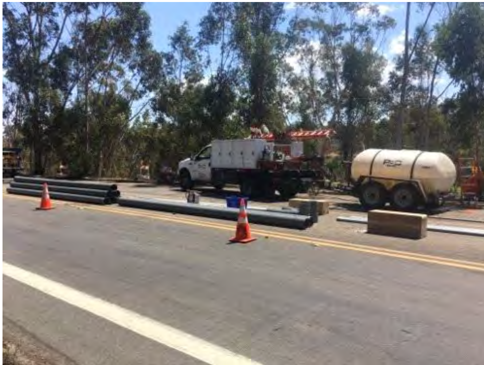
Caption Fire equipment on site on Pomerado Road.
