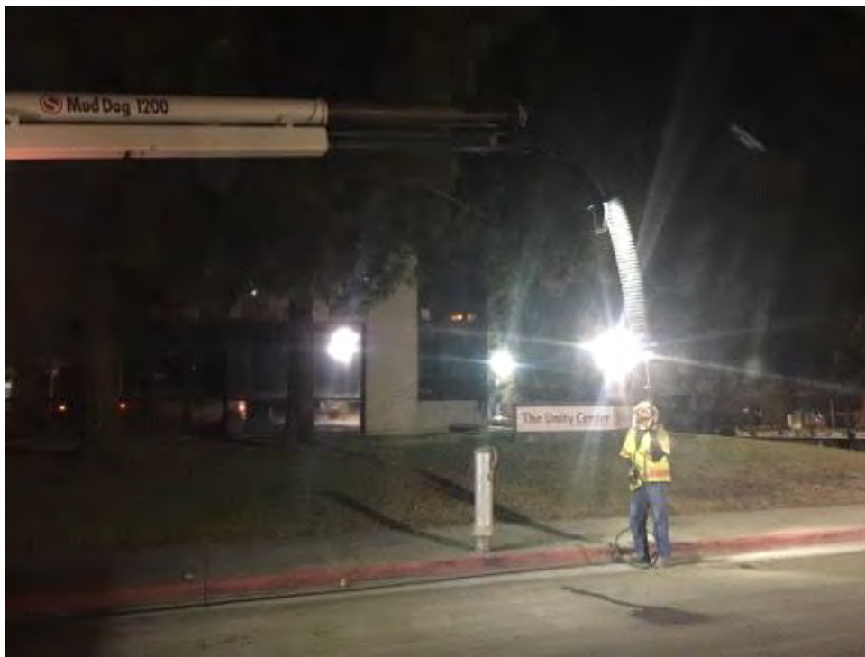
Caption Potholing near activity.
