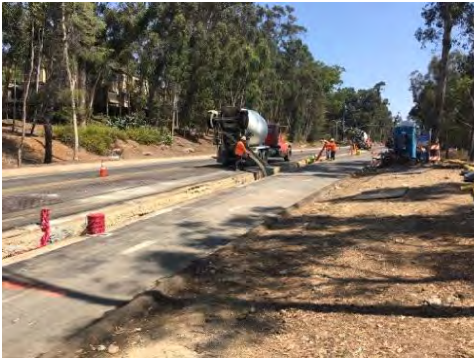
Caption Concrete work on Pomerado Road.
