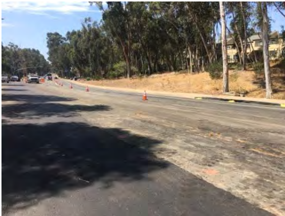
Caption Traffic lane looking at Ave of Nations.
