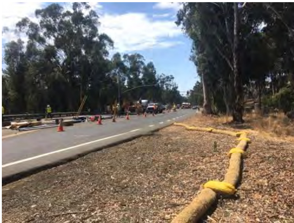
Caption Pomerado Road just east of Scripps Ranch Blvd., notice BMPs.
