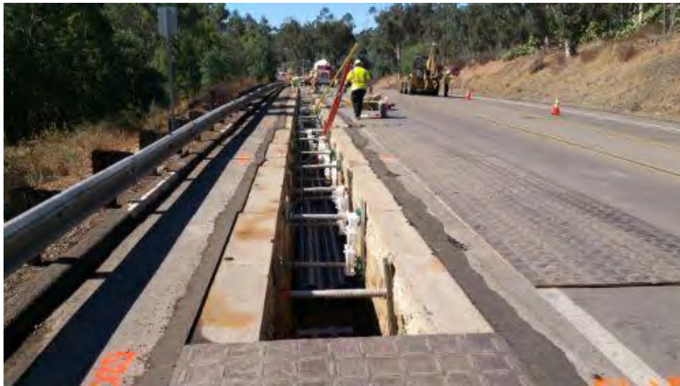
Caption Laying conduit along Pomerado Road.
