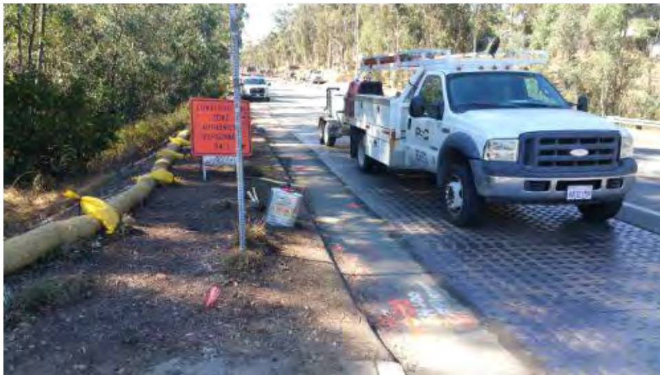
Caption Fire tools accessible, Pomerado Road at Avenida Magnifia.
