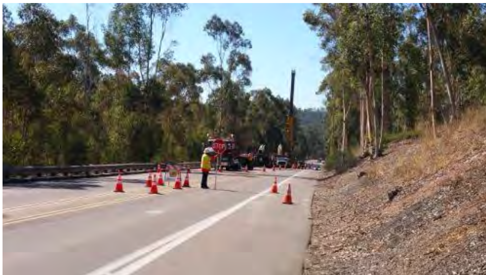
Caption Traffic control, east end of Pomerado Road work area.
