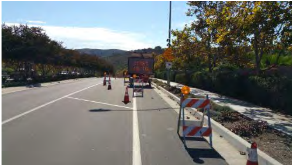
Caption Traffic control, west end of Stonebridge Pkwy.
