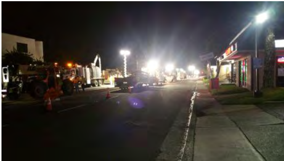
Caption Overview of work area on Black Mtn. Road.
