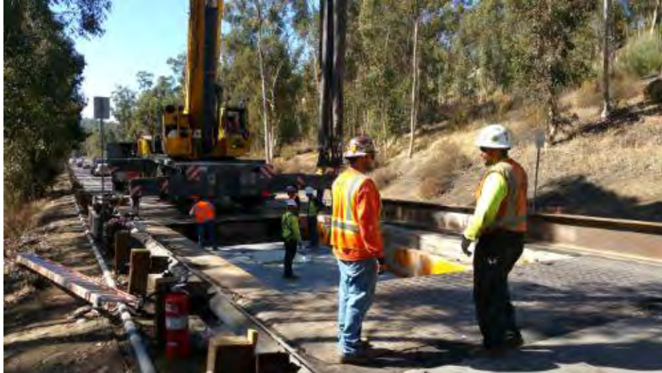
Caption Vault placement, Pomerado Rd.
