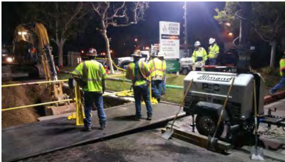
Caption Monitors present at vault work on Activity Road.
