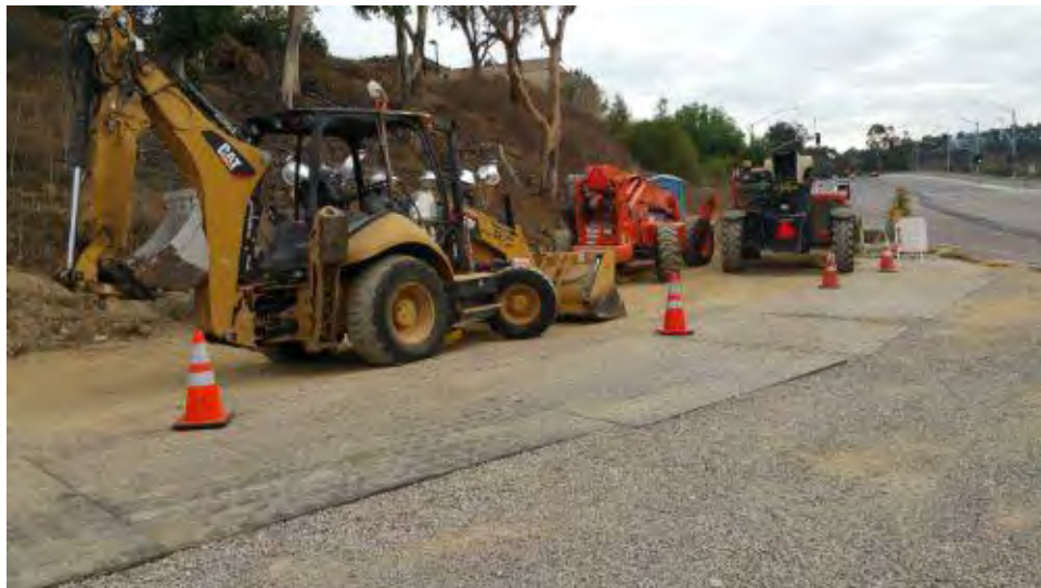
Caption Equipment storage area on Carroll Canyon Road and I-805.
