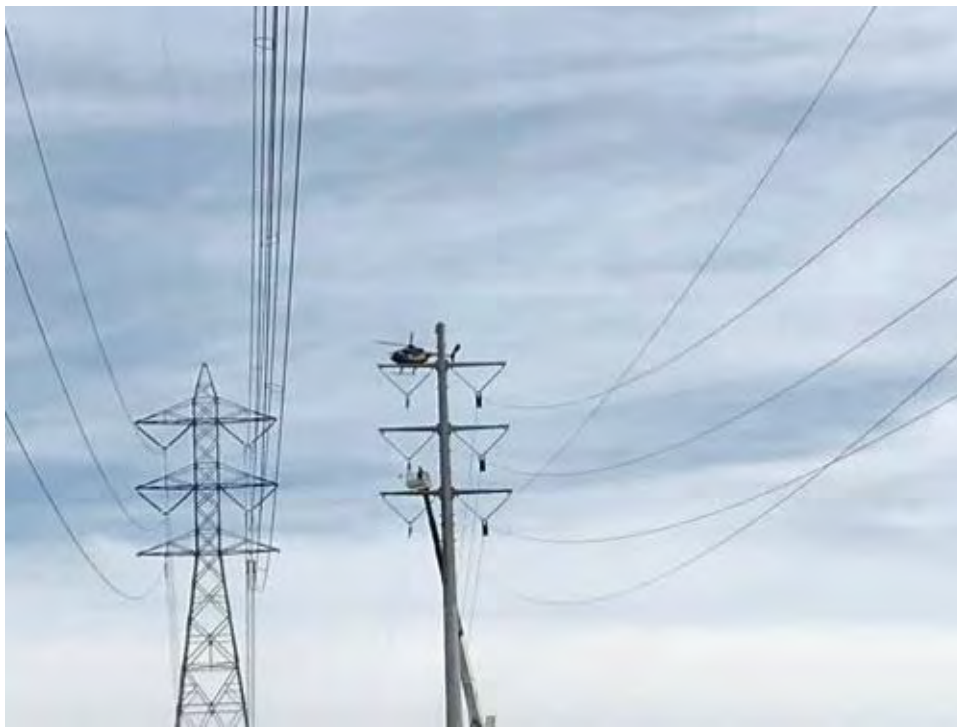
Helicopter pulling sock line to P04.
