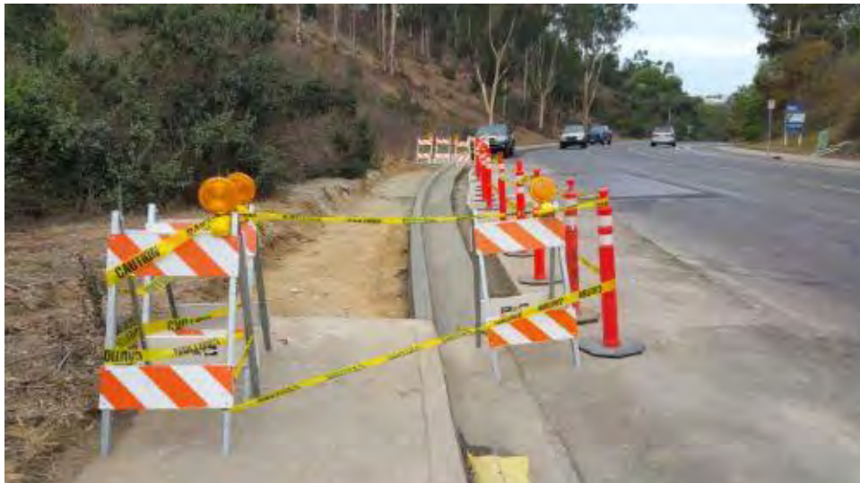
Caption Curb replacement site (night work) on Carroll Canyon Road.
