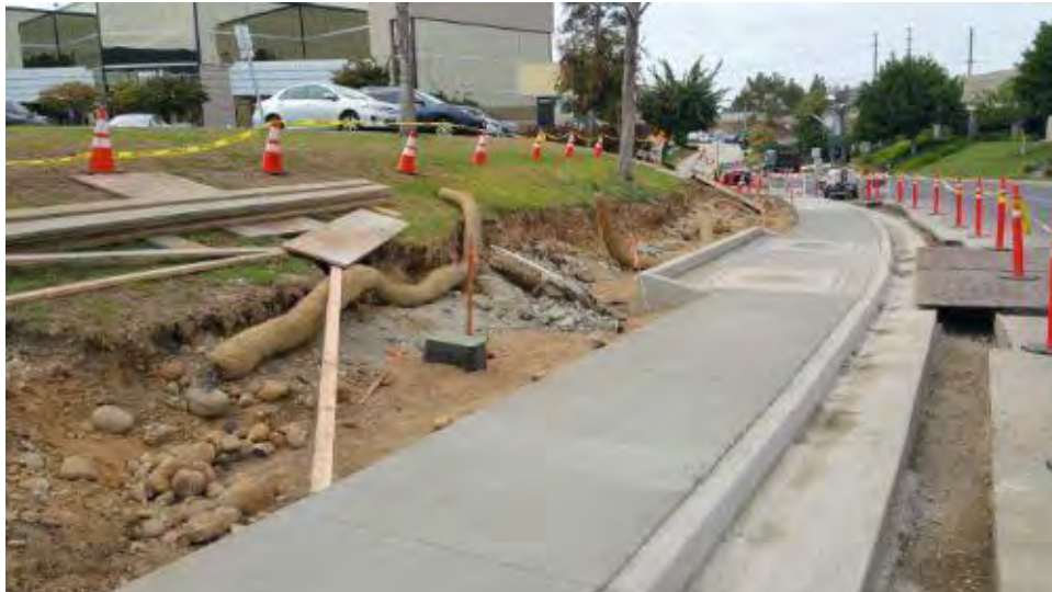
Caption Sidewalk replacement on Activity Rd. Fiber rolls would not work for erosion control; poor site maintenance.
