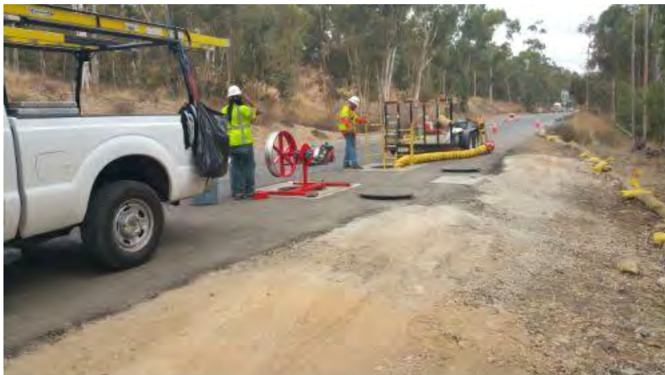
Caption Crew cleaning underground line on Pomerado Road.
