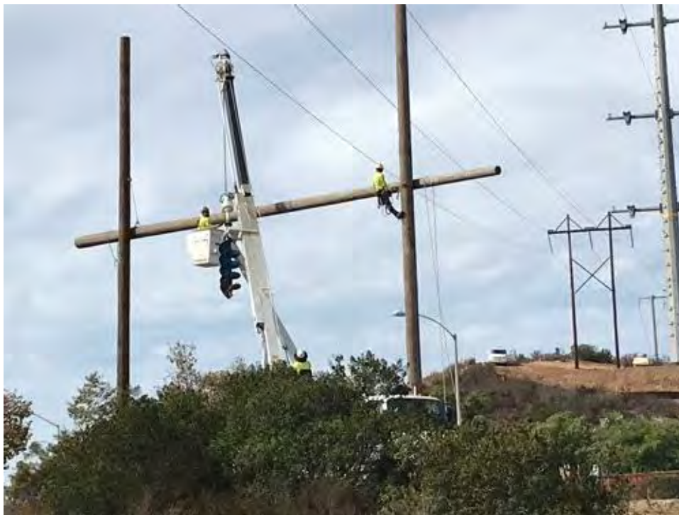
Adjusting guard structure off Stonebridge Parkway.
