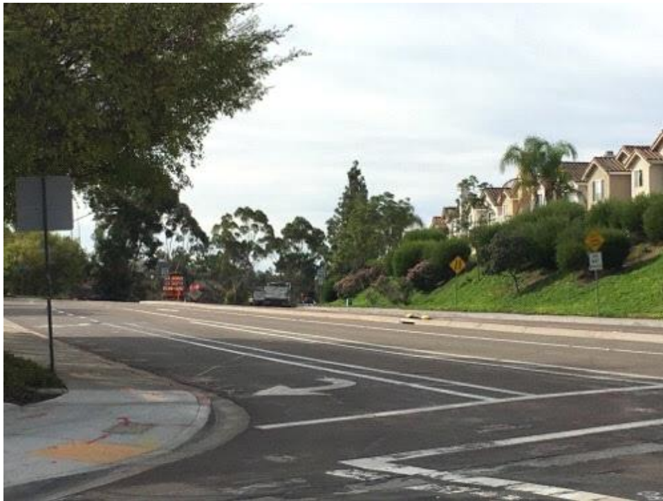
Eastern edge of work/traffic control before intersection at Spring Hill Road.
