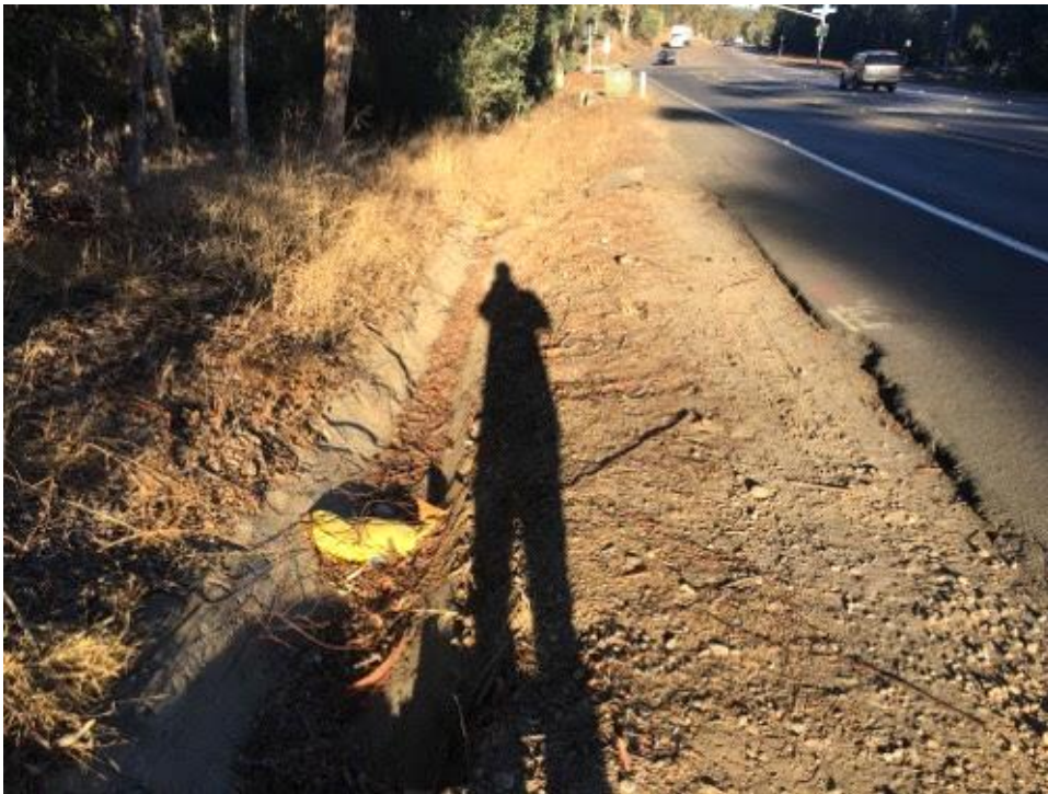
Caption Leaf litter in drain, City has requested these areas be maintained.
