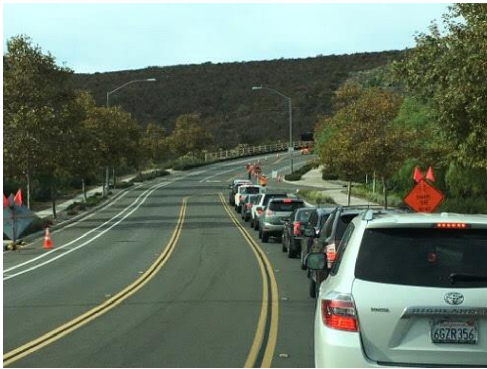
Caption Traffic control on Stonebridge Parkway.
