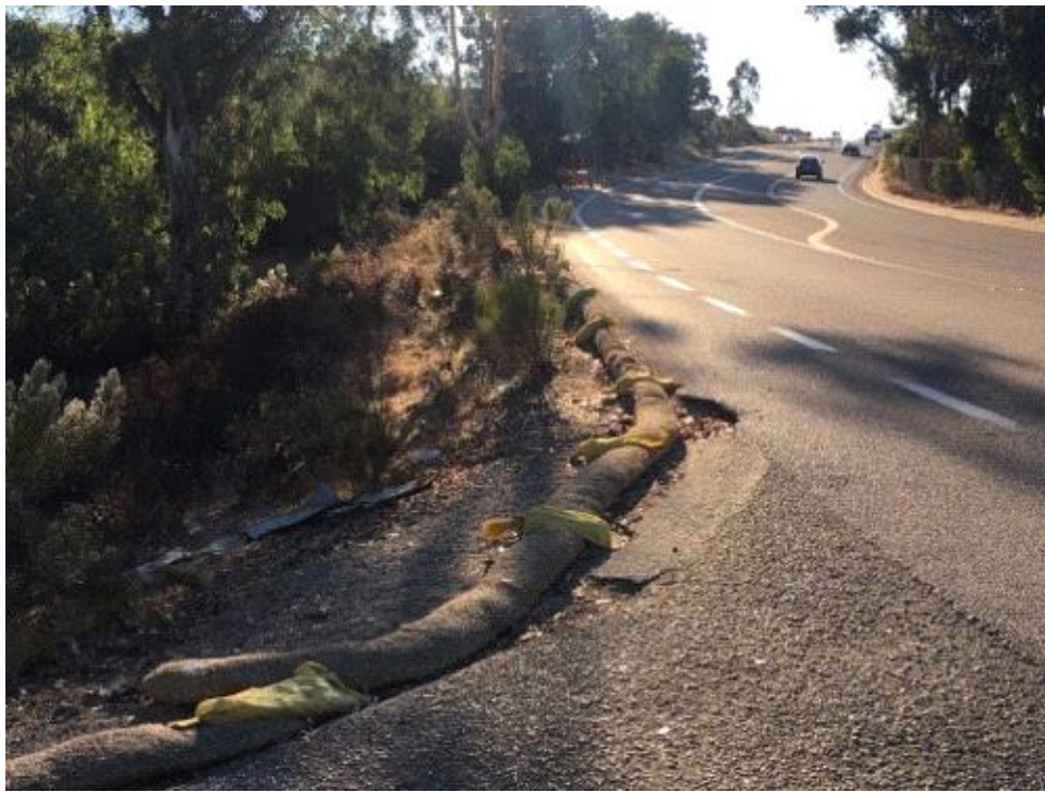
Caption Fiber Roll acting as curb, not staked but no soil disturbance south of the road.
