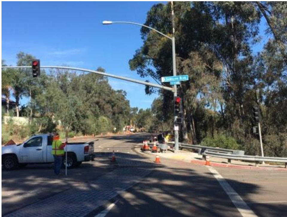
Caption Work on Pomerado Road at intersection with Semillon Blvd.
