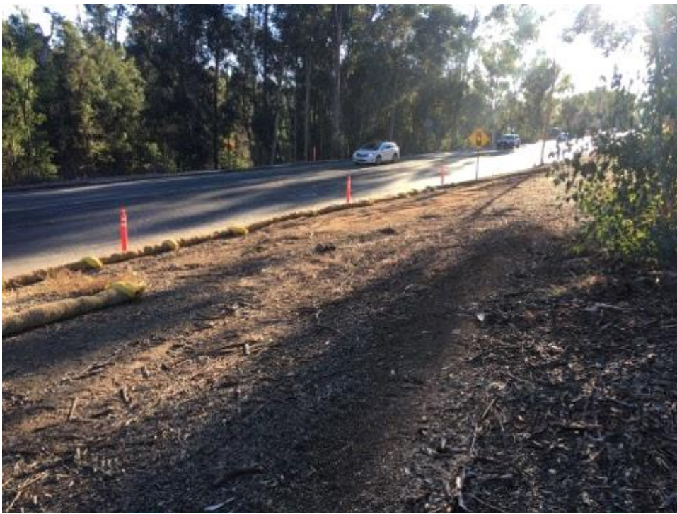
Caption Area still needs to be trenched and staked.
