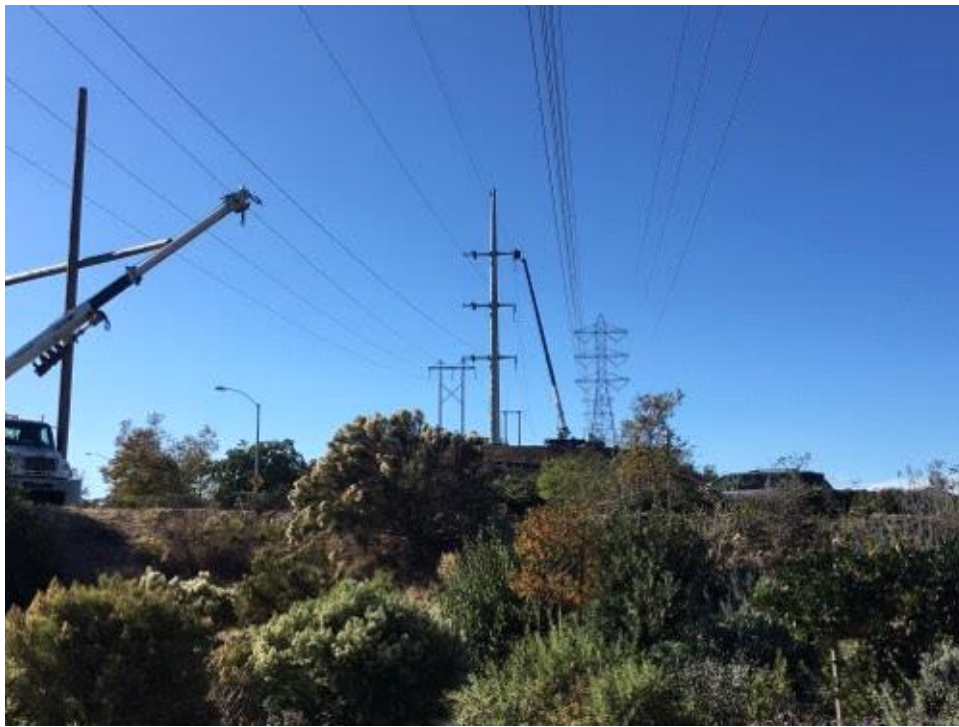
Caption Overhead wire work at P05.
