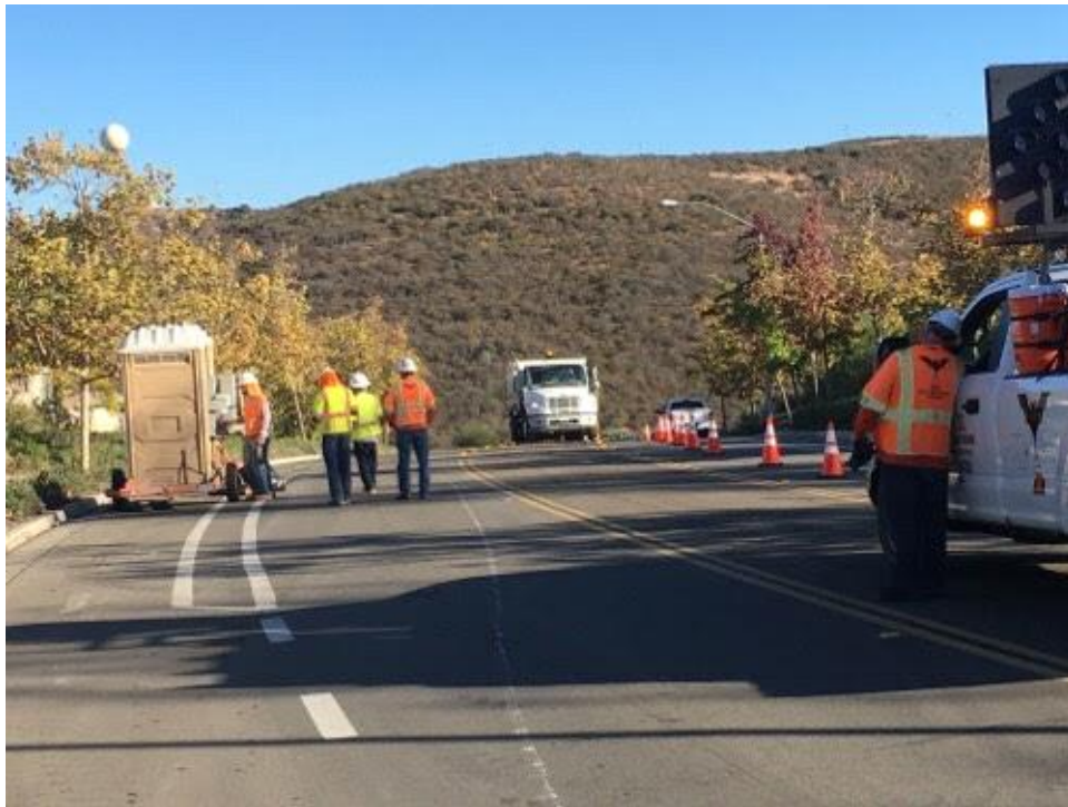
Caption Street sweeper cleaning Stonebridge Parkway work site.
