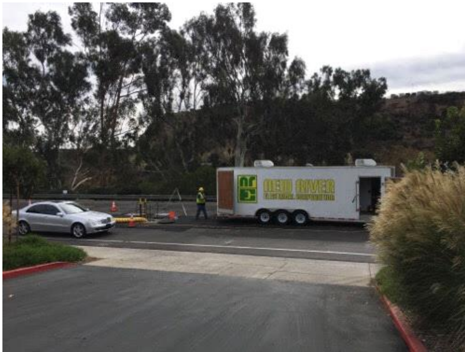
Cable/vault work on Carroll Canyon Road.
