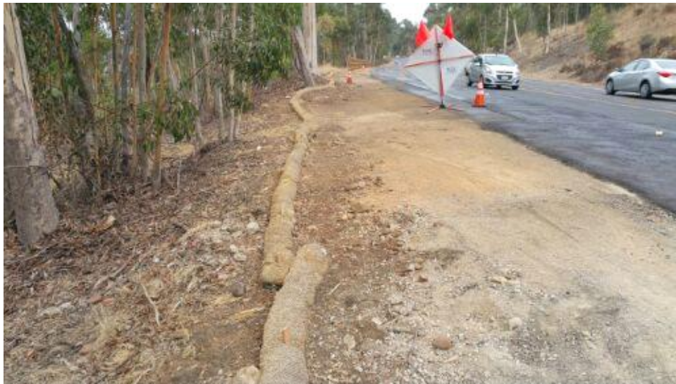
Caption Fiber roll installation on Pomerado Road.
