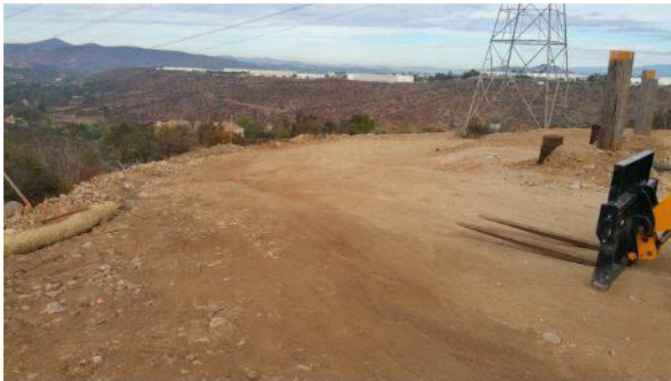
Caption Erosion control BMPs at PO6 site: fiber rolls and gravel berm.
