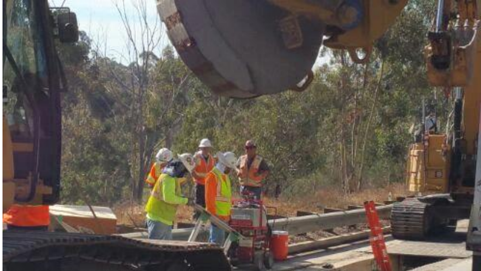
Caption Trenching on Pomerado Road. Three resource monitors observing work.
