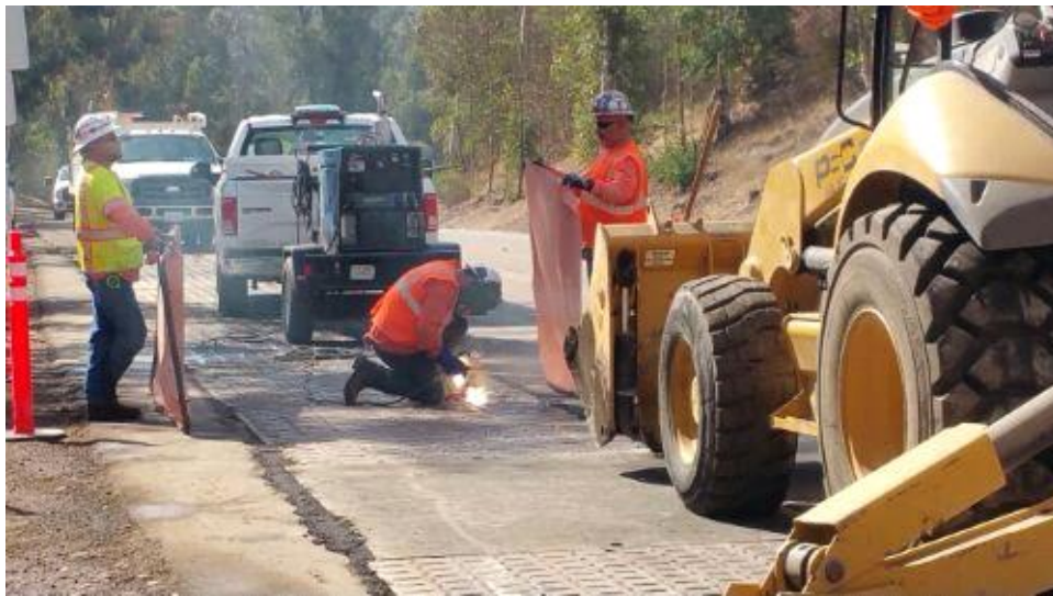
Caption Fire protection in place during trench cutting on Pomerado Road.
