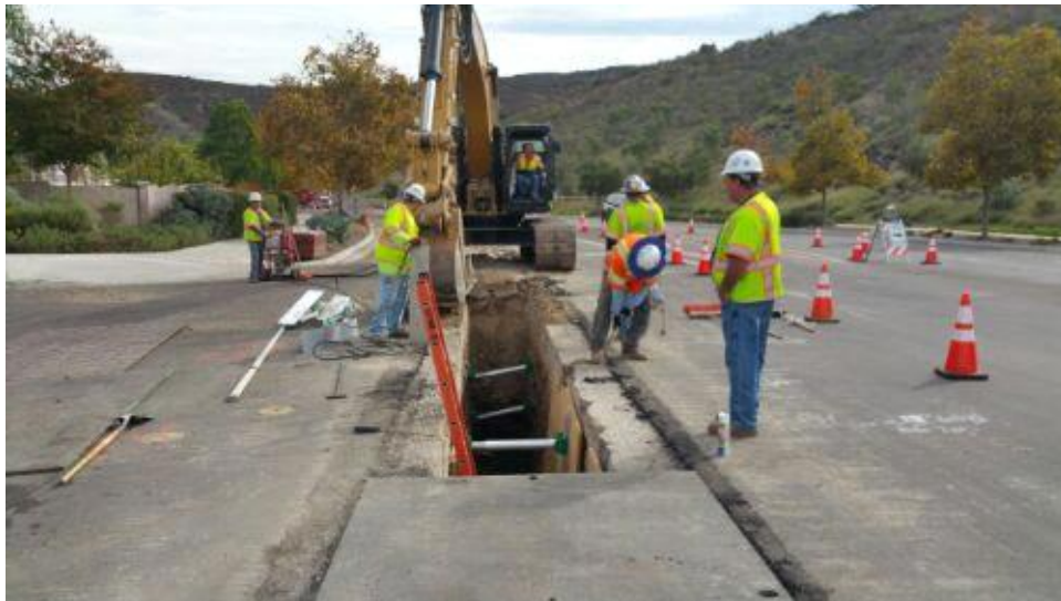
Caption Excavation on Stonebridge Parkway, monitors present.
