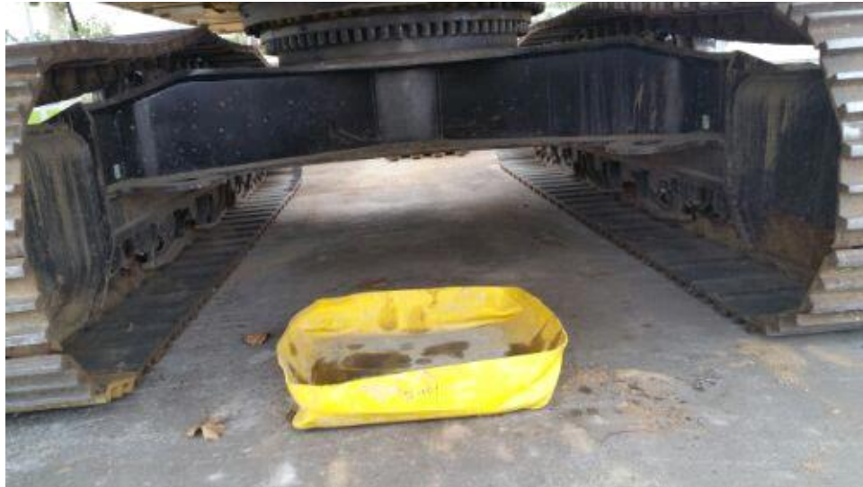
Caption Properly placed drip pan at Padgett Street 'staging area.
