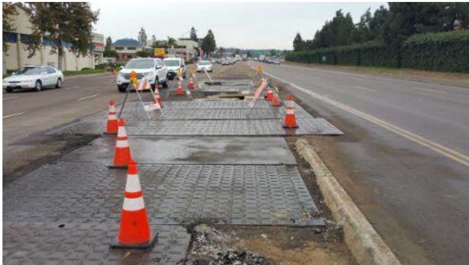
Caption Well-marked work zone on Miramar Road.
