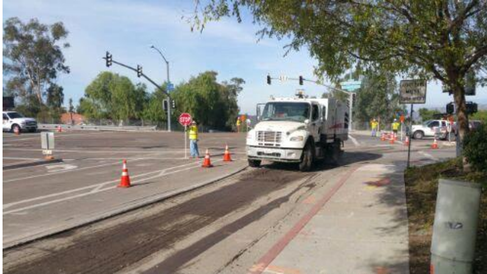
Caption Street sweeping and five flaggers at Pomerado Road corner.
