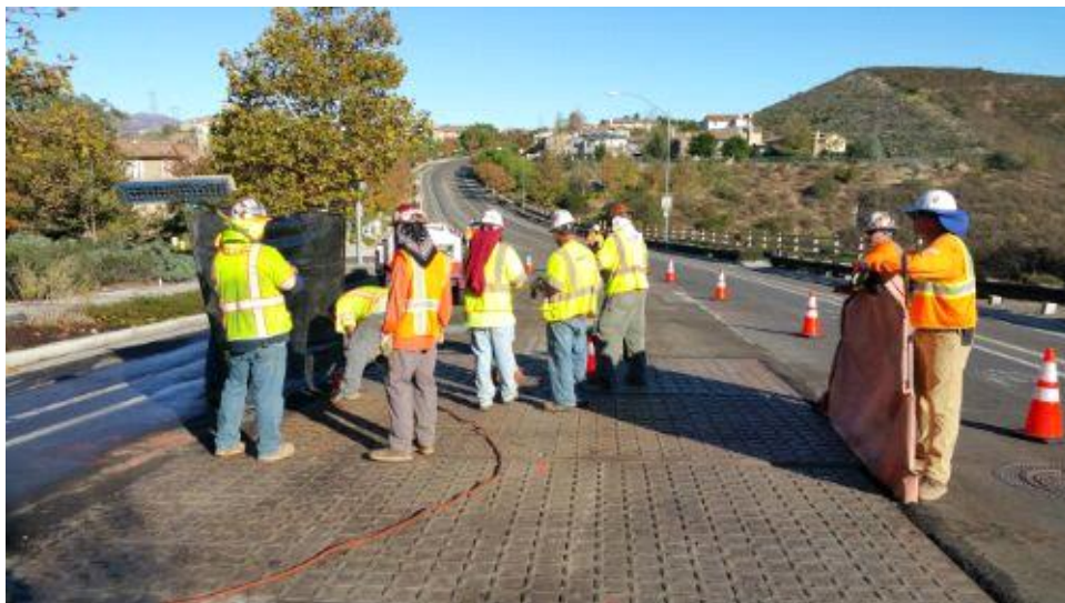
Caption Welding trench plates with excellent fire protection on Stonebridge Parkway.
