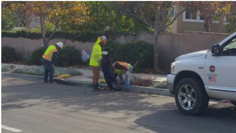
Caption Crew maintaining sediment traps on Stonebridge Parkway.
