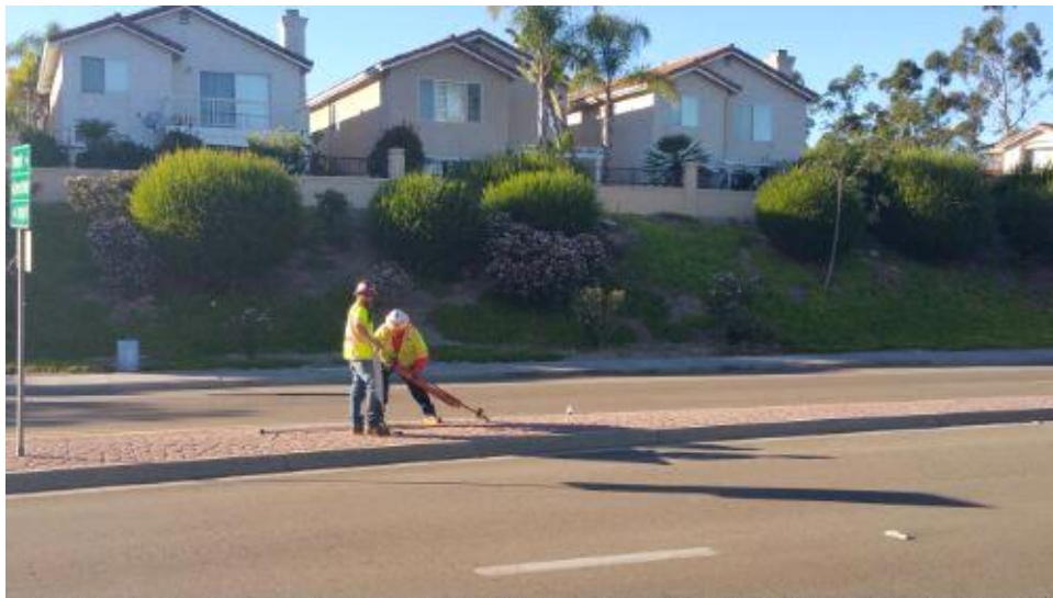
Caption Taking down traffic control signs on upper Pomerado Road.
