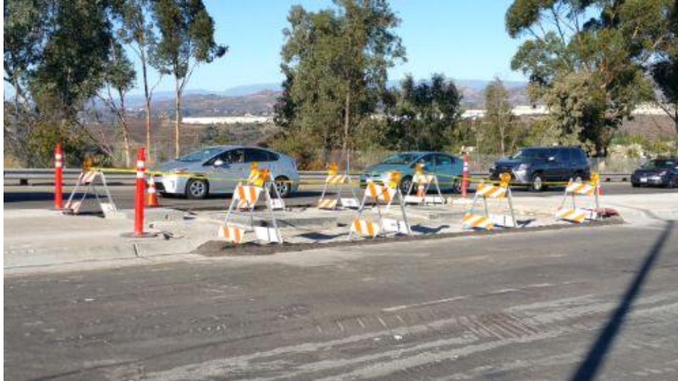
Caption Barrier around vault on Pomerado Road.
