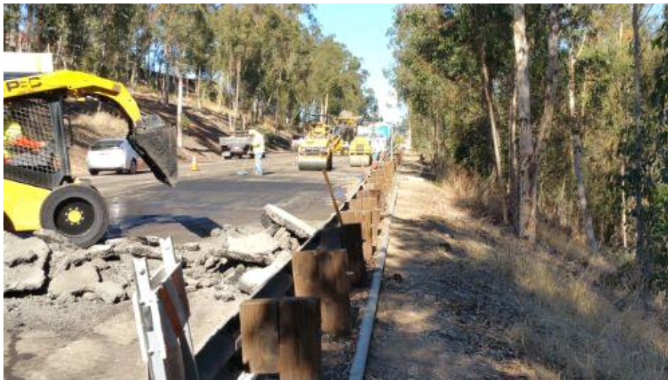
Caption Asphalt removal on Pomerado Road.
