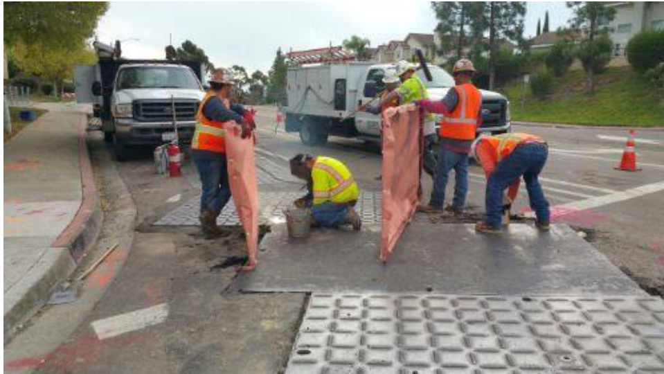
Caption Welding trench plates shut on Pomerado Road.
