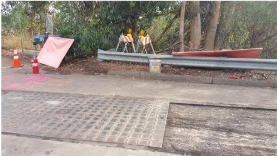
Caption Fire protection equipment, Pomerado Road at Sycamore Test.
