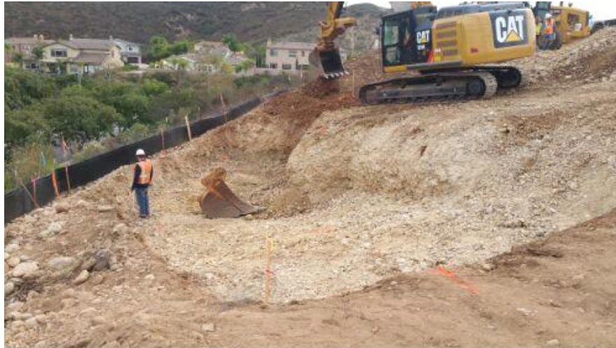
Caption Excavation at PO5 for retaining wall.
