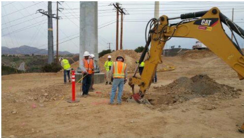
Caption Excavation for risers at PO3. Archaeology monitor present.
