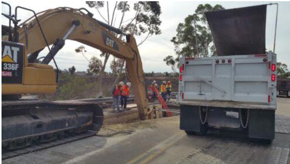
Caption Excavation, Pomerado Road. Monitors present.
