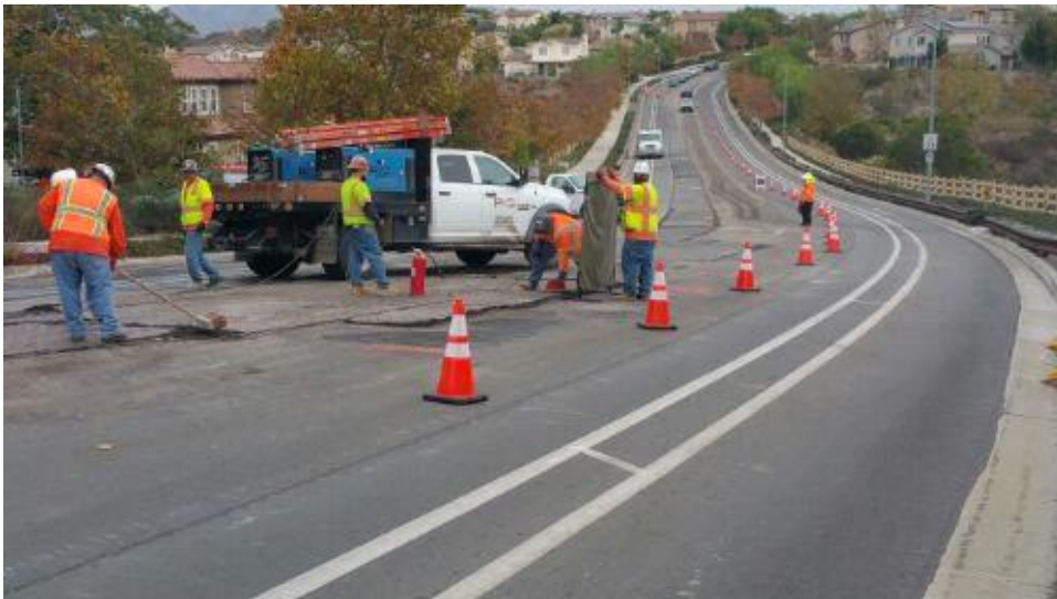
Caption Welding trench plates on Stonebridge Parkway.
