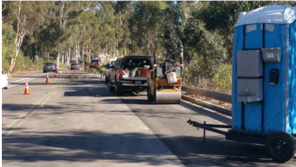
Caption Repaving crew on Pomerado Road.
