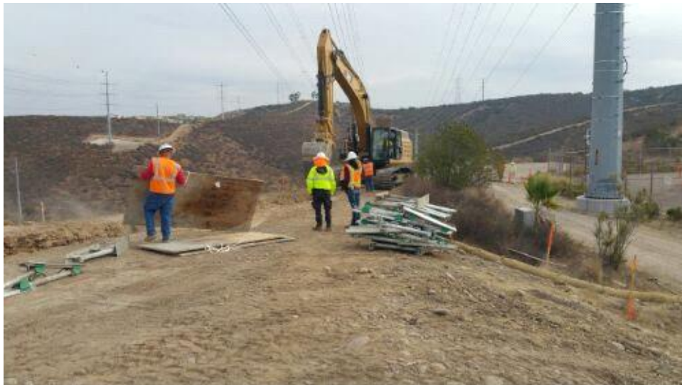
Caption Trenching at PO3 with monitors present.
