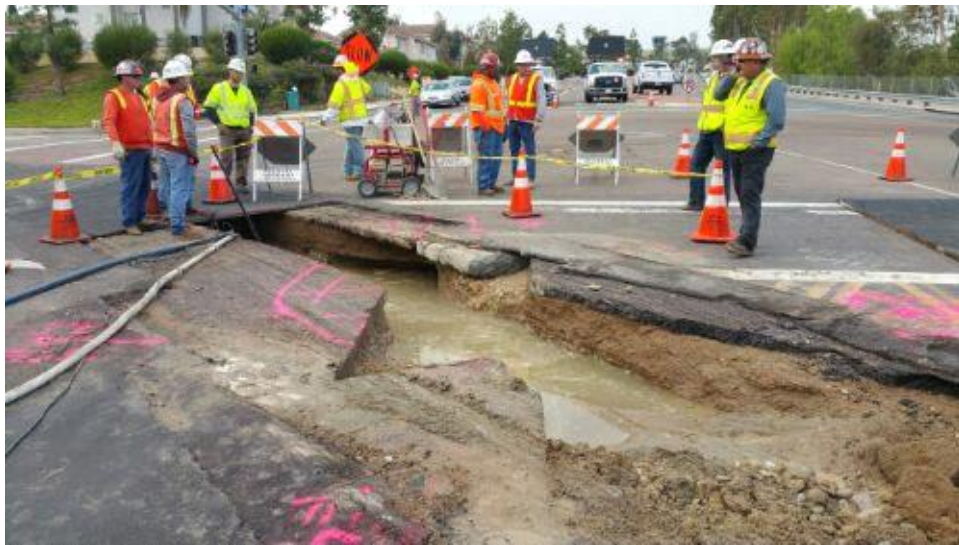
Caption Water line repair in progress on Pomerado Road.
