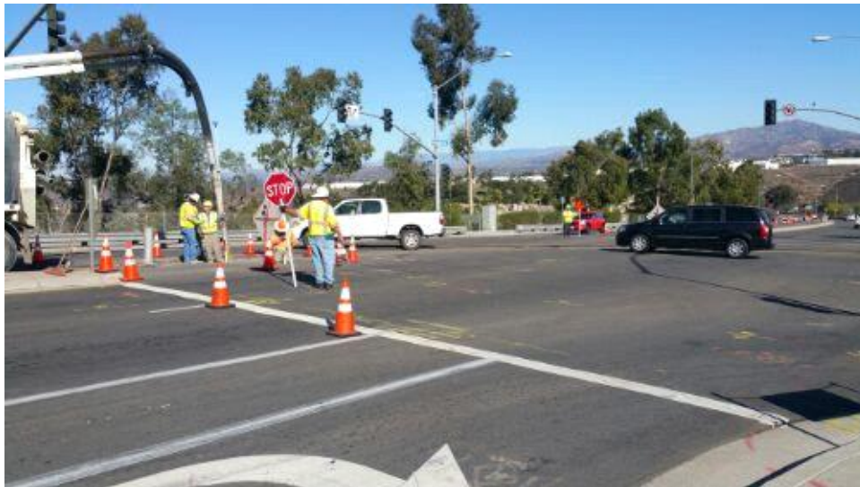
Caption Potholing at Pomerado Road and Stonebridge Parkway.
