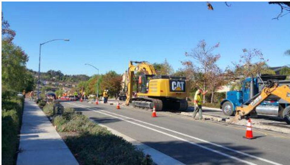
Caption Digging on Stonebridge Parkway. Two monitors on hand.
