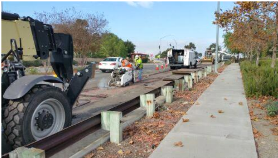
Caption Grinding pavement on Stonebridge Parkway.
