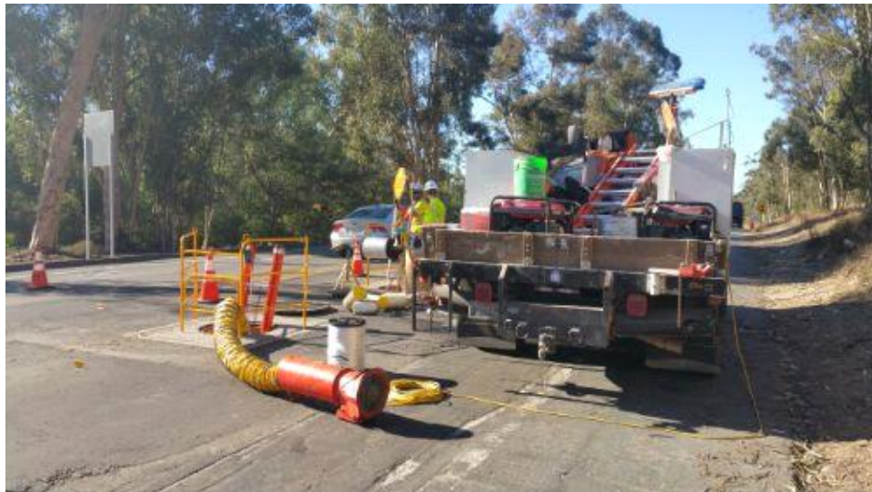
Caption Mandreling crew with traffic control and fire equipment.
