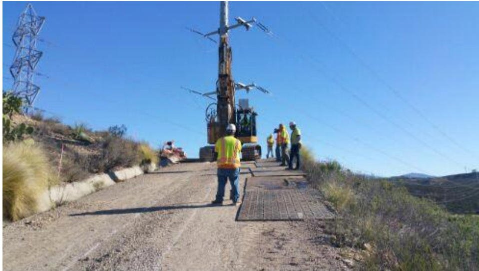
Caption Digging trench in PO5 access road.
