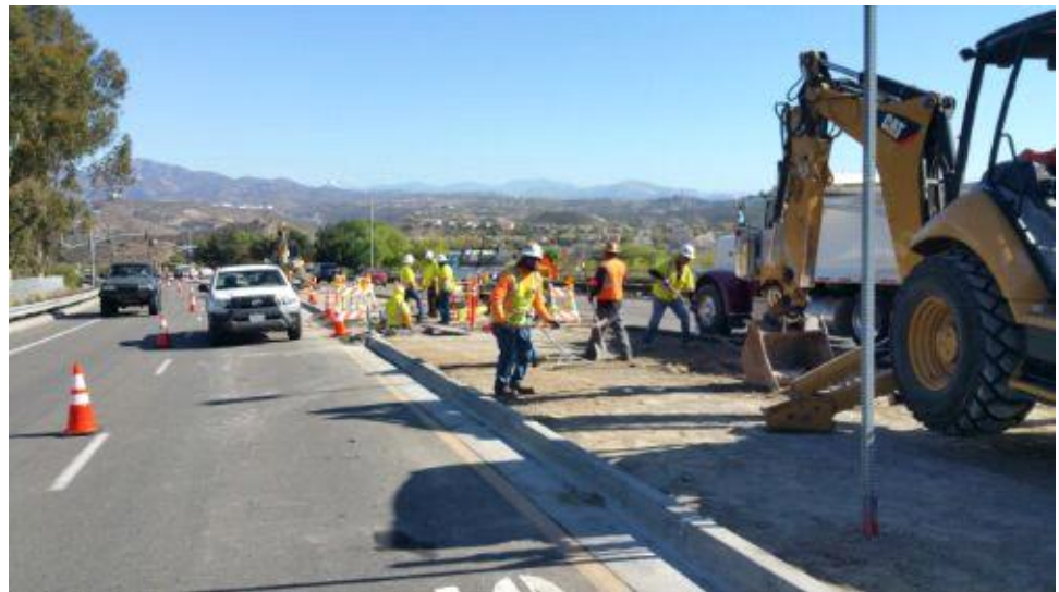
Caption Removing concrete from Pomerado Road median and mandreling.
