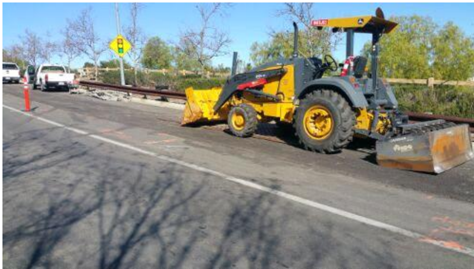
Caption Staging area on Stonebridge Parkway. Drip pan is under equipment.
