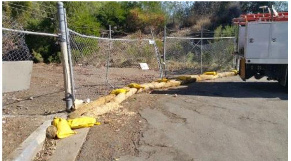
Caption Erosion controls BMPs at bottom of Kearney Mesa Road work area.
