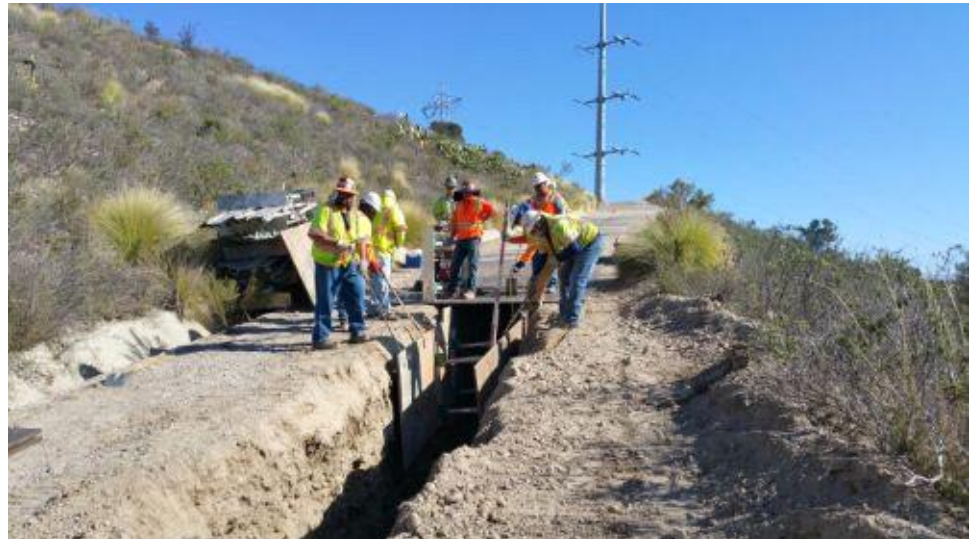
Caption Trenching in PO5 access road, 2 monitors present.
