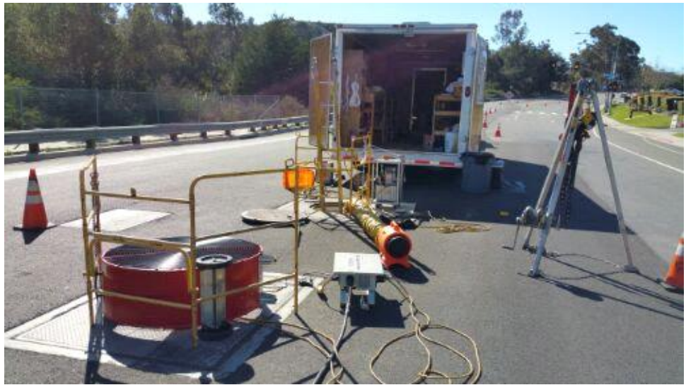
Caption Vault work site, Carroll Canyon Road.
