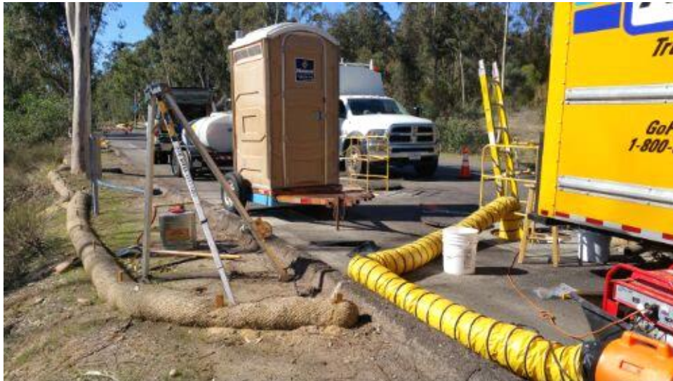
Caption Vault work site on Pomerado Road.
