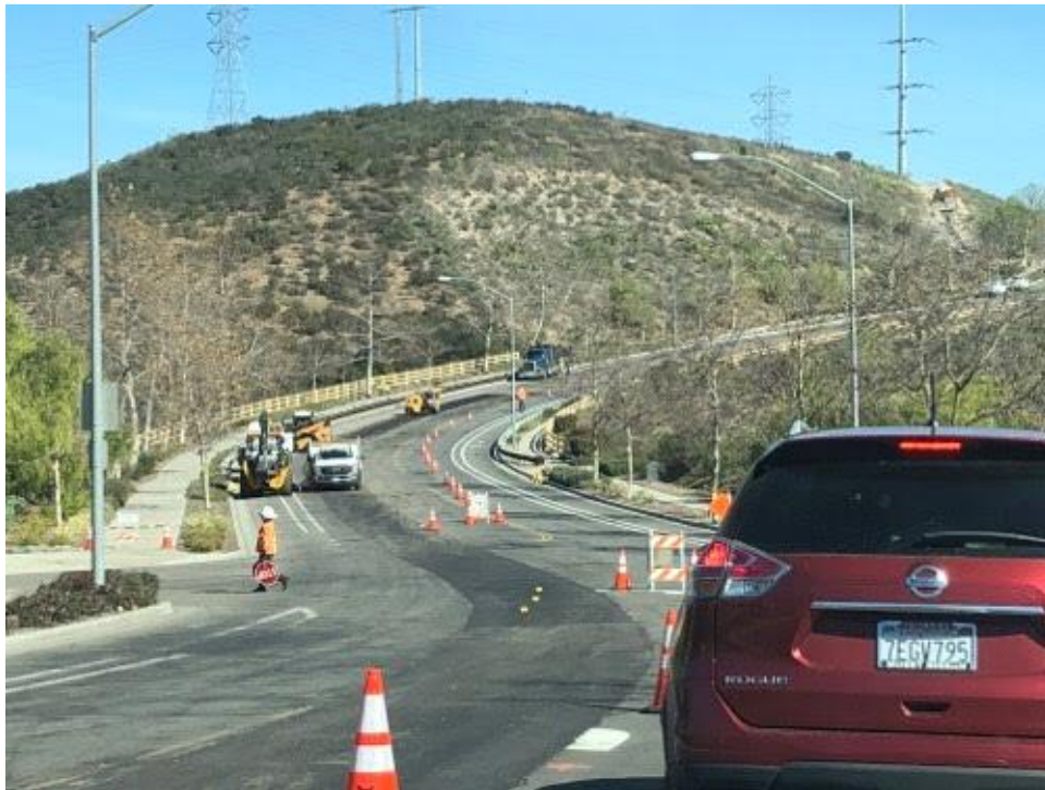
Caption Paving and traffic control on Stonebridge Parkway.
