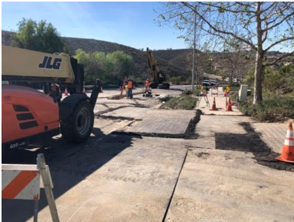
Caption Trench work on Stonebridge Parkway.
