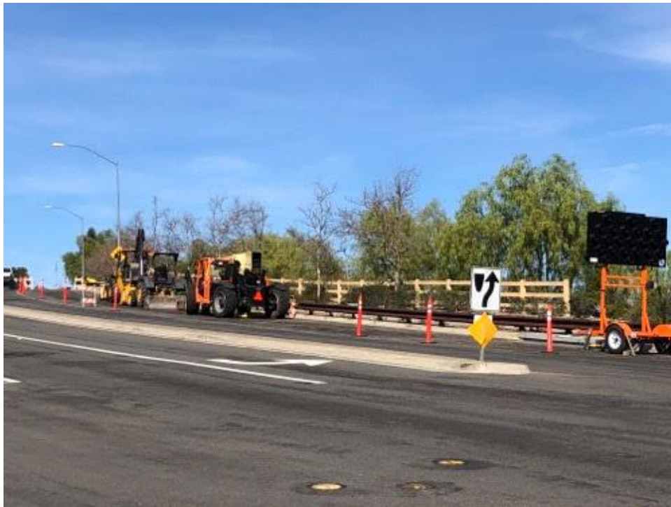
Caption Equipment storage Stonebridge Parkway.
