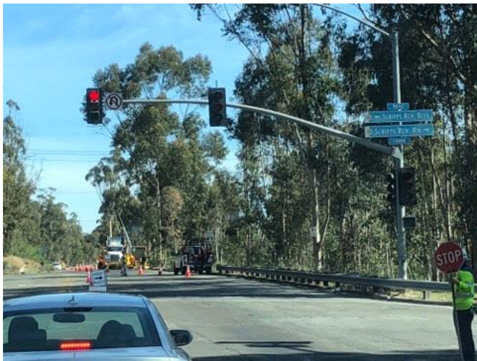
Caption Cable installation on Pomerado Road.
