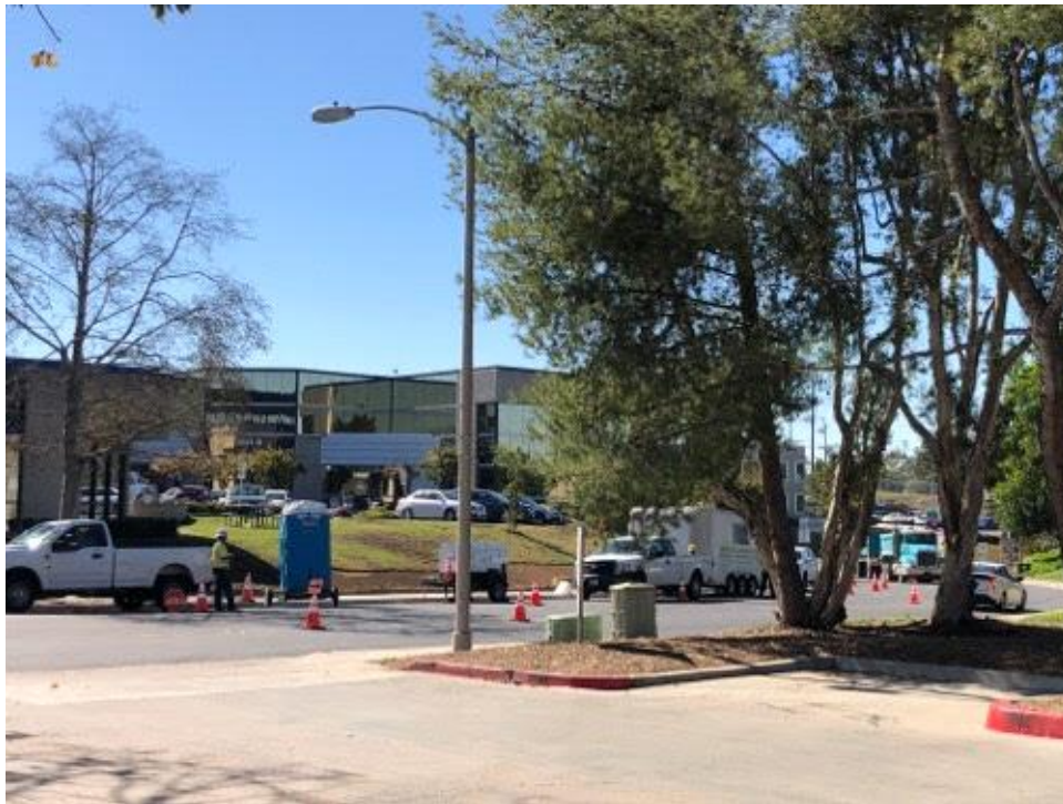
Caption Vault/cable work on Activity Road.
