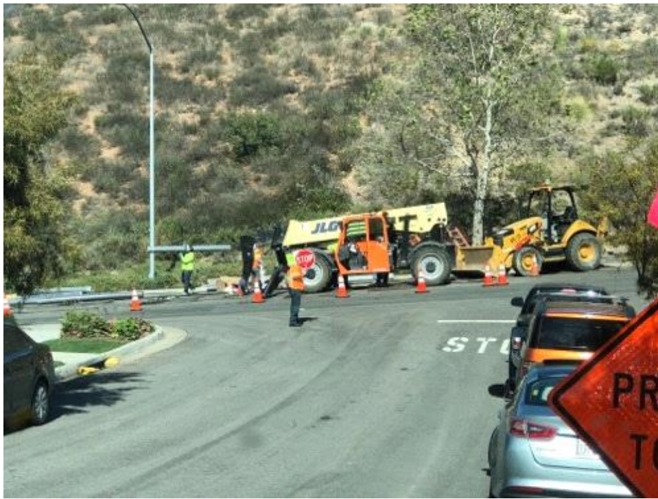
Caption Trench work and traffic control on Stonebridge Parkway.
