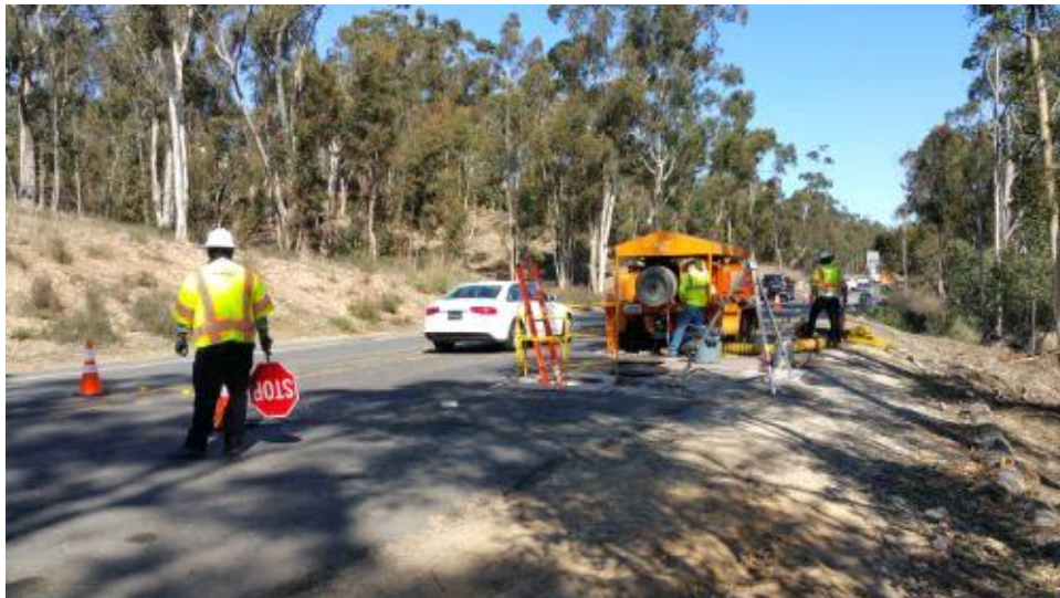
Caption Mandreling and cable pulling on Pomerado Road.
