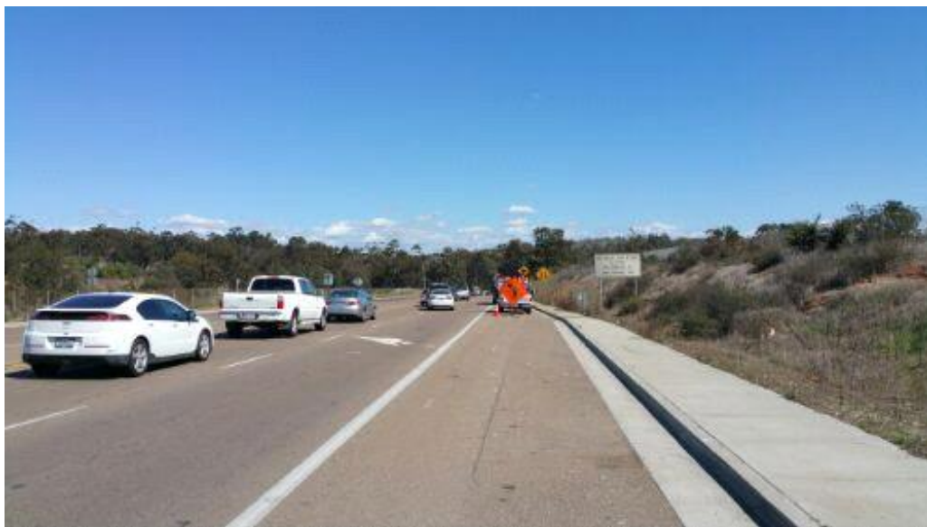
Caption Traffic control at east end of Pomerado Road work area.
