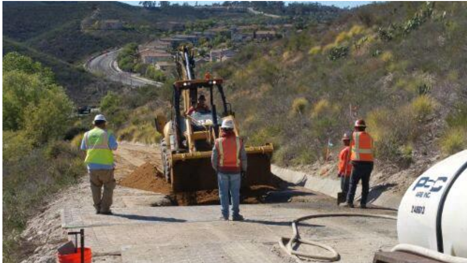
Caption Filling trench at PO5 access road.
