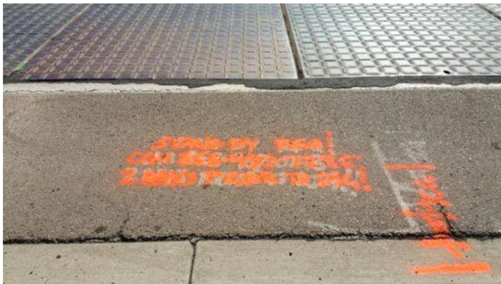
Caption Water line intersecting trenching route on Pomerado Road.
