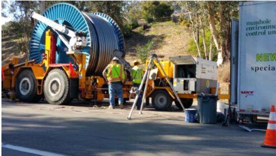
Caption Stringing cable on Pomerado Road.
