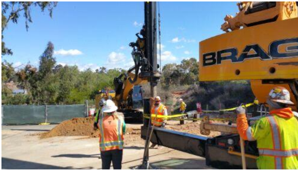
Caption Drilling for placement of supports for pit at Kearney Mesa Road. Paleontology monitor present.
