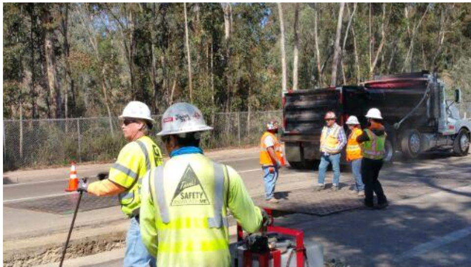
Caption Resource monitors at trenching site on Pomerado Road.
