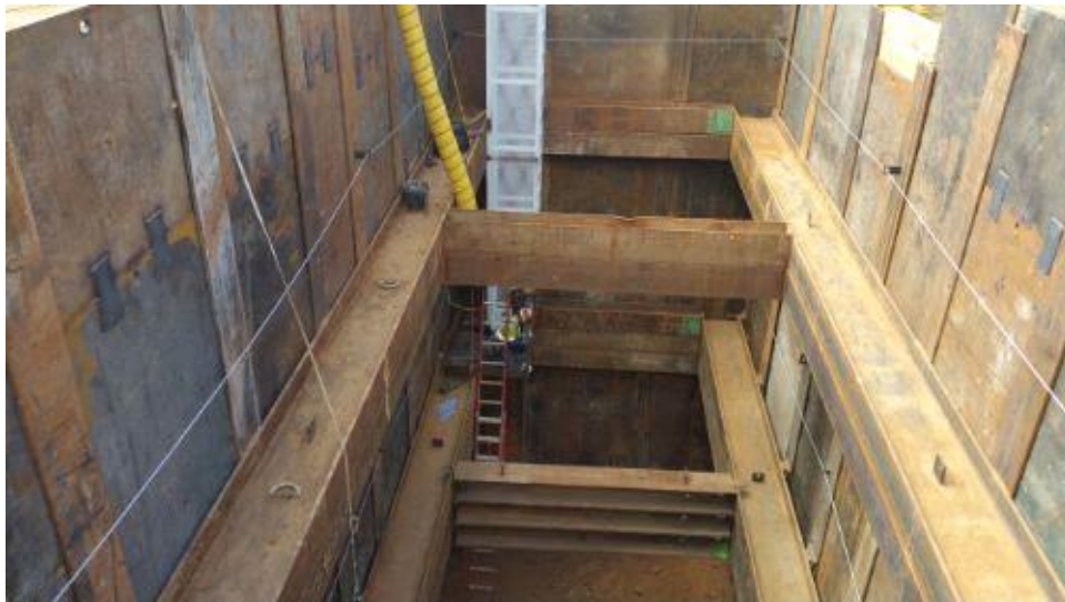
Caption Installing ladder in sending bore pit, Kearney Mesa Road.
