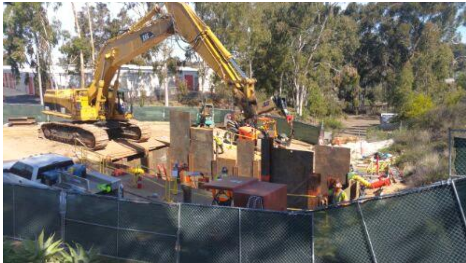
Caption Kearney Mesa Road sending pit site overview.
