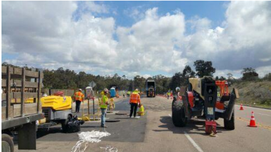
Caption Repaving and mandreling on Pomerado Road.
