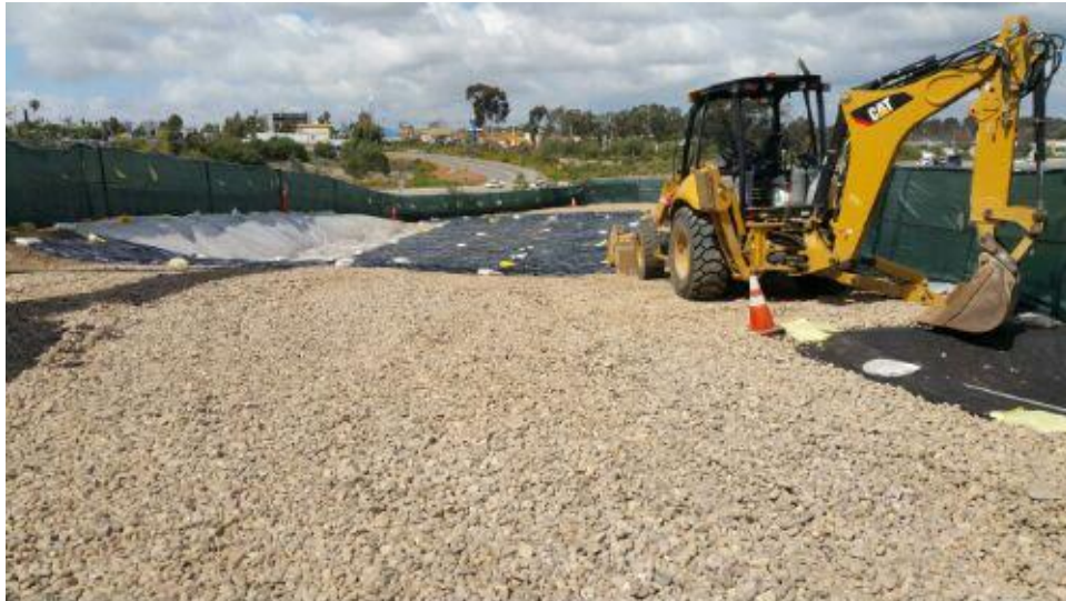
Caption Receiving pit site, near I-15 ramp.
