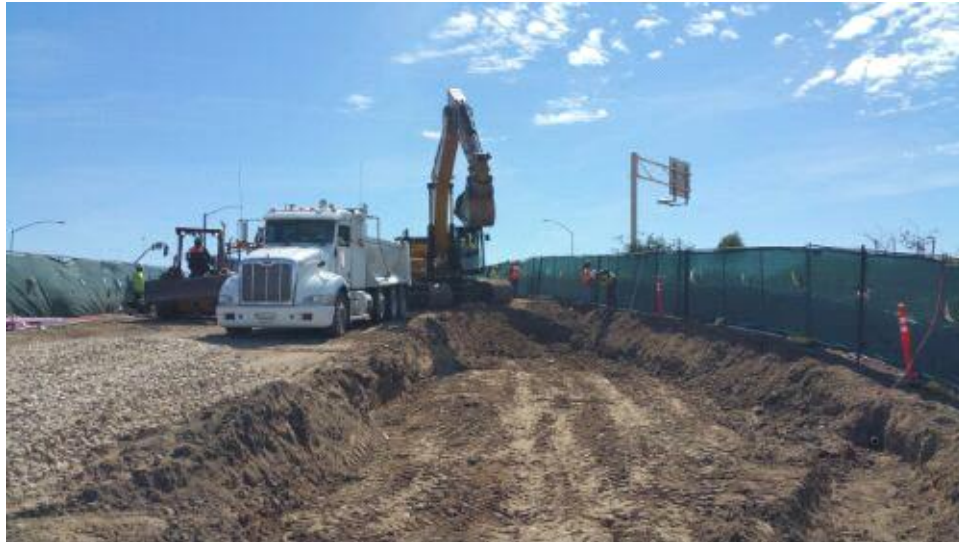
Caption Grading for receiving pit. Native American and archeology monitors on site.
