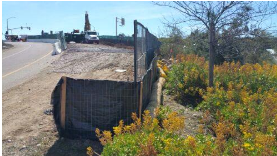
Caption Erosion control BMPs, receiving pit site.
