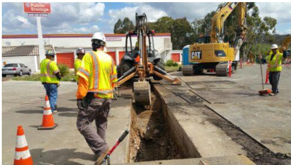
Caption Trenching on Kearney Mesa Road.
