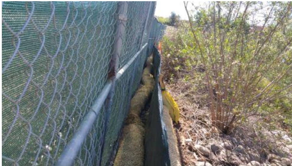
Caption Erosion control BMPs, receiving pit site.
