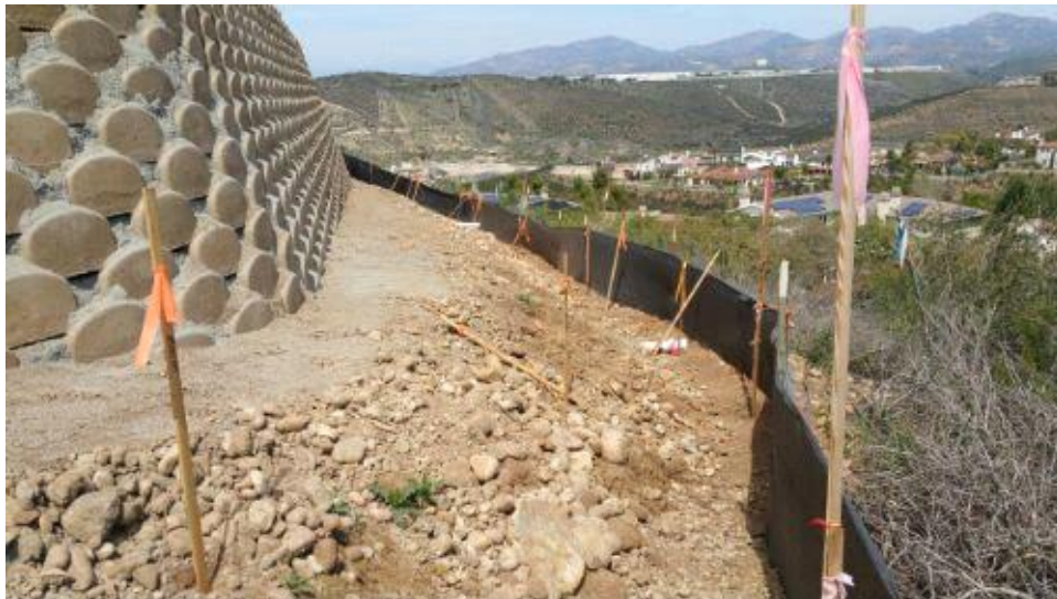
Caption Drains installed below Verdura wall at PO5.
