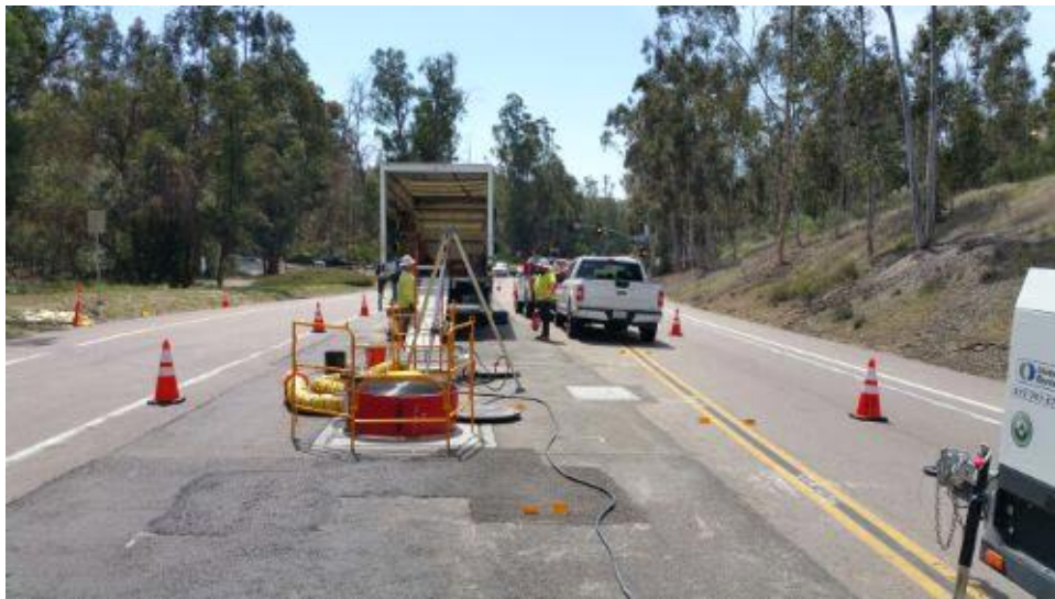
Caption Splicing work site on Pomerado Road.
