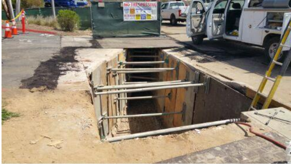
Caption Trench to Kearney Mesa Road sending bore pit.
