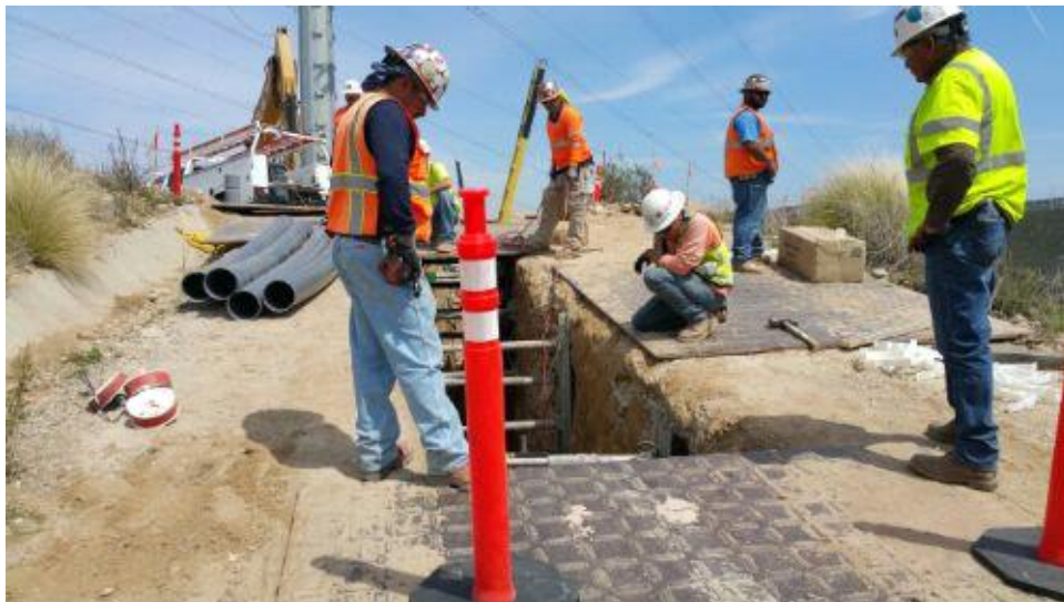
Caption Placing conduit in PO5 access road.
