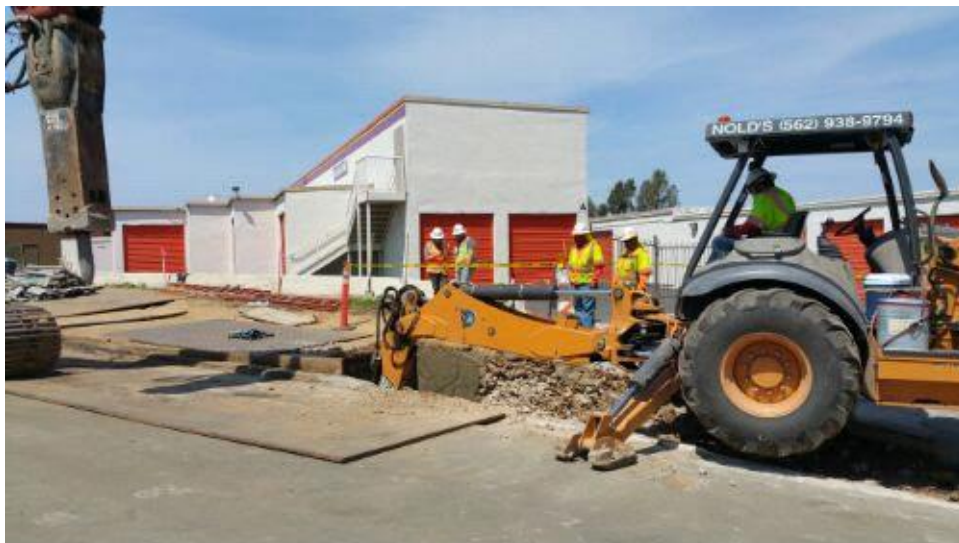
Caption Cultural and paleontology monitors at trench excavation, Kearney Mesa Road.
