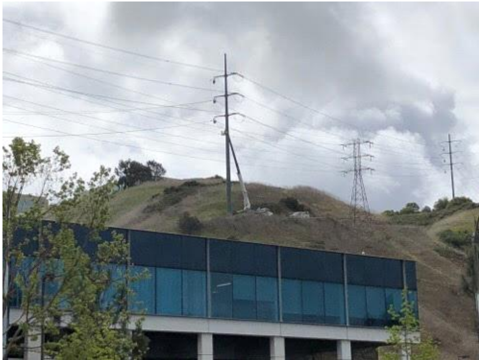
Caption Overhead pull crew at pole south of Sorrento Valley Boulevard.
