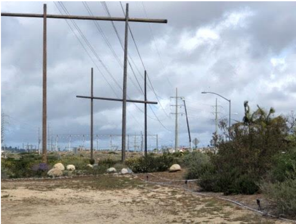
Caption Overhead crew at Penasquitos Substation.
