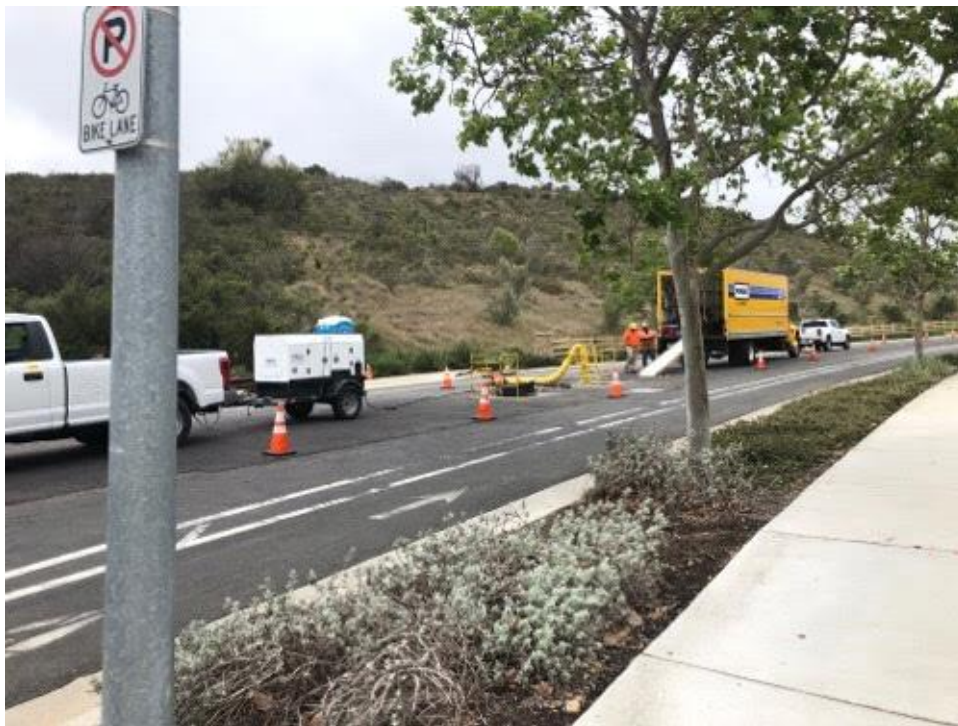
Caption Vault work on Stonebridge Parkway - splicing crew.
