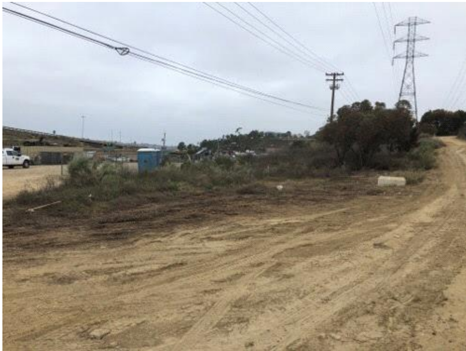
Caption Wood poles removed from CC MM CP site.
