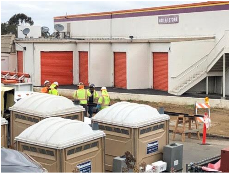
Caption Workers prepping steel beams for bore pit.
