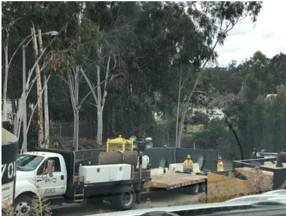
Caption Supply delivery, crane will lift into bore pit.
