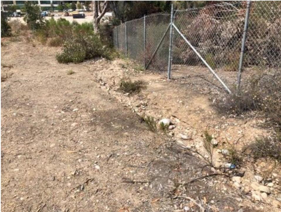
Channel off outlet road.
