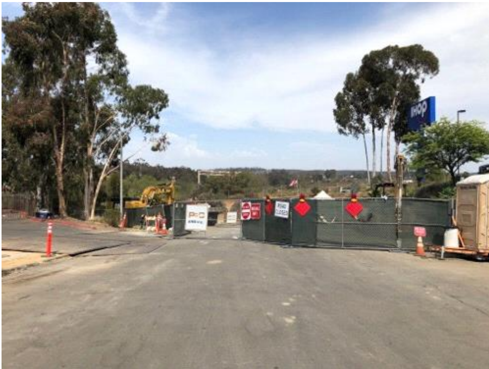
Caption Western vault no work at time of photo.
