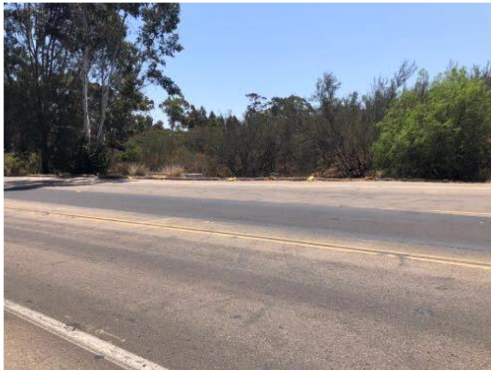
Caption BMPs and repaving east of I-15 on Pomerado. Photo Attributes Capture Date/Time: Sat Jul 14 2018 12:12:04 GMT-0700 (PDT) Coordinates: 32.894613, -117.109039 View Direction: Southeast
