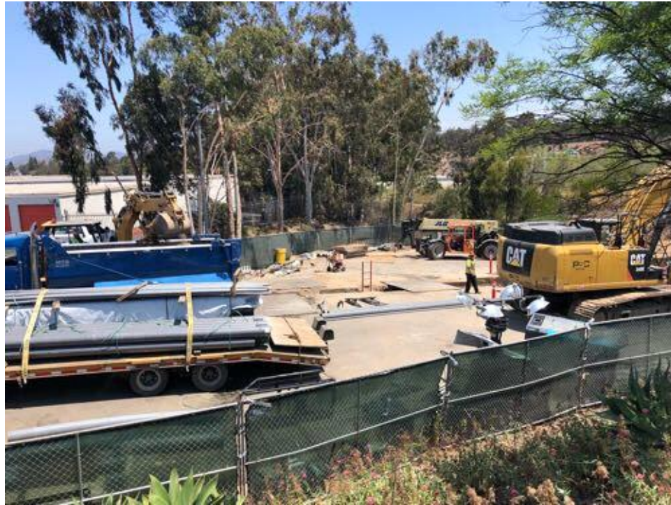
Caption West vault.
