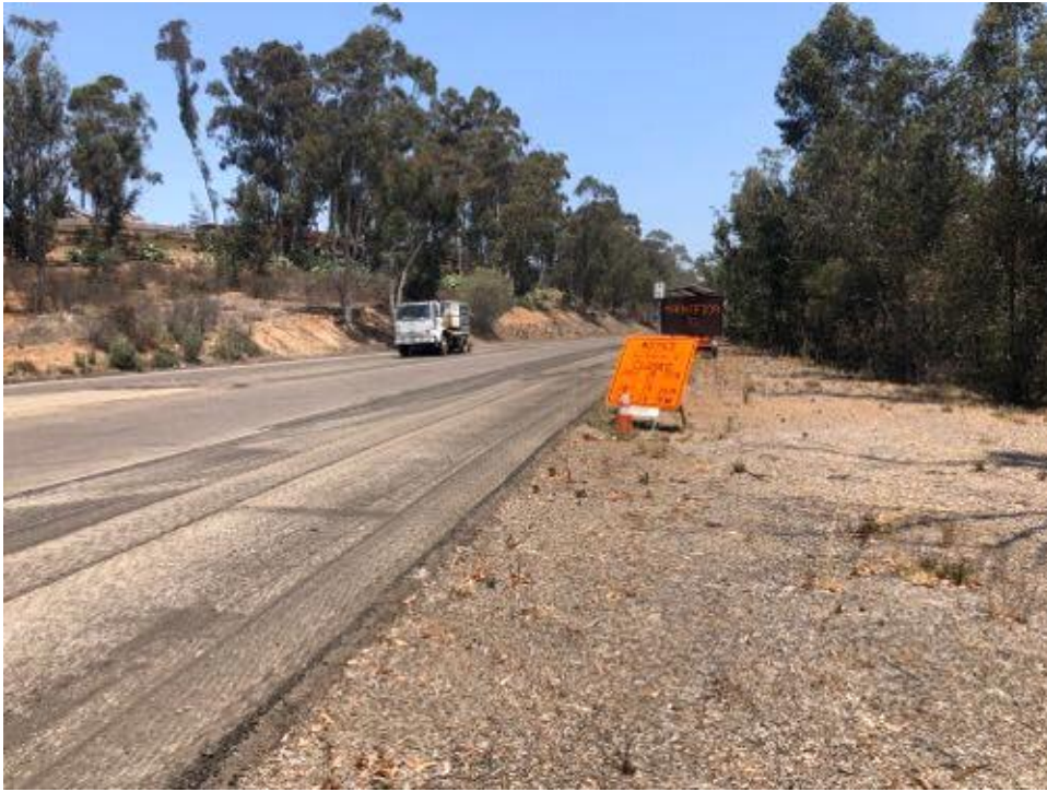
Caption Road cap and grinding plus water truck.
