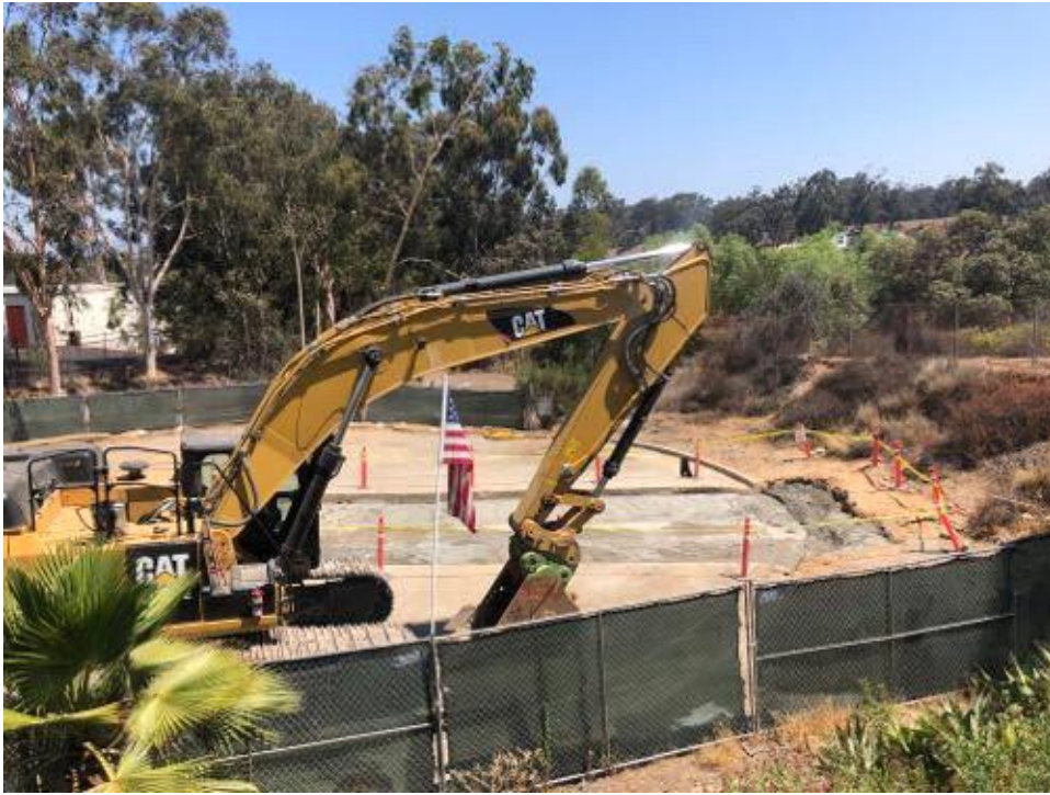
Caption Bore pit filled with concrete.
