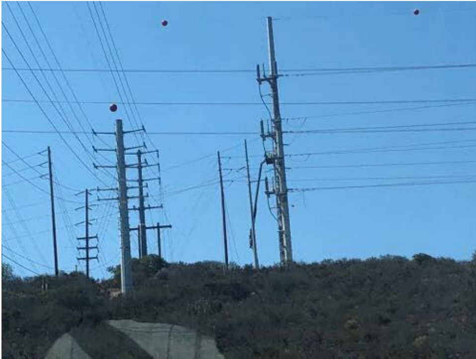
Caption Overhead work at P03.
