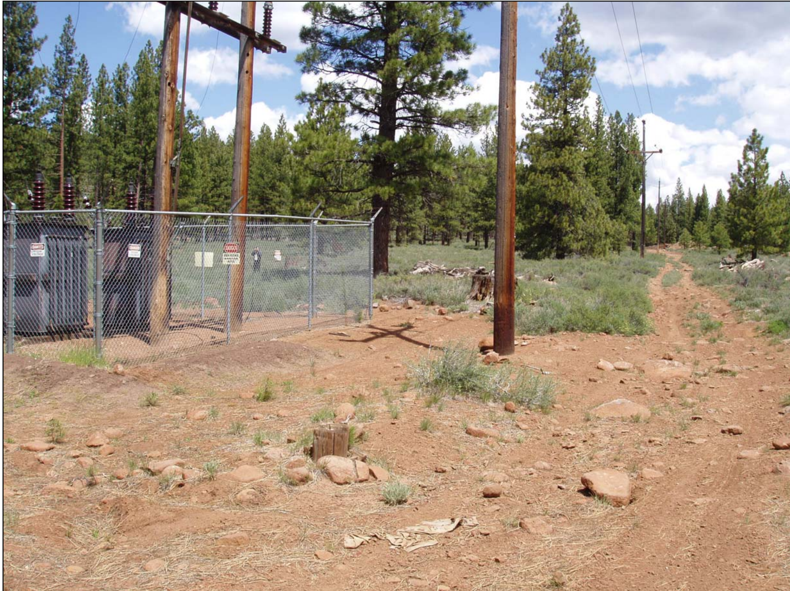
Photo 3: Existing Hobart Substation and access road (looking north)
