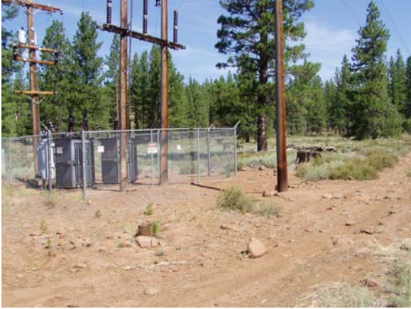
View of the existing substation and expansion area
