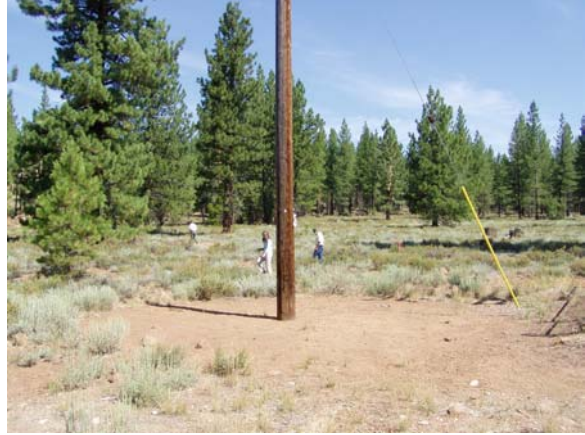
View of the substation expansion area
