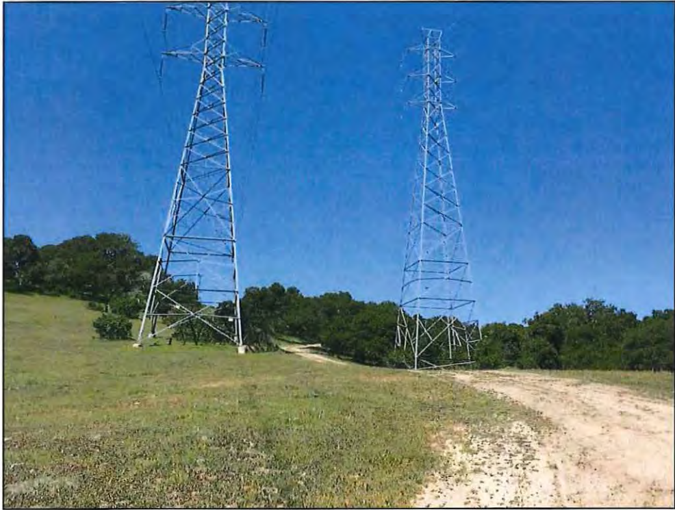
Photo 1. Overview of Tower 10/50 (left), view west-northwest.
