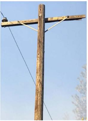
**Figure 2:** Pole and Damaged Crossarm (Source: PG&E)
