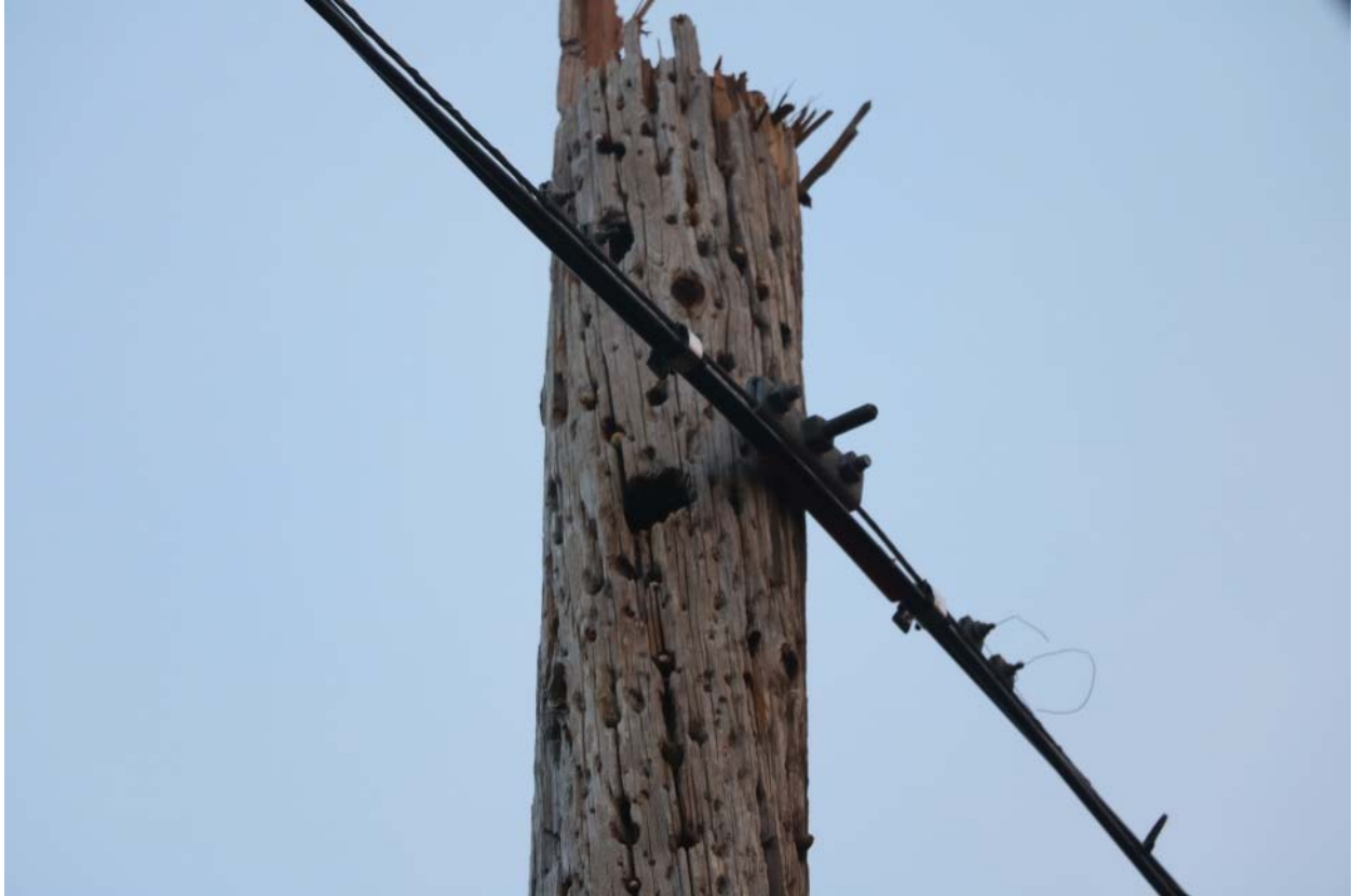
Figure 7. Break 18 inches above the communication conductor attachment on Fuse Cutout Pole 1447 with woodpecker holes (Source: CAL FIRE)
