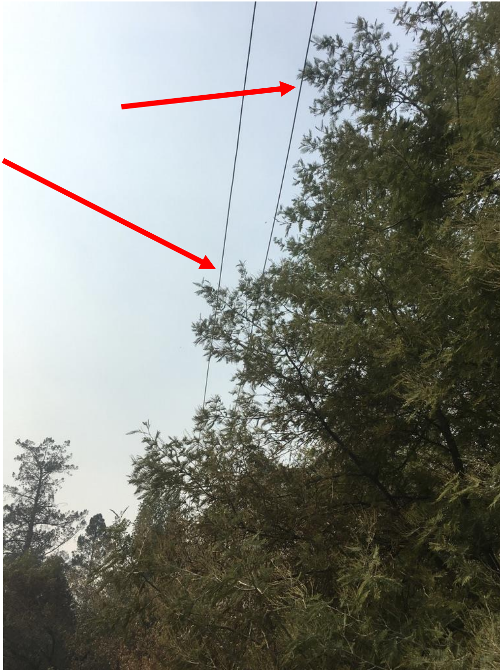
Photo 12 - existing conditions of clearance. Trees along span in contact with wire and overhanging.
