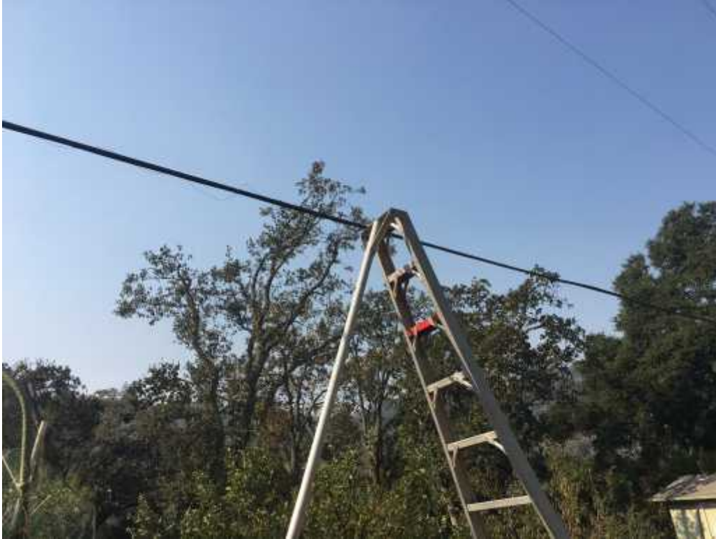
Figure 2: Photo of CIP cable mid-span with lashing wire
