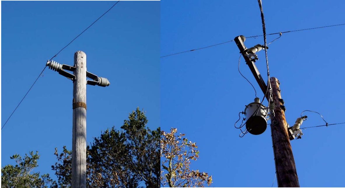
Figure 6. Atlas 1 Left: Subject pole #1, 40-foot pole (PG&E pole #102292423, coordinates: 38.409797, -122.246232). Photo taken from the southeast side of pole, looking north. Right: Subject pole #2, 45-foot pole with transformer attached (PG&E pole #102292420, coordinates: 38.409435, -122.245904). Photo taken from southwest side of pole, looking northeast.
