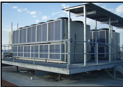
Example 150-Ton Air Cooled Chiller
